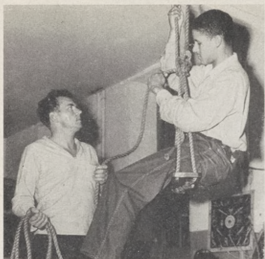
Able-bodied Seamen's upgrade course includes rigging a bo'sun's chair.
