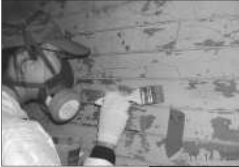
Workman cleaning a barrack wall. Using SAT funds, paint and putty were removed to reveal poems by Chinese immigrants.
