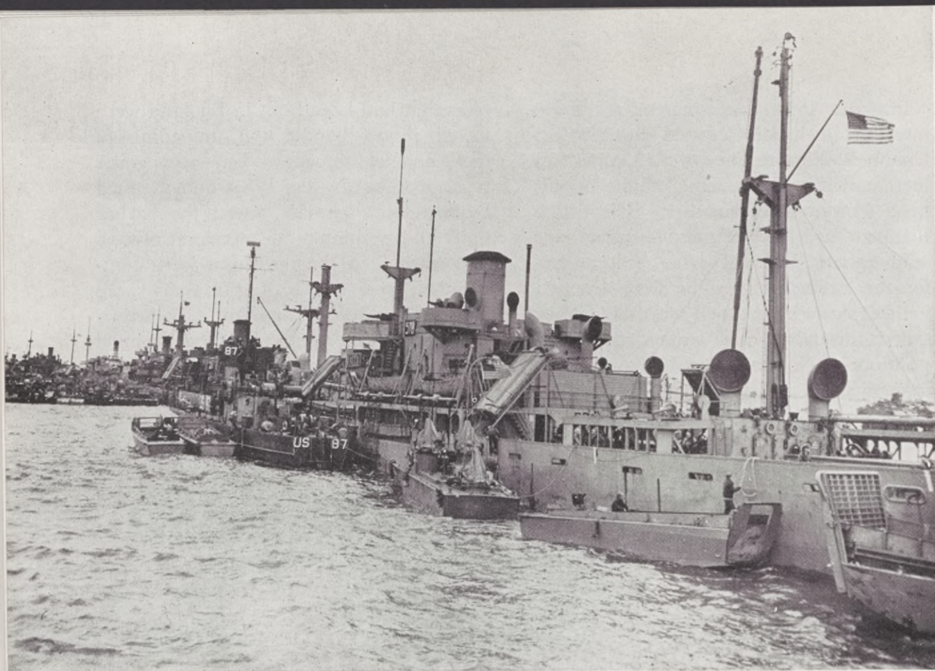
Liberty ships and tankers too old or too badly damaged to keep sailing serve to protect the artificial harbor off Normandy.
