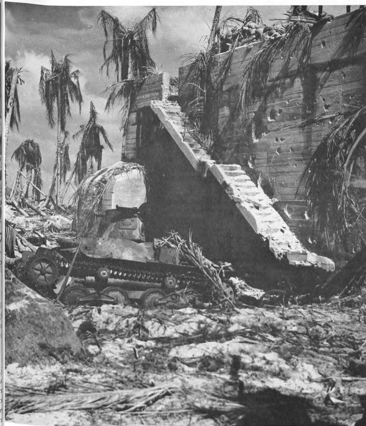
JAPANESE COMMAND POST with enemy tank in foreground. Shells and bombs had little effect on this reinforced concrete structure.
