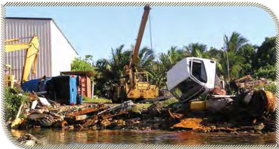
*Using trash and scrap material to build shoreline protection has many negative impacts on the coast and surrounding ecosystem and should be avoided.*
