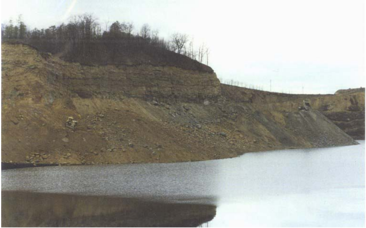
Photo 11. Construction of Seepage Barrier (Long View of Dozer and Truck) - March 6, 1995. Source: GAI. The work is being conducted at the southwest side of the impoundment. Pool elevation 1,000 feet msl. Mine roof elevation 964 feet msl.
