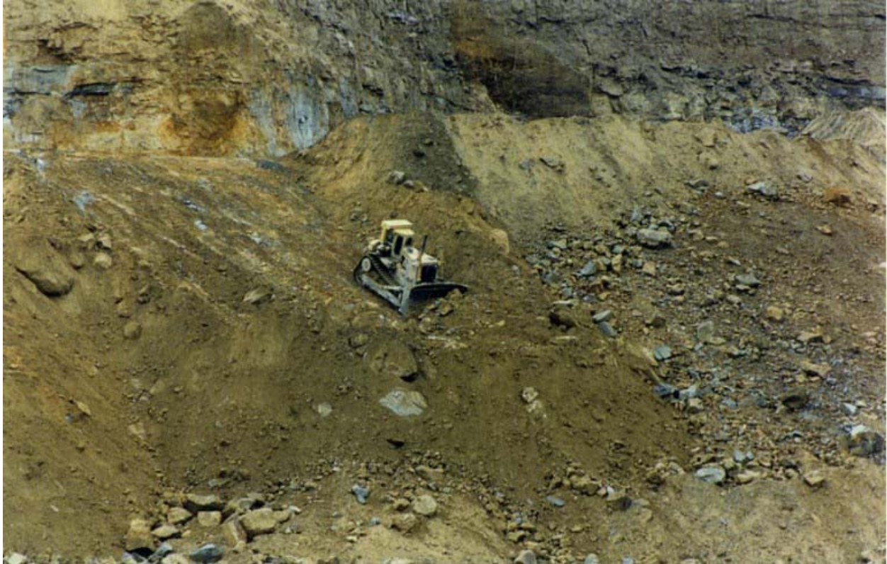
Photo 9. Construction of Seepage Barrier (Dozer Work) - March 6, 1995. Source: GAI. The work is being conducted at the southwest side of the impoundment.
