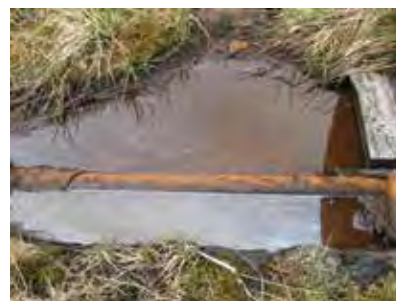
Fuel tank farm 2 with leaking fuel. D. Rudis, USFWS.
