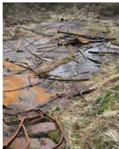
Collapsed tanks at fuel tank farm 2 and residual POL. D. Rudis, USFWS.
