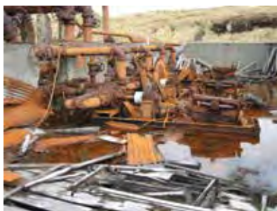
Fuel Tank Farm 2 – lower pump station is typical of all fuel pump stations on Attu. D. Rudis
