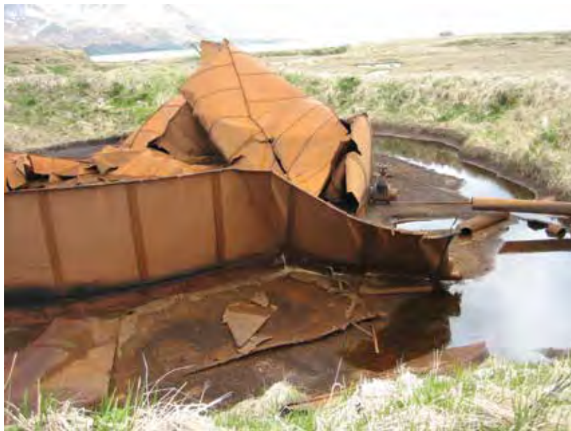
Fuel tank at fuel tank farm 2. These tanks were burned in an unsuccessful attempt to remove remaining fuel. D. Rudis, USFWS
