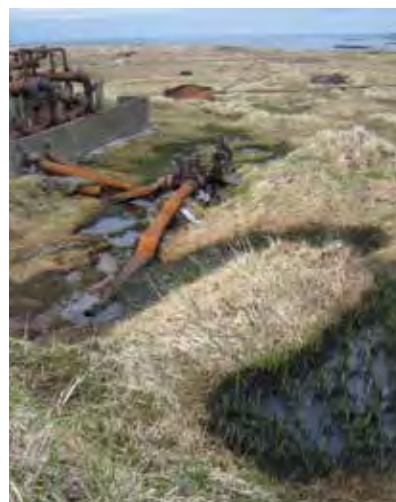
Fuel tank farm 2, lower pump station POL contamination into the downstream swale. D. Rudis, USFWS.
