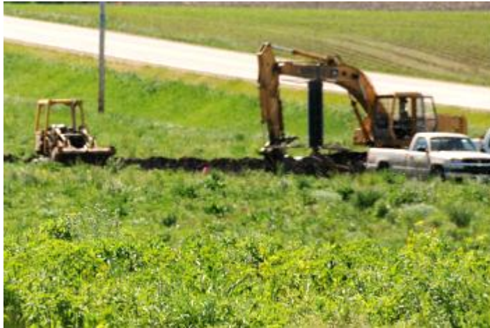
Drainage Tile Installation
