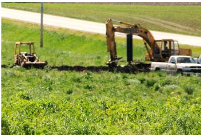
Drainage Tile Installation
