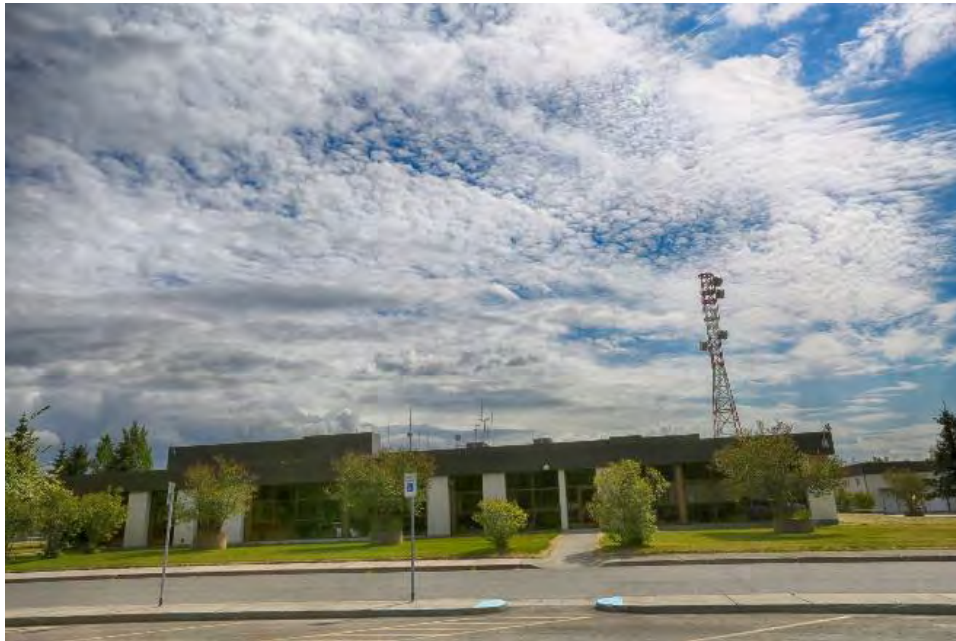
Figure 127. Air Traffic Control Center, 700 North Boniface Parkway, Anchorage was designed by Lucien Cassetta, 1967 (source: Anchorage Air Route Traffic Control Center 2016).
