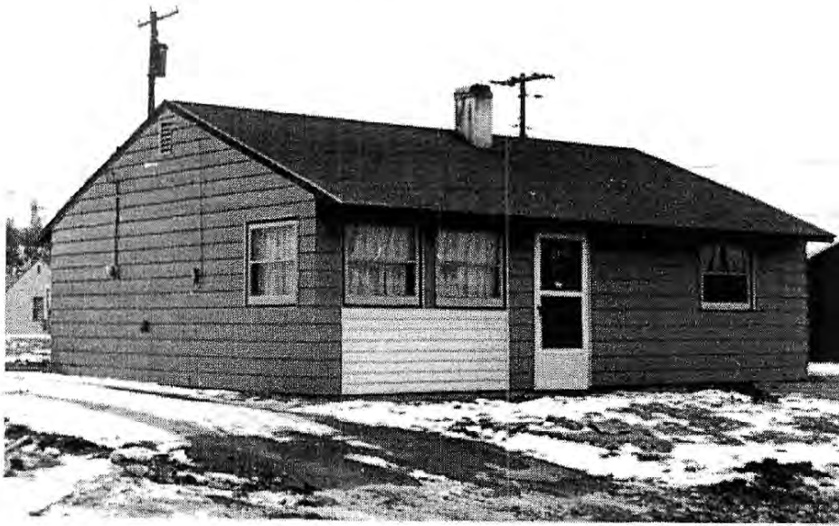
Figure 7. Housing constructed in 1954 on Elmendorf Air Force Base, extant (source: Stokes 2006).
