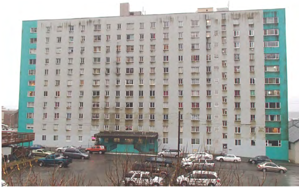
Figure 60. The Marine View Tower (formerly Wingren Court) as seen today (source: Yarborough and Welsh, 2014).
