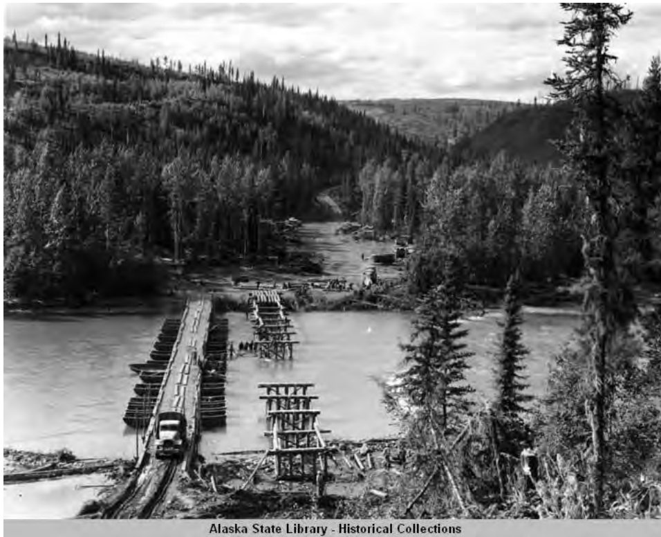
Figure 23. Bridge construction along the Alaska Highway, 1943 (source: Alaska State Library, Historical Collections, Alaska Highway Construction Photograph Collection, ca. 1942-1943, ASL-PCA-193-047).
