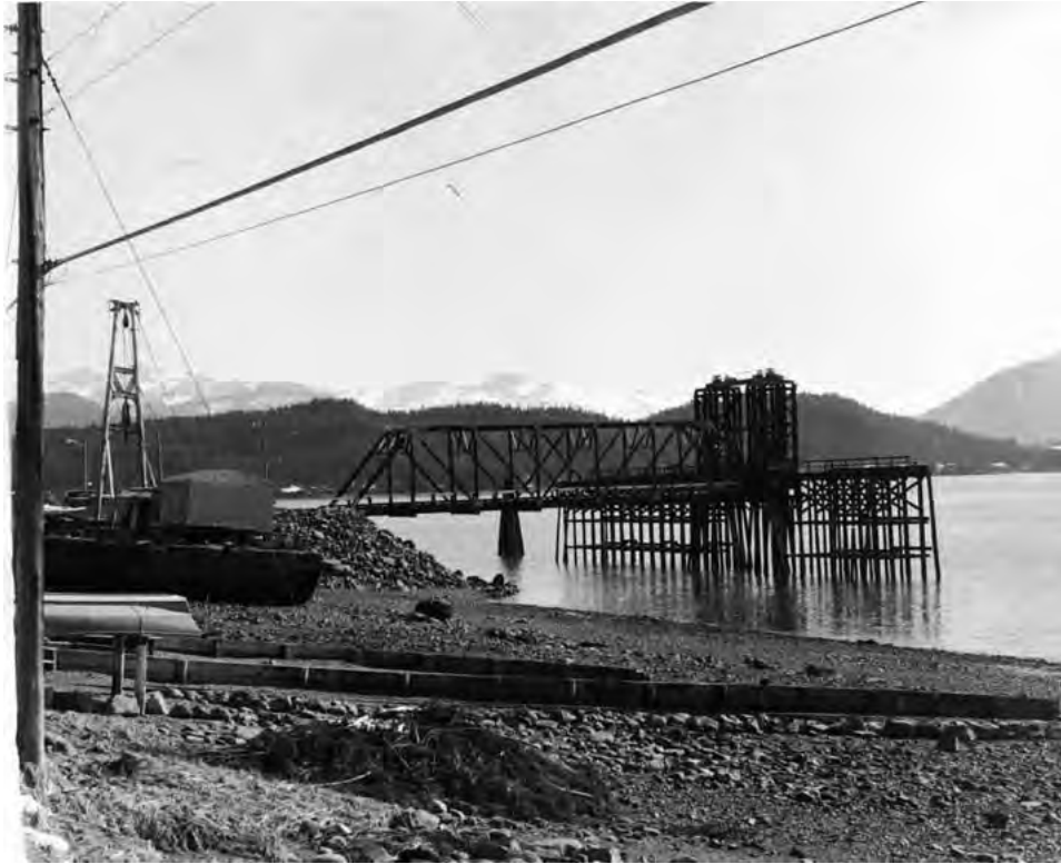
Figure 26. Auk Bay Ferry Terminal, Tee Harbor, 1963; demolished (source: Alaska State Library, Historical Collections, Alaska State Library Place File, ASL-Juneau-Vicinity-AukeBay-TeeHarbor-11).
