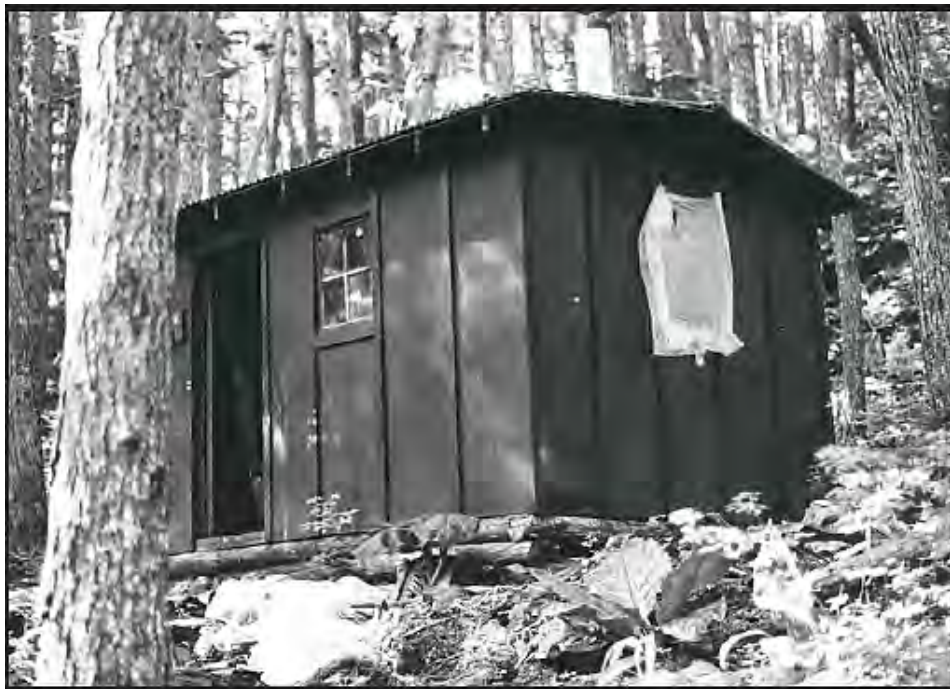
Figure 46. A public use cabin at Shelter Island, built by USFS in 1955, using plywood (source: Lantz 2010).
