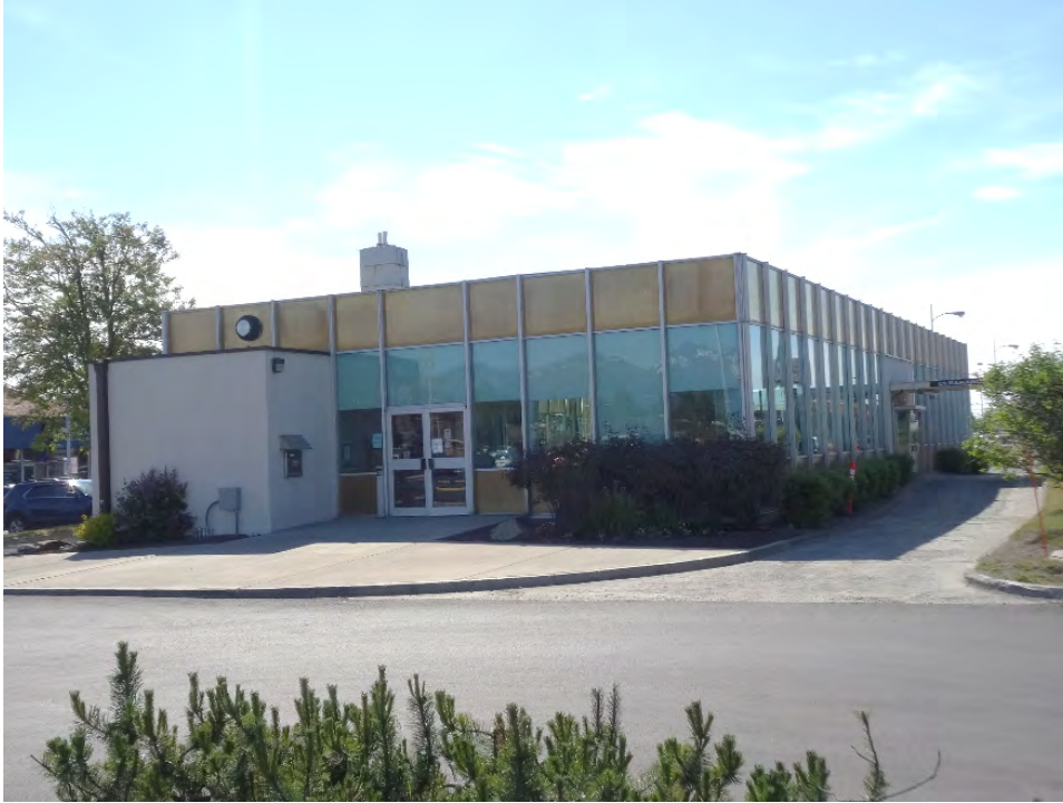
Figure 37. First National Bank, Northern Lights Branch, Anchorage, present-day (source: TNSDS 2016).
