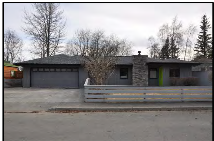
Residential Building, South Addition, Anchorage
