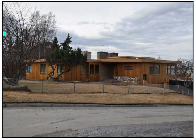
Residential Building, South Addition, Anchorage
