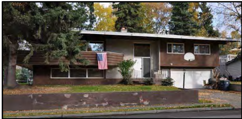
Bi-level Contemporary- Residential Building, College Village, Anchorage
