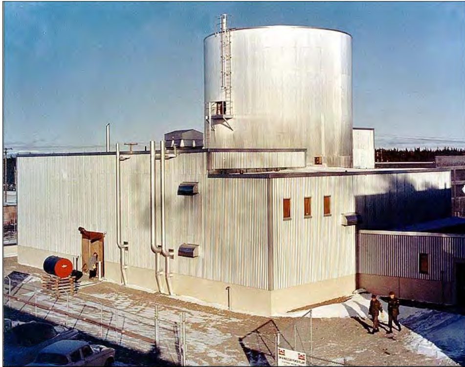
Figure 15. The SM-1 Reactor Facility at Fort Greely, ca. 1965 (source US Army 1965).
