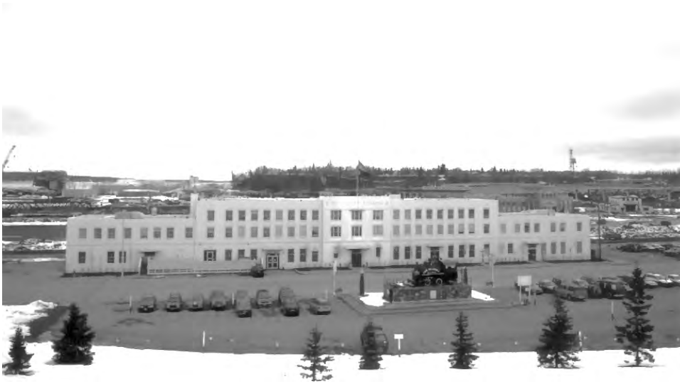
Figure 96. The Alaska Railroad Anchorage Depot, as seen in 1999 (source: National Register Nomination, Blasingame 1999).
