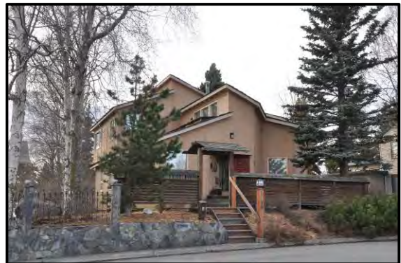
Residential Building, South Addition, Anchorage
