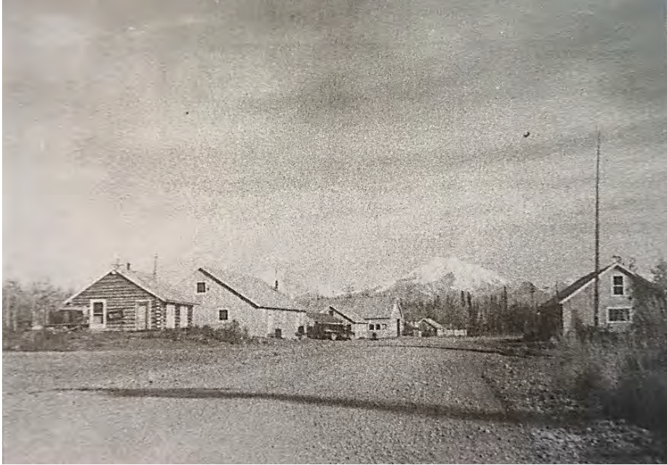
Figure 83. The Alaska Road Commission depot at Glennallen, ca. 1950, some buildings still extant (source: Alaska and Polar Regions Collections, Elmer E. Rasmuson Library, University of Alaska Fairbanks, Fred Machetanz Collection in the National Archives).
