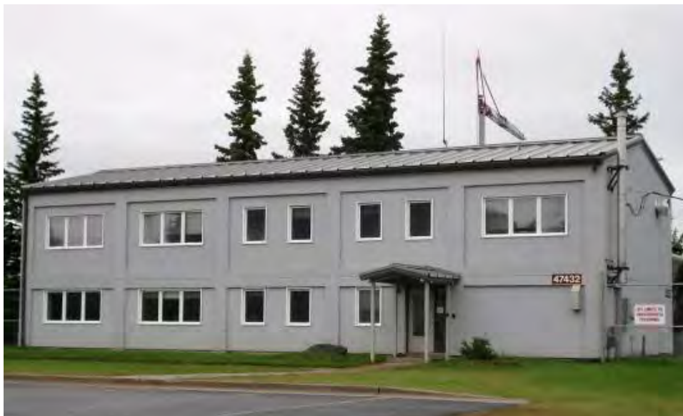
Figure 89. Civil Support Team building, (Bryant Army Air Field, built 1960) Elmendorf Air Force Base, present day (source: Sneddon and Miller 2012).
