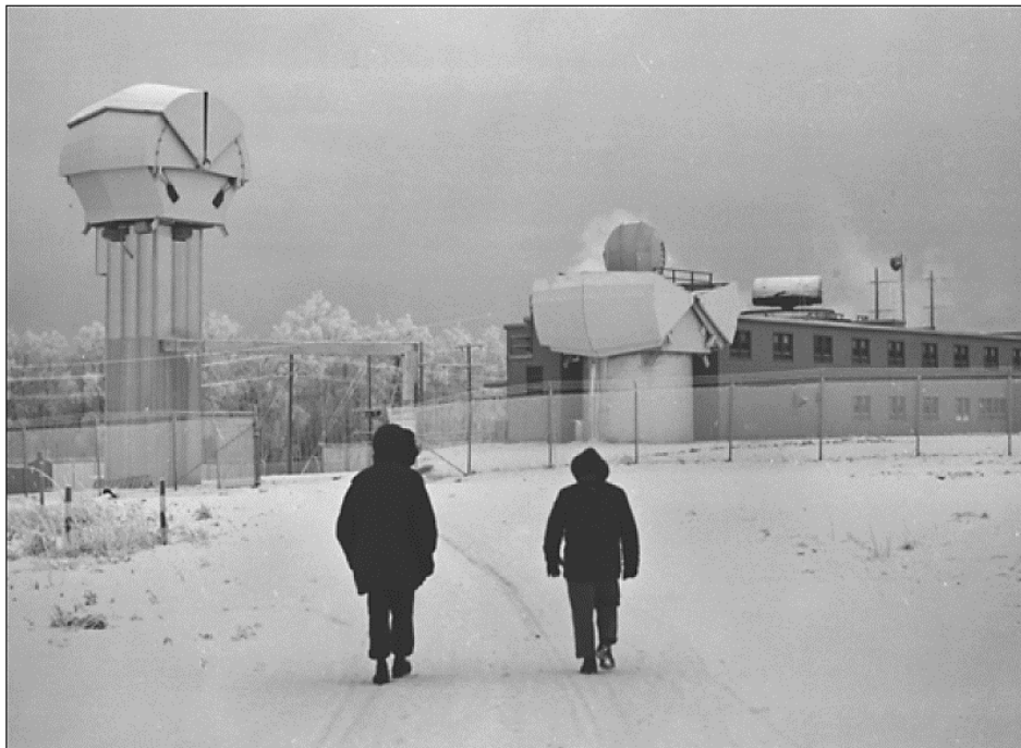
Figure 9. Nike Site Summit, Arctic Valley, 1962; note clam shell over radiodome (source US Army in Hollinger 2004).
