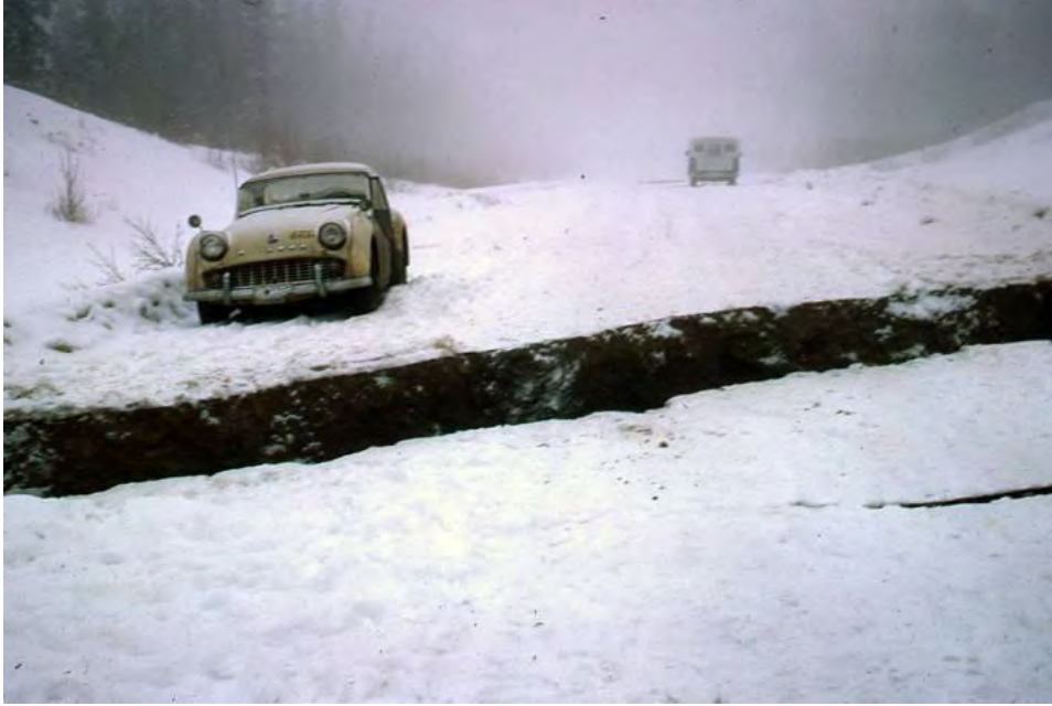
Figure 24. Large fissure on a roadway in Anchorage after the earthquake, 1964 (source: University of Alaska Anchorage, Consortium Library, Archives & Special Collections, Alice and Bob Arwezon photographs, 1949-1973, UAA-HMC-1140).
