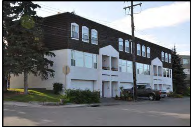
Multi-family Building, South Addition, Anchorage
