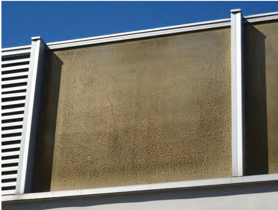
Figure 49. An enameled metal panel with "crackling" finish (source: TNSDS 2016).
