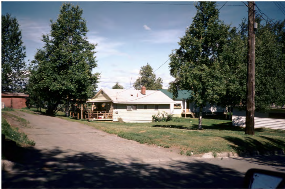
Figure 34. Example of a Harman House, a pre-fabricated metal residence, located on Government Hill, Anchorage (source: Hoagland 1993, 104).
