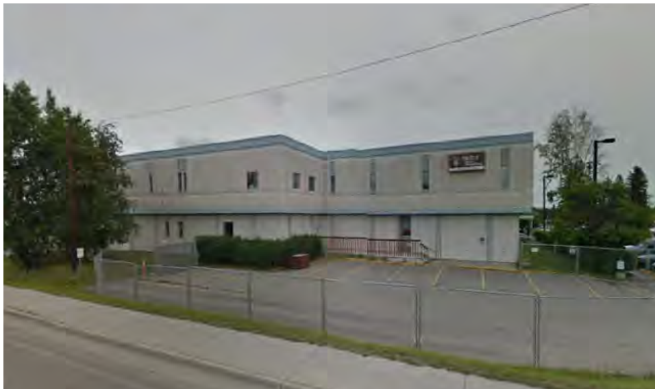
Figure 129. Fairbanks Medical Dental Arts Building, Lathrop Street, Fairbanks, and designed by Roger Cotting (source: Google Earth 2016).
