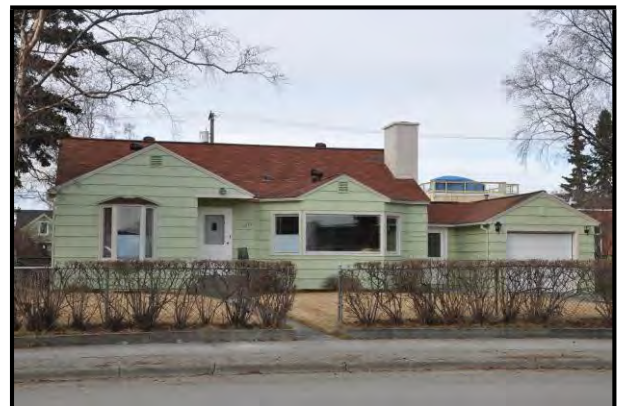
Residential Building, South Addition, Anchorage
