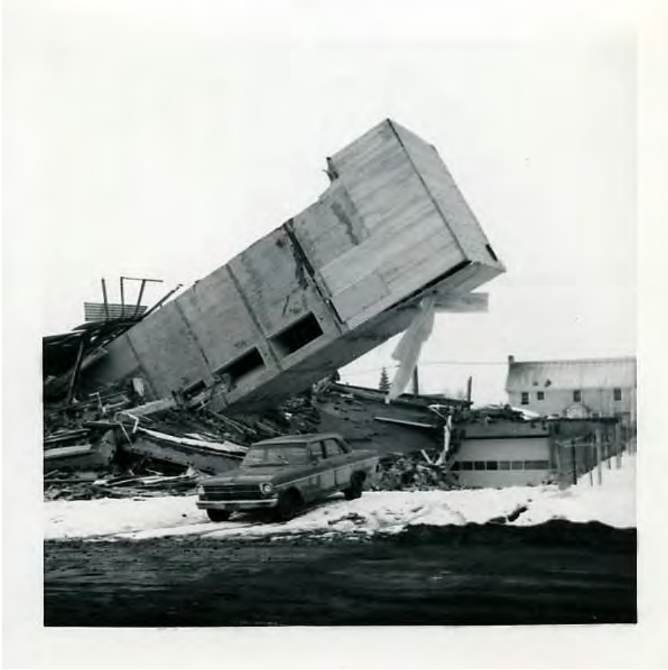
Figure 20. The six-story Four Seasons Apartment building in downtown Anchorage; it completely collapsed with only the elevator shaft remaining intact, 1964 (source: University of Alaska Anchorage, Consortium Library, Archives & Special Collections, Edith and Edward Lindsay papers, 1964, UAA-HMC-1135-p7).
