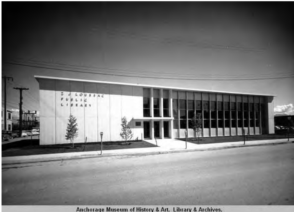
Figure 141. The original Z.J. Loussac Library, 1955, F Street, Anchorage, Alaska (source: Anchorage Museum at Rasmuson Center, Ward Wells Collection, AMRC-wws-1640-2).
