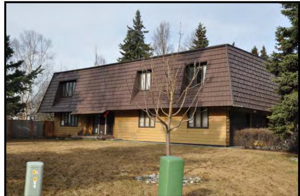
Residential Building, Geneva Woods, Anchorage
