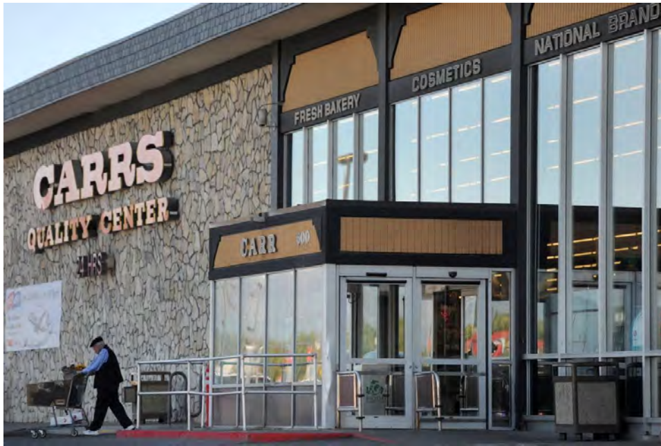
Figure 65. Example of open front commercial building, 600 E. Northern Lights Blvd., Anchorage; Built 1968 (source, Washington Post, 2016).
