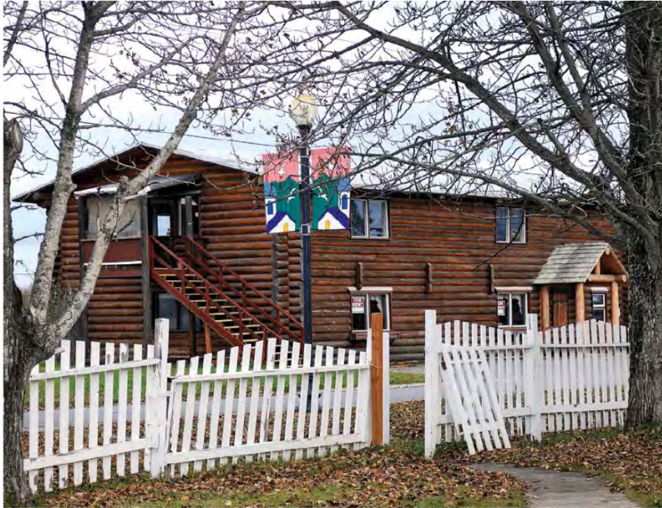
Figure 74. Fort Kenay in Old Town Kenai, extant (source: Brown 2015).
