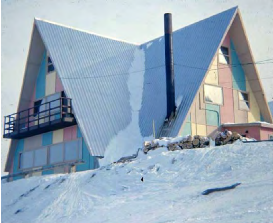
Figure 48. Cleary Summit Ski Lodge on the Steese Highway, 1966; built in 1960 with an aluminum roof but longer extant (source: University of Alaska Anchorage, Consortium Library, Archives & Special Collections, Alfred and Mae Bakken slides and memorabilia, UAA-hmc-0589-4-107).
