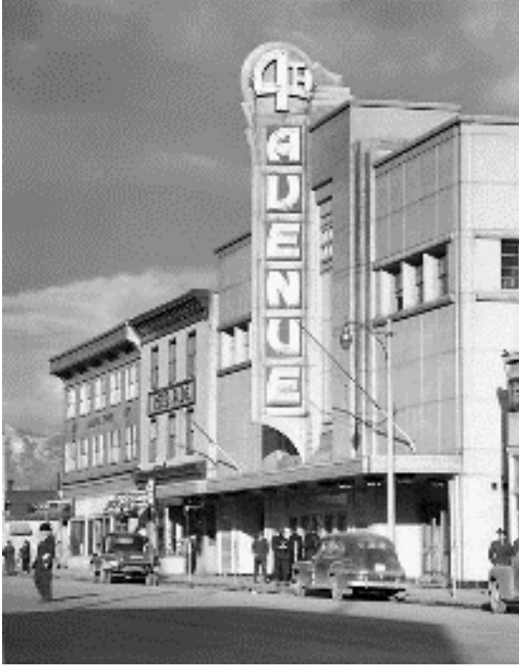
Figure 41. The facade of the Fourth Avenue Theater in Anchorage is made of reinforced concrete, 1949 (source: Anchorage Museum at Rasmuson Center, Sidney Hamilton Photograph Collection, Gift of Emily Turner, B1976.82.31).
