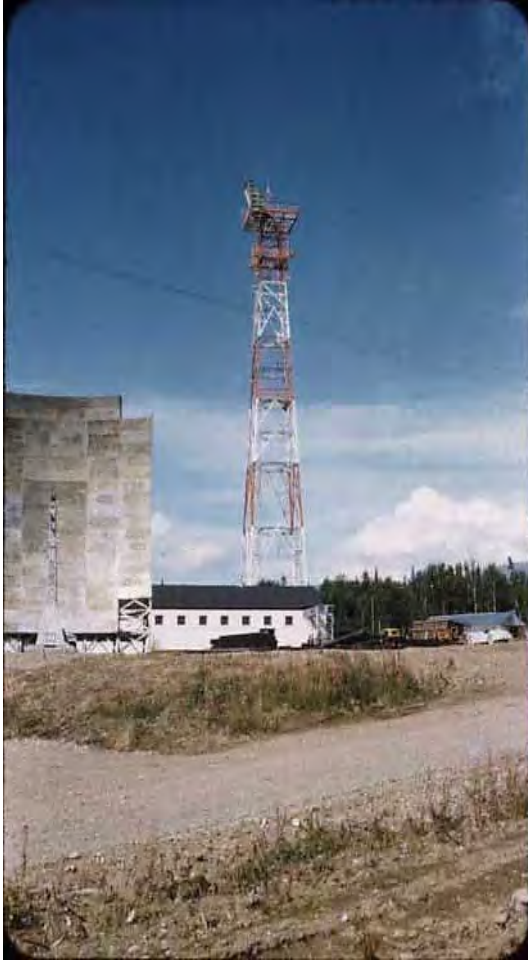
Figure 6. White Alice Communications Site at Wasilla, 1955, with microwave tower and tropo antenna; no longer extant (source: University of Alaska Anchorage, Consortium Library, Archives & Special Collections, Leland A. Olson papers, 1955-1961, UAA-HMC-1064).
