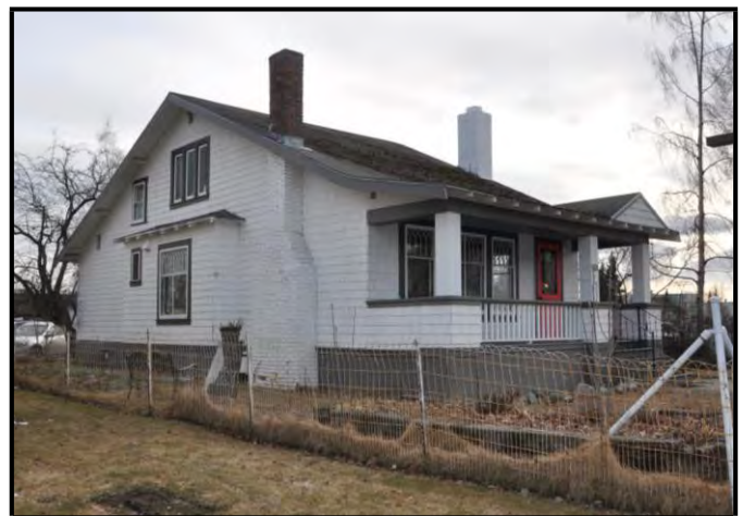
Residential Building, Downtown Anchorage
