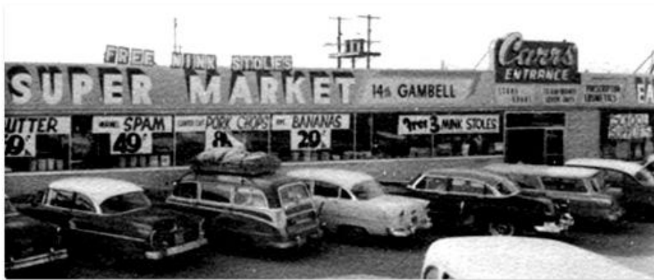
Figure 2: Carrs Supermarket, Gambell Street, Anchorage, date unknown (source: Carrs/Safeway)
