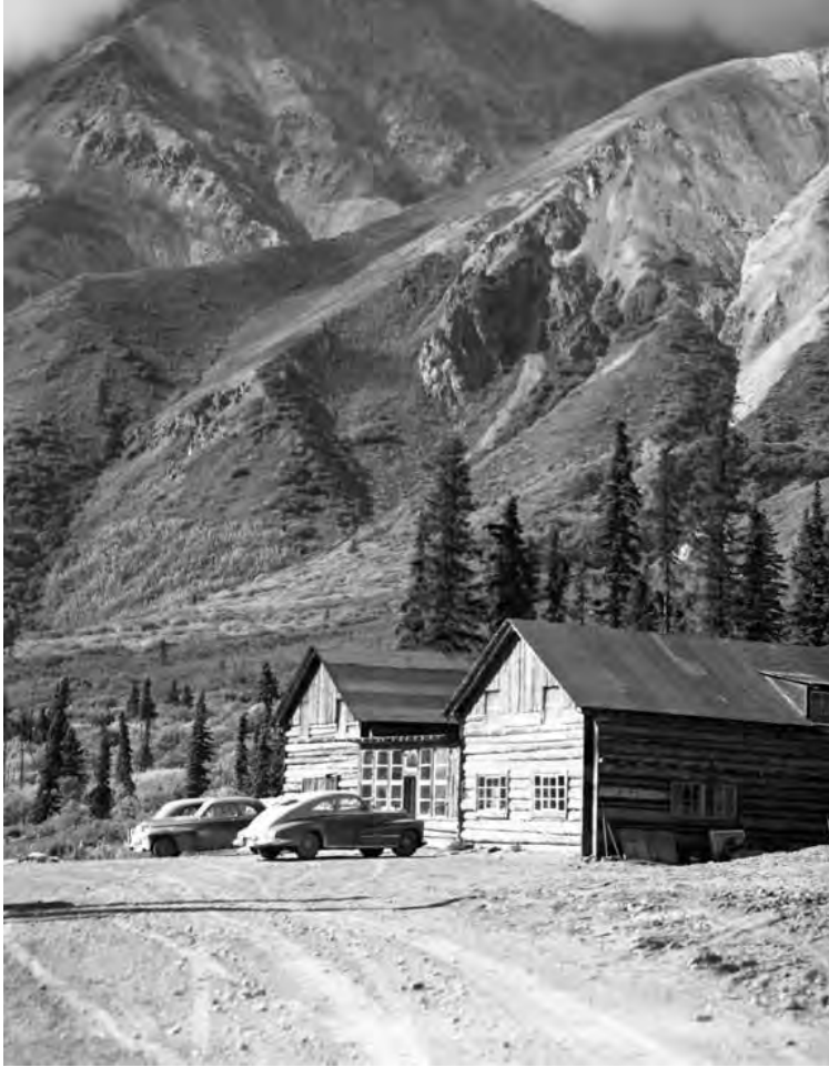
Figure 28. Sheep Mountain Lodge, ca. 1948, extant (source: Anchorage Museum at Rasmuson Center, Sidney Hamilton Photograph Collection, AMRC-B1976-82-271).
