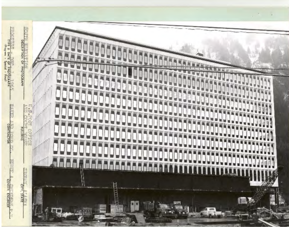
Figure 79. US Post Office and Courthouse, Juneau, Alaska, 1966, extant (source: History of the Federal Judiciary 2016).
