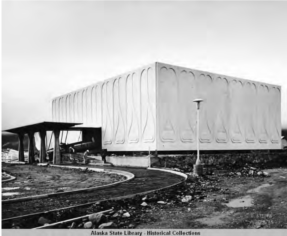
Figure 73. Alaska State (Centennial) Museum, Juneau, demolished (source: Alaska State Library - Historical Collections, Don Steffa Photograph Collection, ca. 1958-1977, ASL-P283-2-451 ).
