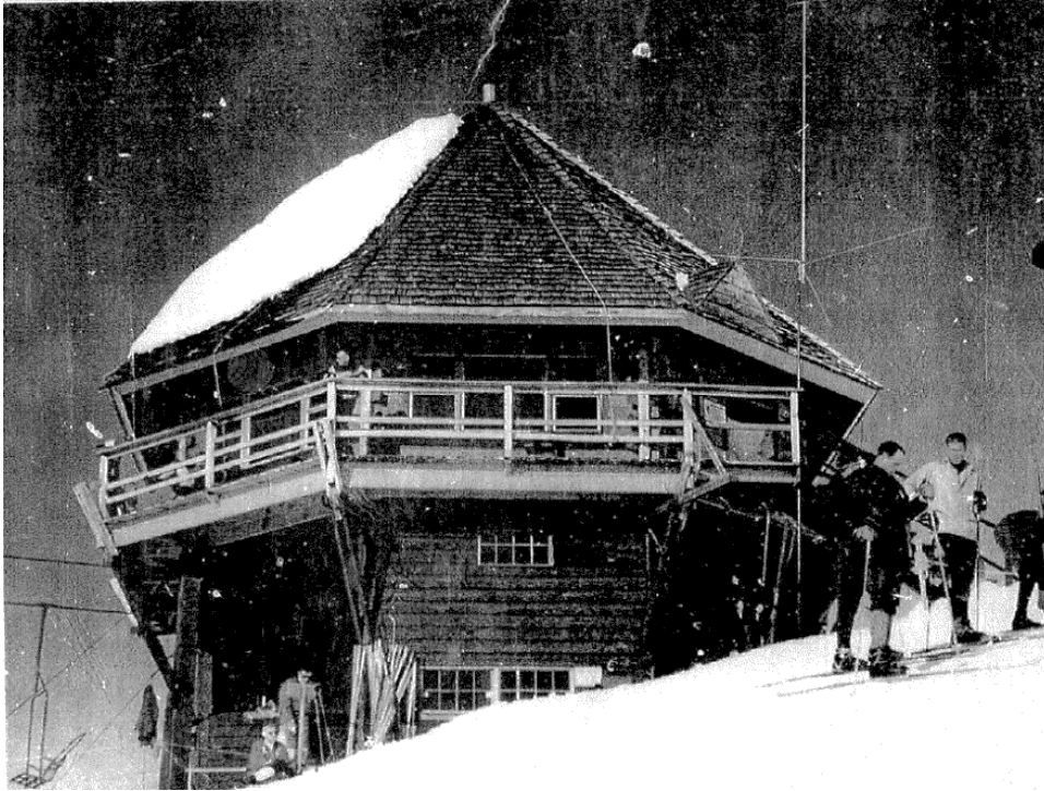
Figure 116. The Mount Alyeska Round House, ca. 1960, extant and restored (source: National Register Nomination 2002).
