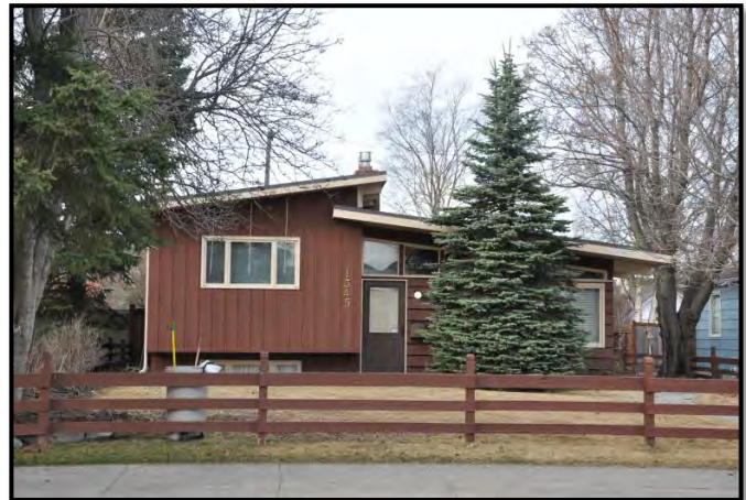
Residential Building, South Addition, Anchorage
