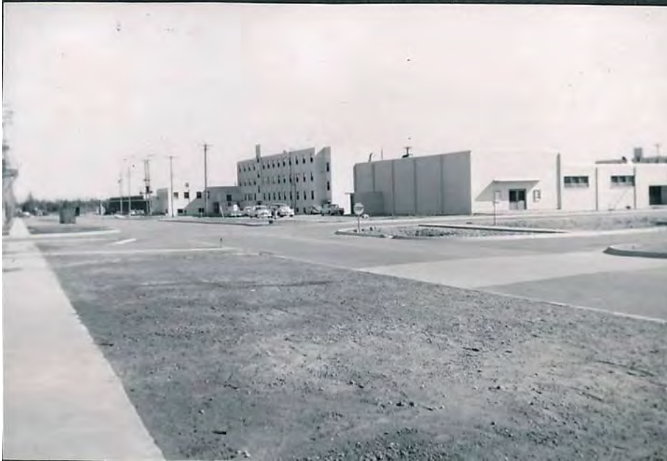
Figure 10. Fort Greely, near Delta Junction, 1957 (source: University of Alaska Anchorage, Consortium Library, Archives & Special Collections, Grace P. Hurst photograph album, 1957, UAA-HMC-0914-17d).
