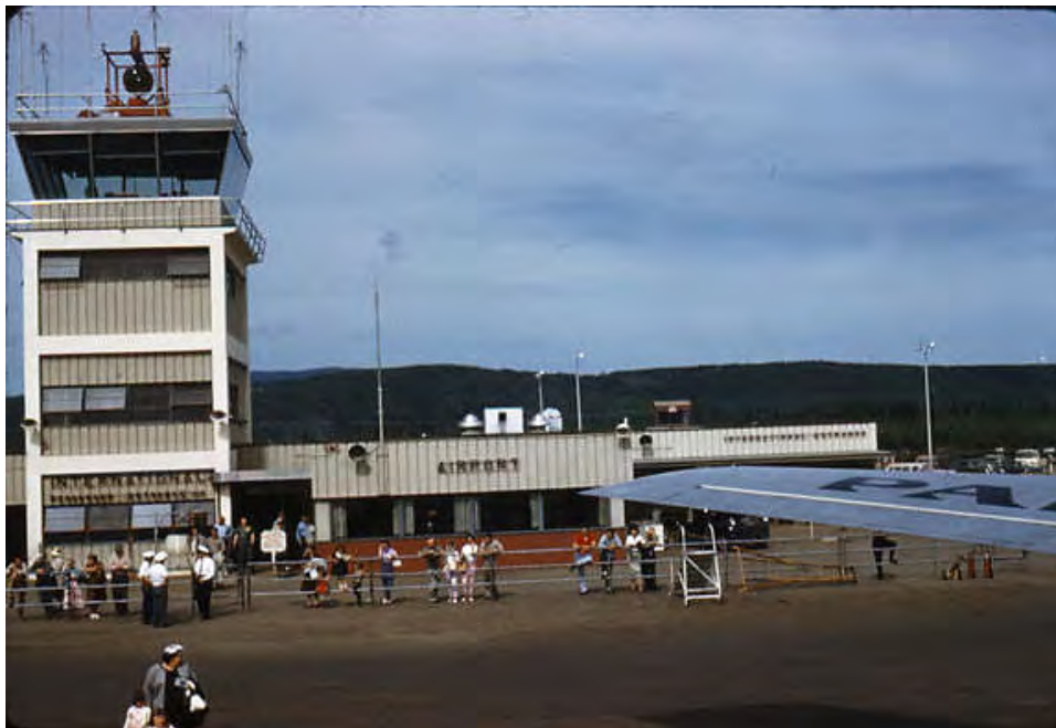
Figure 86. Fairbanks International Airport Terminal and Control Tower, 1961 (University of Alaska Anchorage. Consortium Library. Archives & Special Collections, Donald Arthur Post slides, 1953-1959, UAA-hmc-0917-619).
