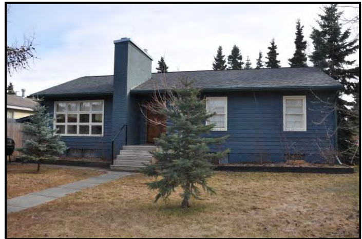
Residential Building, South Addition, Anchorage
