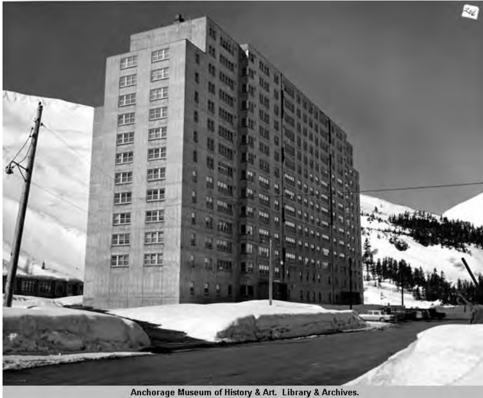
Figure 59. The Hodge Building, Whittier, a high-rise apartment building, as seen in 1964 (AMRC-b79-38-23).
