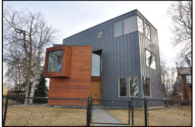
Residential Building, South Addition, Anchorage
