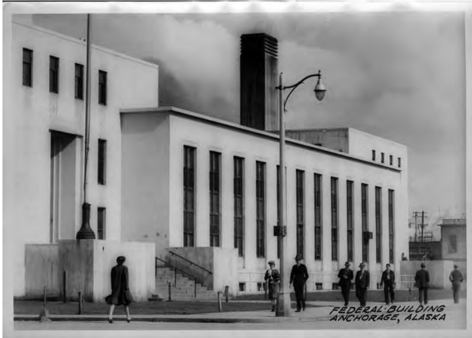
Figure 154. The Anchorage Federal Building, 4th Avenue, 1942 (source: Anchorage Museum at Rasmuson Center, Sidney Hamilton Photograph Collection, Anchorage Museum, Gift of Emily Turner, B1976.82.879, AMRC-B1976-82-048).
