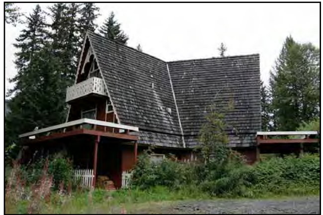
Residential Building, South Addition, Anchorage
