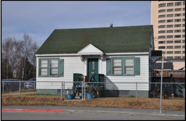
Residential Building, Downtown, Anchorage
