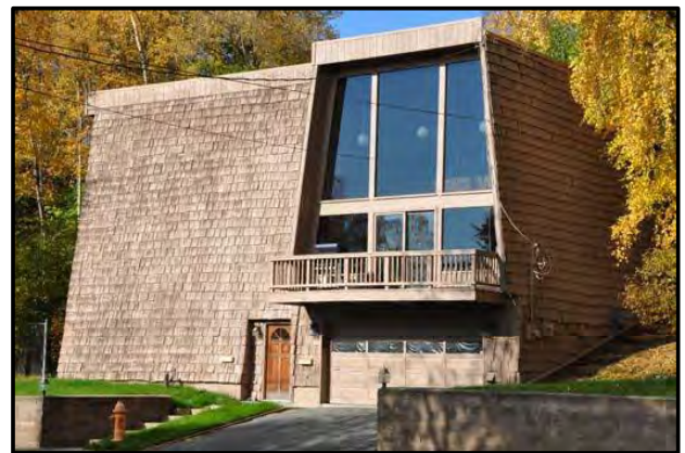
Residential Building, South Addition, Anchorage
