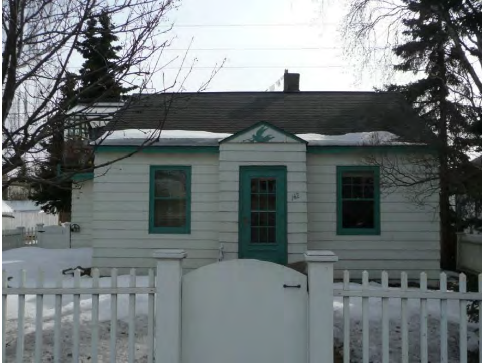
Figure 50. Arctic entry on a residence located at 142 East 10th Avenue, Block 13 Lot 15 in Anchorage's Pilot Row Neighborhood (source: True North SDS 2014).
