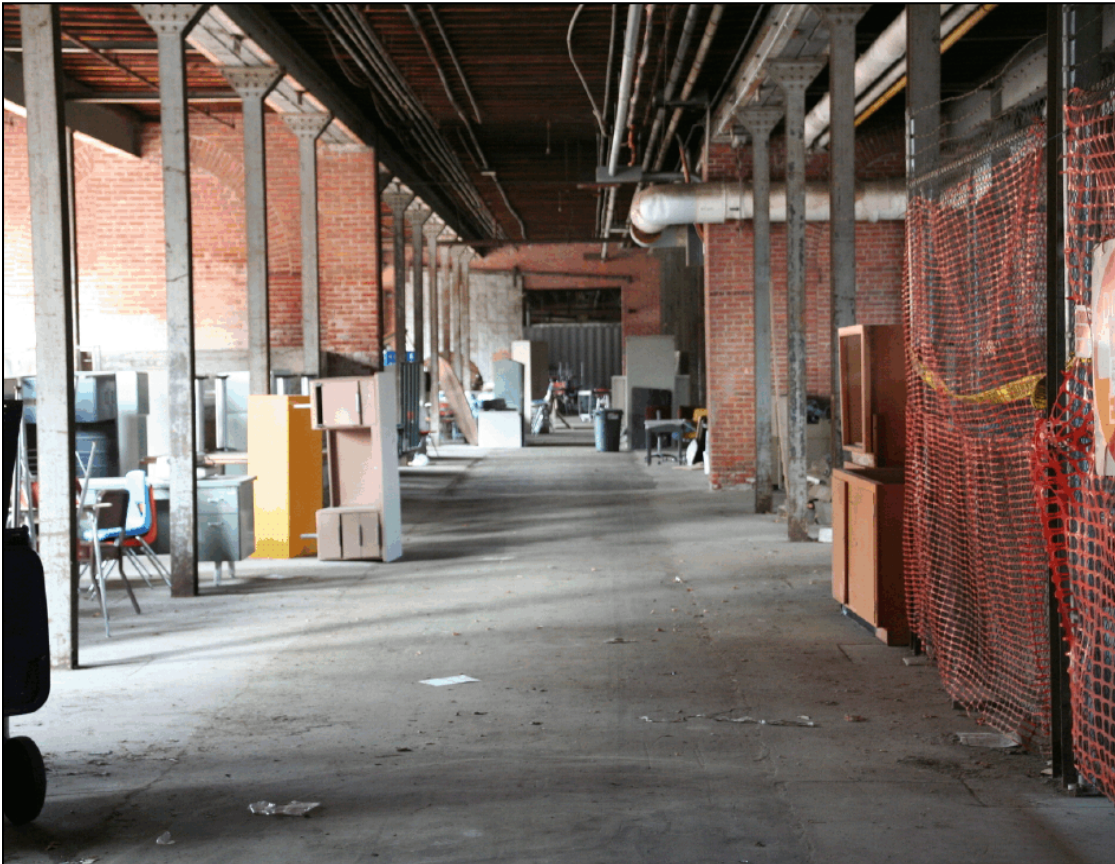
Figure 4.22. In 2005, Building 19 (interior photo) was open to weather, pigeons and vandals, its interior used for storage of miscellaneous objects. In 2009 the concrete barriers were gone, leaving the brick piers unprotected from cars and trucks (photos: author).
