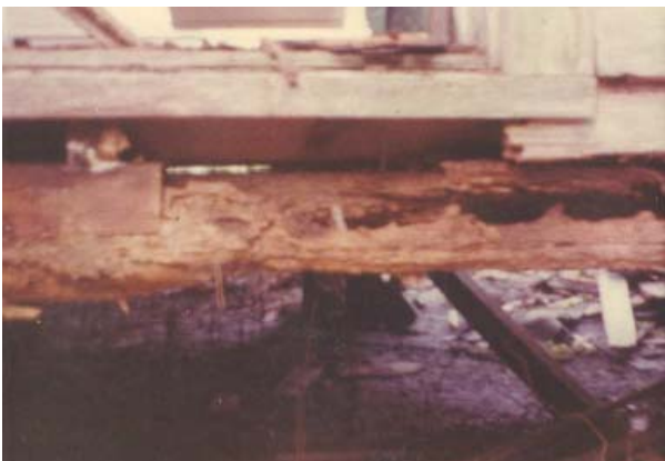
Figure 32. Termites in sill, 1979. (CALO Polaroid album)
