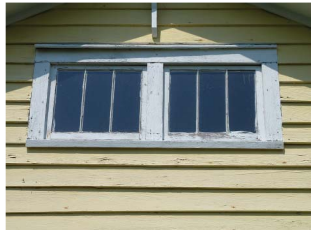
Figure 74. Casement windows in east gable. Those in the dormer are similar.
