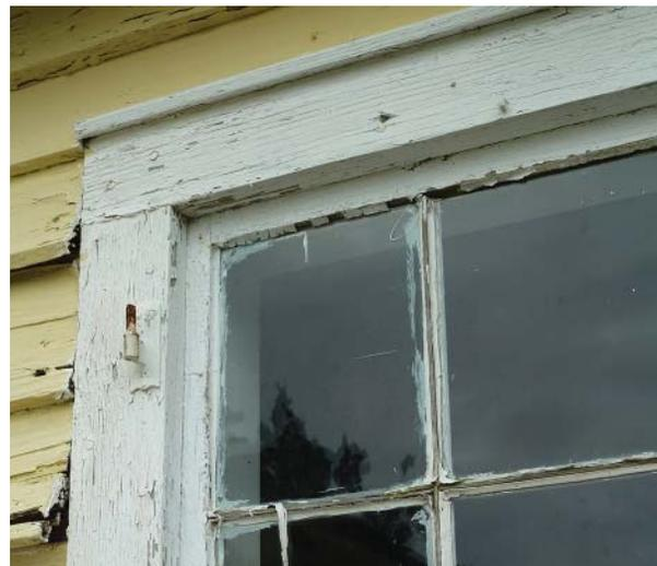
**Figure 77.** Casing and drip cap typical of all windows, and shutter pintle similar to those found at some older window openings.
