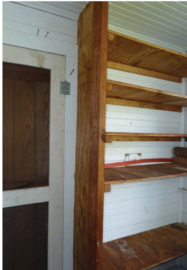
Figure 103. View of north wall of Room 104.
