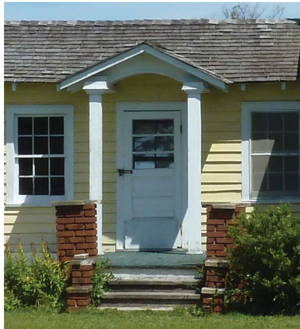
Figure 131. Tilted brick cheek wall at steps to front deck.
