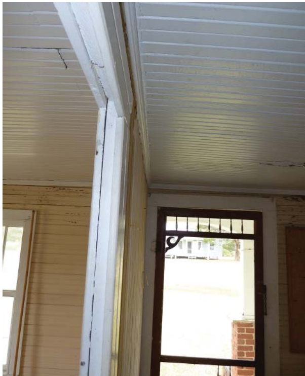
Figure 94. Wall between Rooms 101 and 102.
