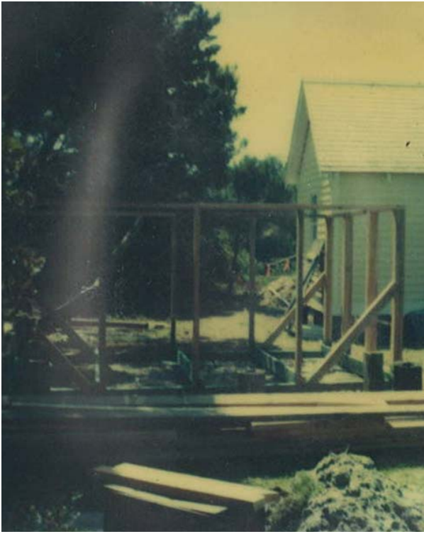
Figure 41. Reconstructed frame for rebuilt shed, 1980. (CALO Polaroid album)
