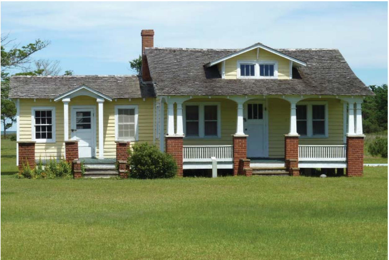
Figure 85. Front (south) elevation.
