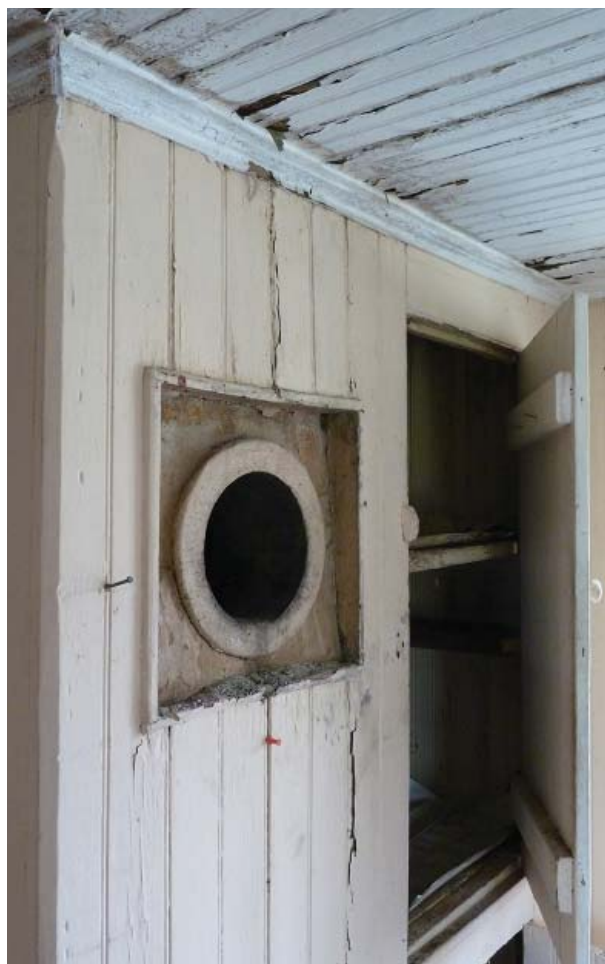
Figure 118. Stove flue and upper door of pantry closet.
