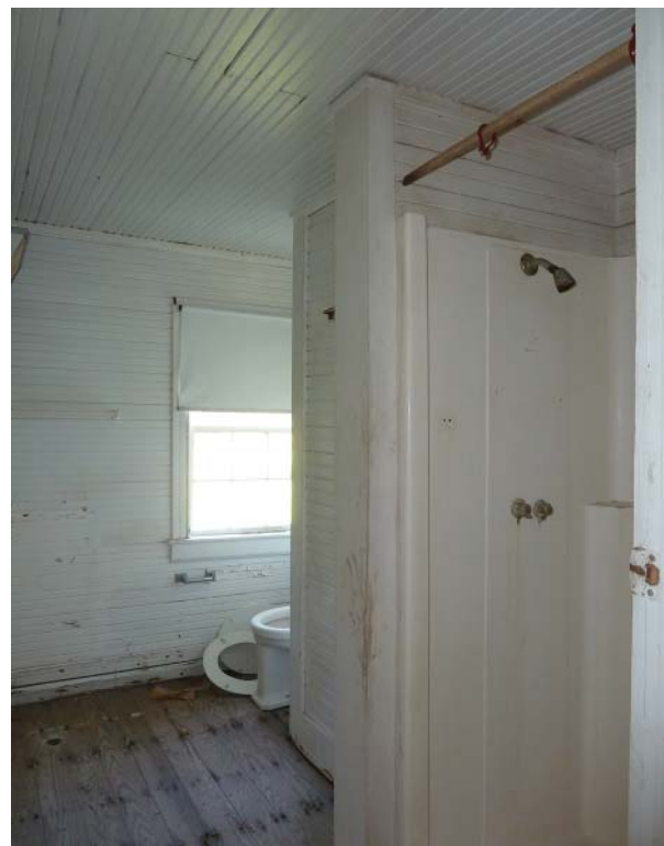
Figure 99. Looking east in Room 103.
