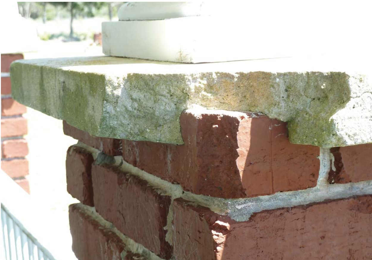
Figure 61. Typical materials in brick piers.
