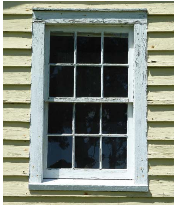
Figure 76. Typical six-over-six window installed in the 1960s.
