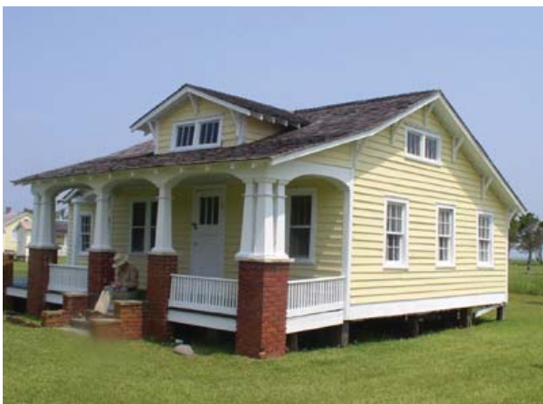
Figure 46. Front and east elevations in 2007. (NPS List of Classified Structures [LCS])
