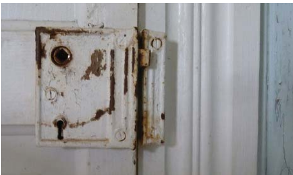
Figure 111. Rim lock on door between Rooms 105 and 101.
