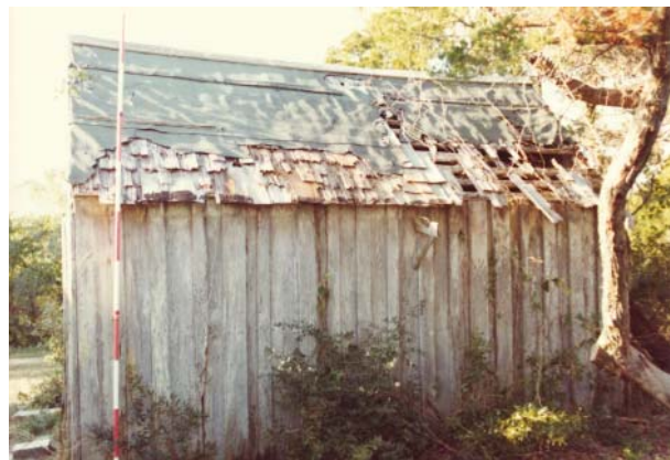
Figure 40. East side of shed before work, 1979. (CALO Coll. f290)
