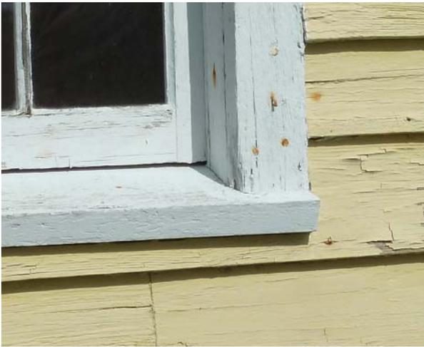
Figure 78. Typical casing and sill.
