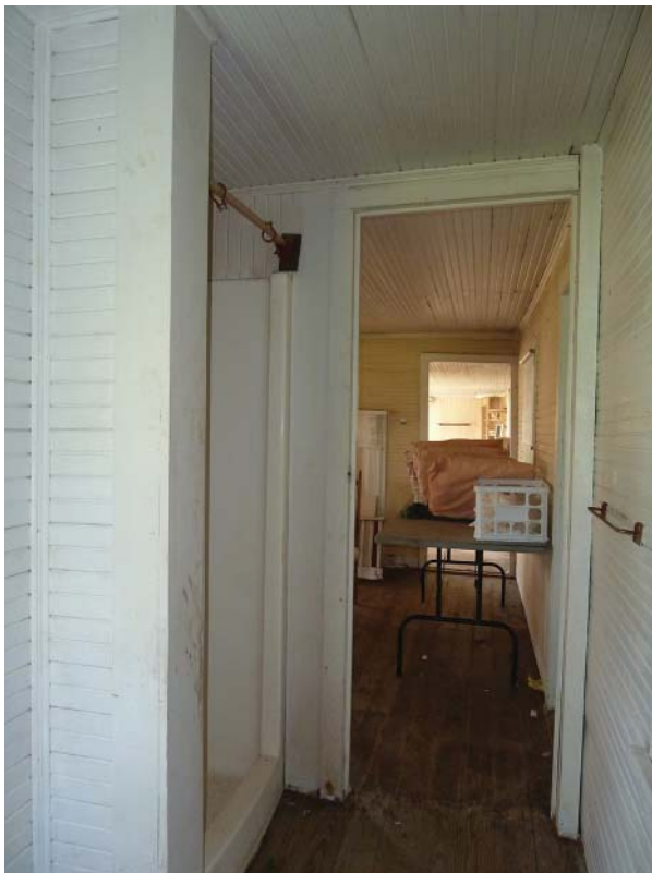
Figure 100. Looking west from Room 103 to Room 101.
