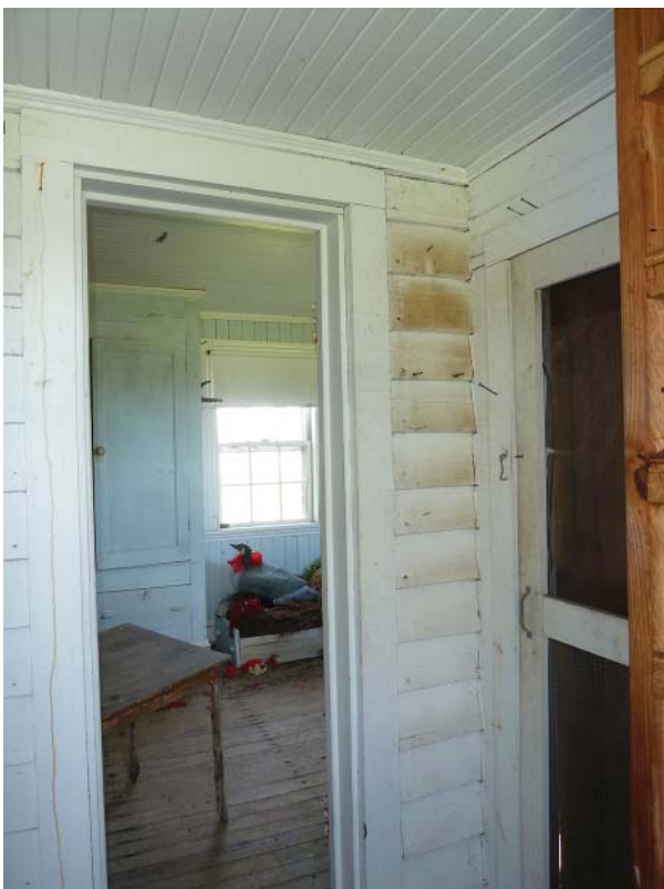
Figure 102. View from Room 104 into Room 105.
