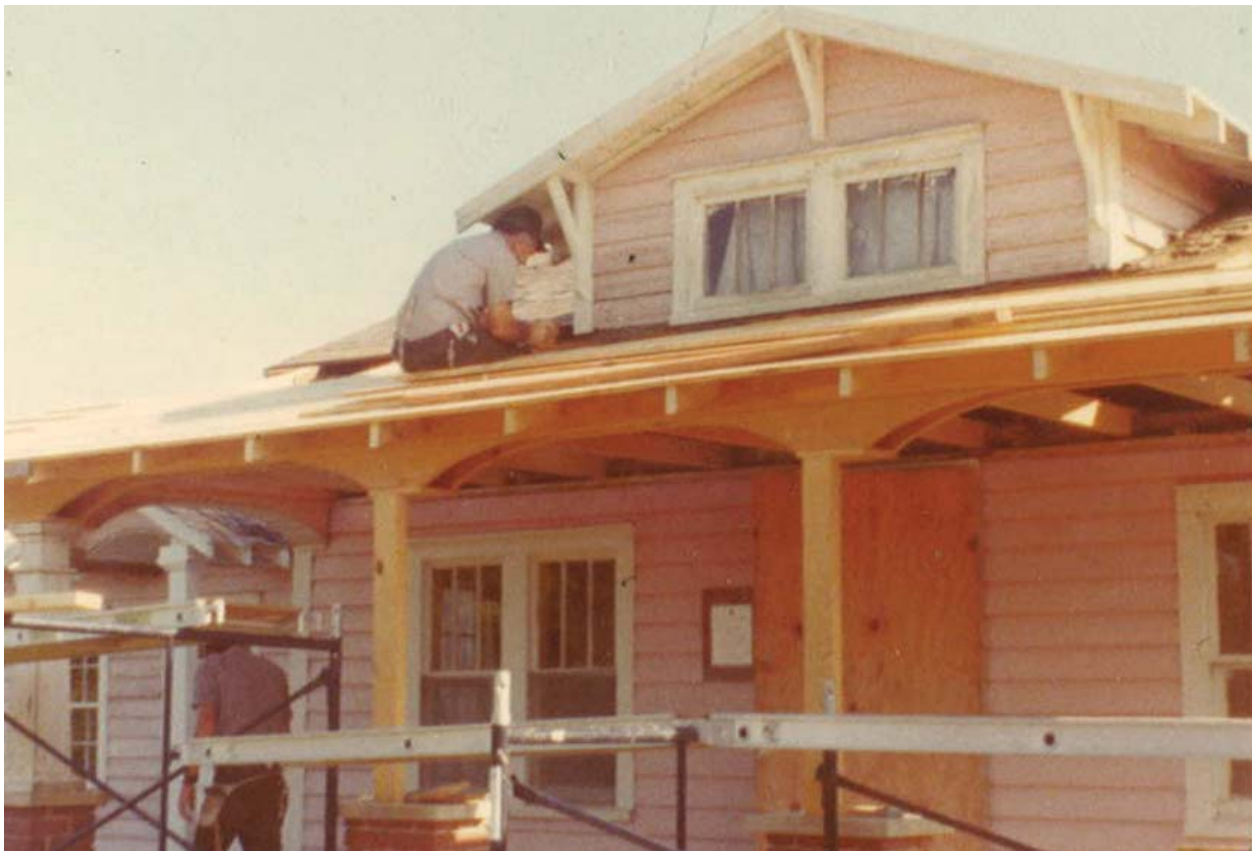
Figure 36. Replacing porch roof, arches, posts, 1979. (CALO Polaroid album)
