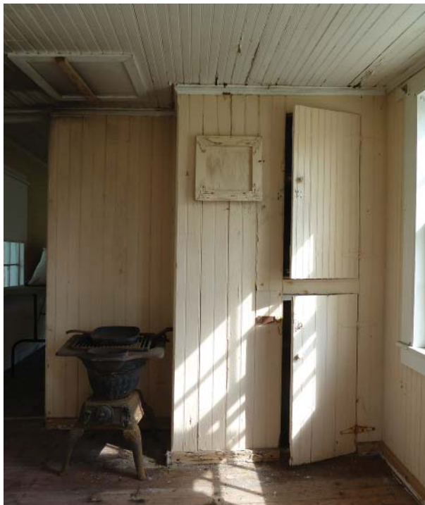
Figure 113. Looking east in Room 106, showing floor-to-ceiling pantry closet.
