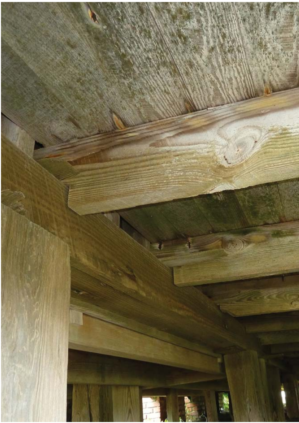
Figure 63. Typical joist/stud/sill/post connections.
