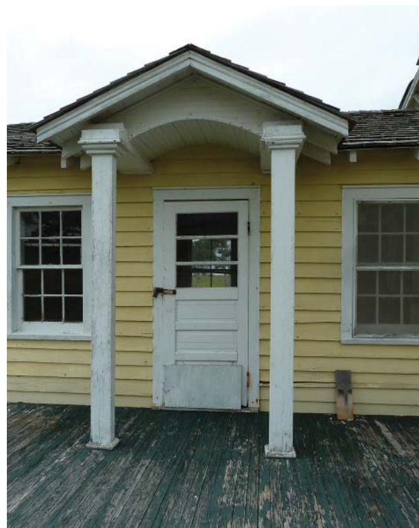
Figure 87. View of portico added to west wing as part of the ca. 1928 remodeling.
