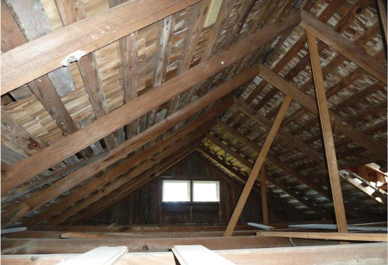
**Figure 68.** Looking east, showing roof framing and ceiling joists above the main block of the house.
