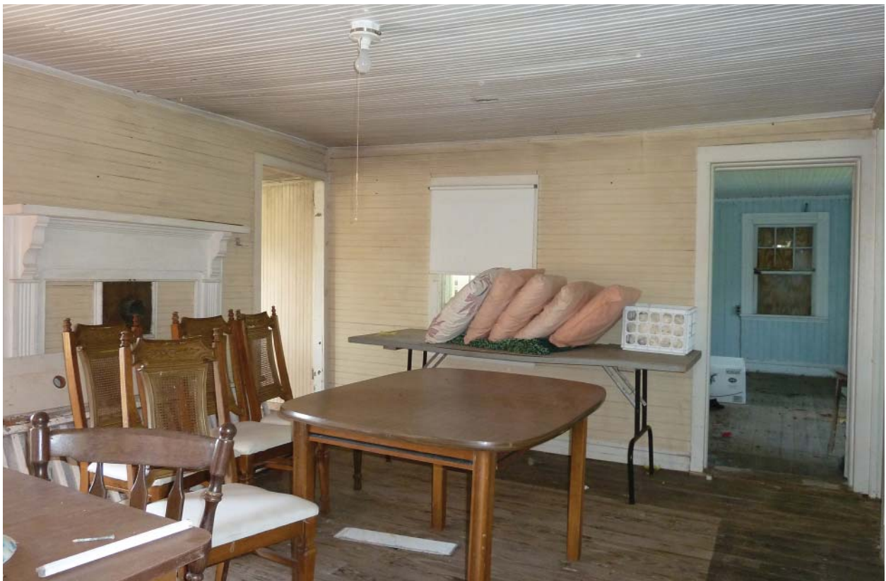
Figure 93. Northwest oblique, Room 101.
