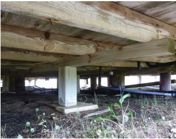
Figure 57. Added supports on west side of main block.
