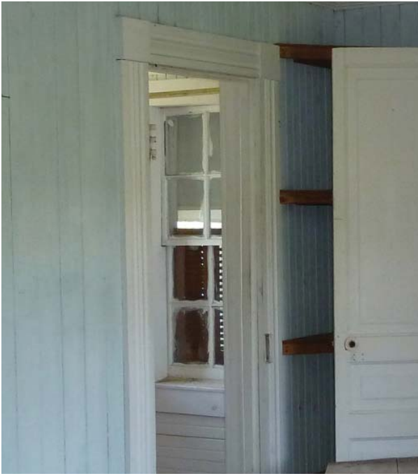
Figure 19. Doorway from north wing to added northeast entrance room, now a storage room. Originally an exterior doorway, it retains the Victorian trim found in the wing. (2013 photograph)
