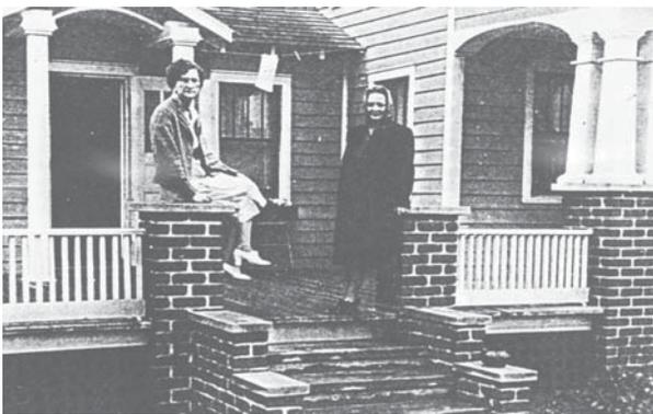
**Figure 24.** Lida Dixon & Rita Woolard on "kitchen porch," showing the vertical-light sash in the west window of the main block, the new sash and door of the west wing, and the screen door opening to the interior, a distinctive Portsmouth feature. (undated, CALO f74, Linda Robertson Hudson Coll.)
