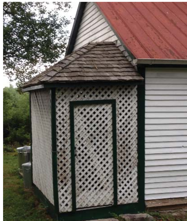
Figure 21. A lattice vegetable house in western North Carolina with exterior door and no access to its associated building.
