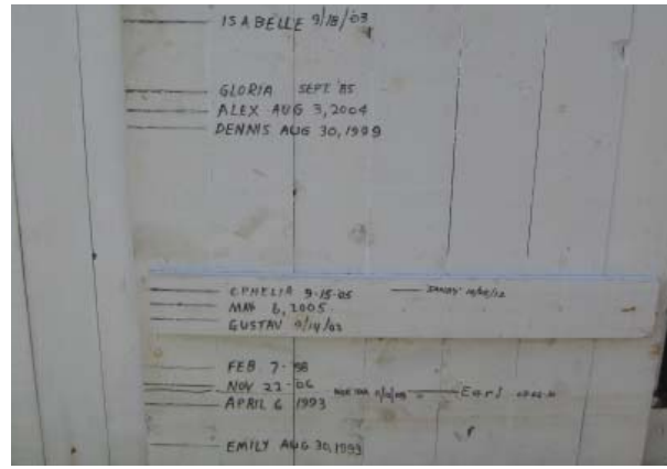
Figure 51. Record of high water marks from storm surge flooding on Theo Salter House shed (NPS 519).
