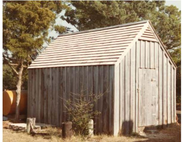
**Figure 43.** Rebuilt shed with louvered vent in gable end, photographed 1983. (CALO Coll. f295)
