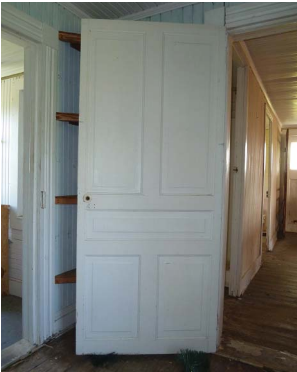
Figure 110. Five-panel door between Rooms 101 and 105.
