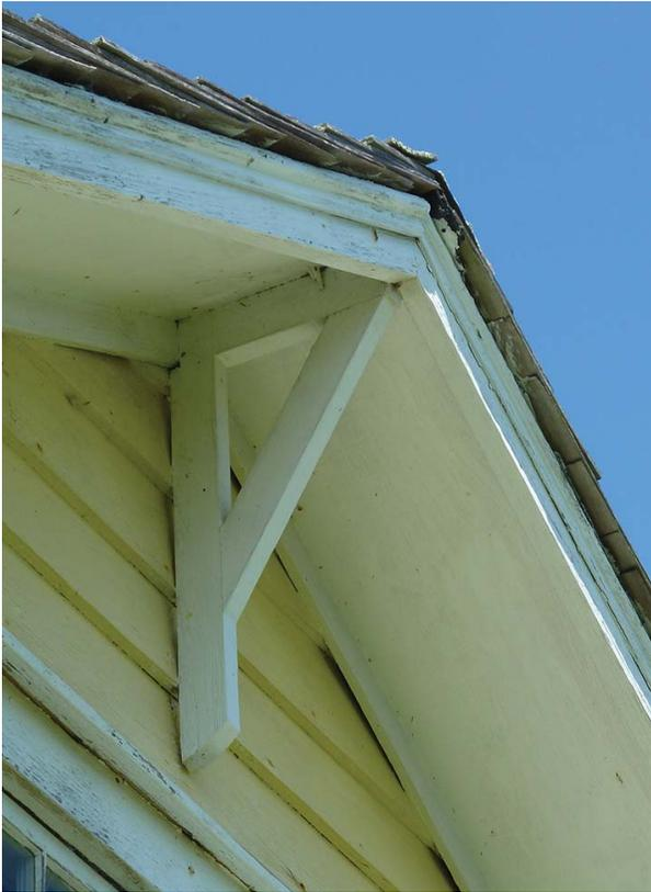
**Figure 84.** Typical knee brace, rake board, siding and other trim.
