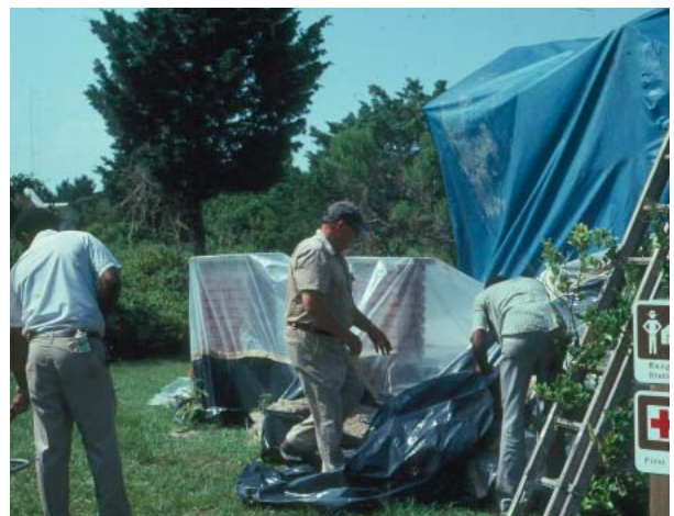
Figure 44. West wing and deck piers wrapped for fumigation project, July 1981. Ranger station sign in front of house. (CALO acc. 05537)
