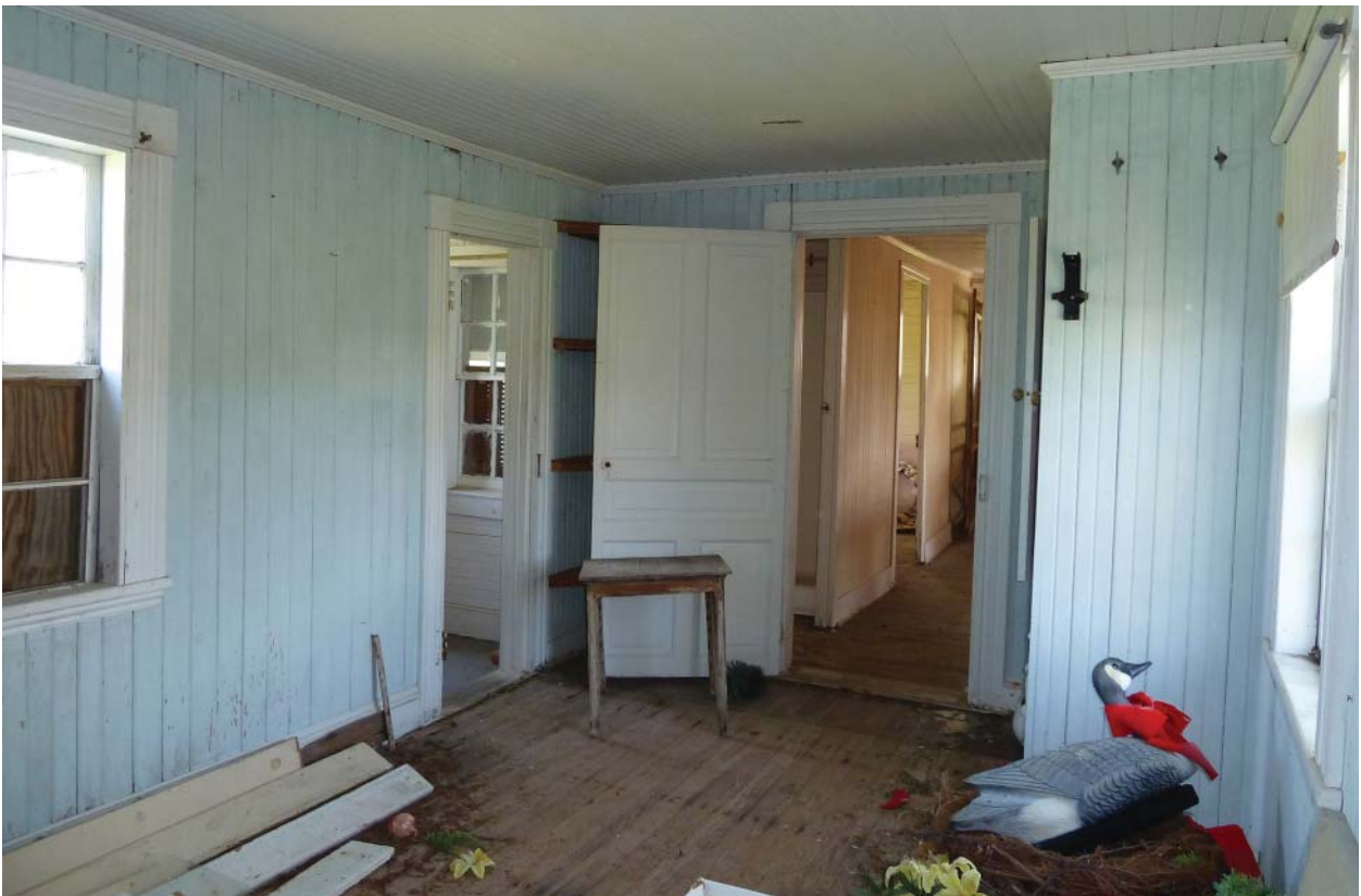
Figure 106. Looking south in Room 105.
