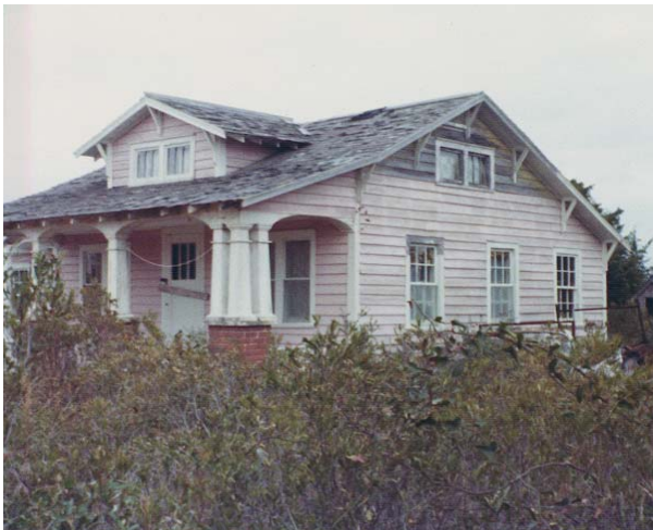
Figure 45. Front and east elevations in 1977. Privy is visible in the background. (CALO Coll. f83)
