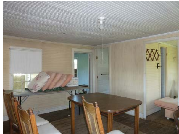
Figure 95. Northeast oblique, Room 101.
