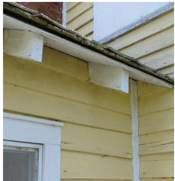
Figure 81. Typical exposed rafter tails.
