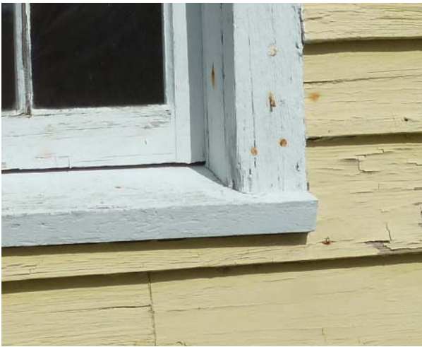
Figure 78. Typical casing and sill.
