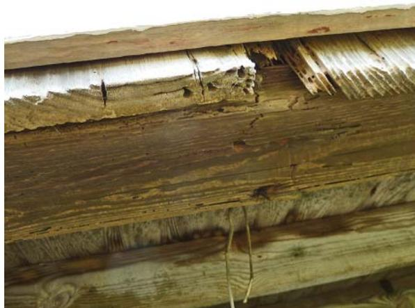
**Figure 66.** Typical sill and bottom ends of vertical sheathing on the main block of the house.
