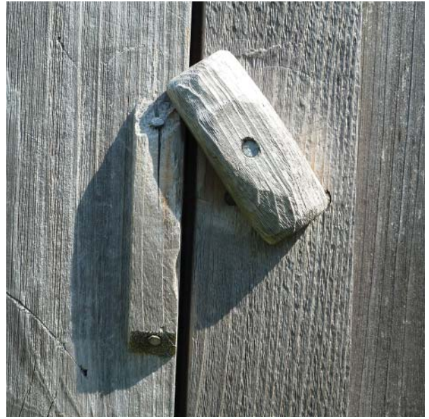
Figure 127. Pivot latch on shed door.
