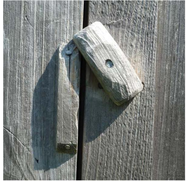
Figure 127. Pivot latch on shed door.
