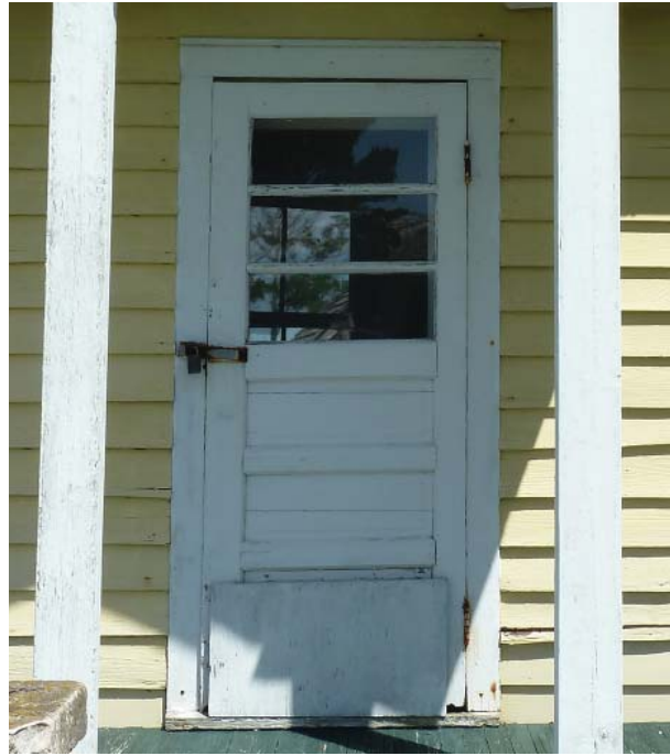
Figure 70. Front door to kitchen (west) wing.
