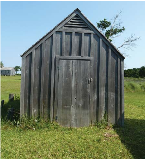
Figure 121. South elevation of shed.
