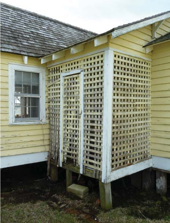
Figure 88. Lattice room at northwest corner.
