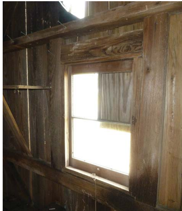
Figure 124. Window at north shed wall.
