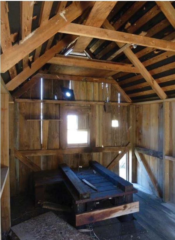
Figure 126. Looking north inside shed.
