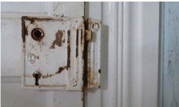
Figure 111. Rim lock on door between Rooms 105 and 101.
