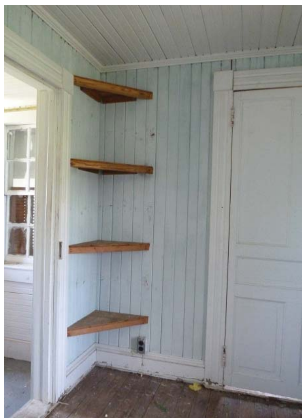
Figure 108. Modern shelving in southeast corner of Room 105.
