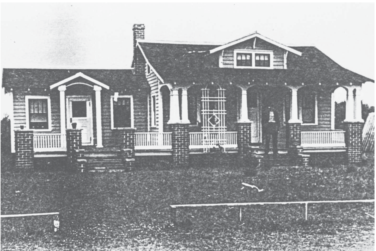
Figure 22. Undated photograph of Tom Bragg on the steps of the Dixon House, showing the 1928 changes to the front of the house, including the dormer, engaged porch roof, porch posts on piers, railings, paired windows, vertical-glazed doors and sash, west portico and deck, steps and cheek walls. This view of the exterior end chimney illustrates the depth of the newly extended eaves. (CALO f75, Linda Robertson Hudson Coll.)
