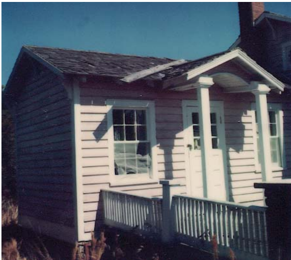
Figure 31. West wing and stepped railing in 1977. (CALO Coll. f80)
