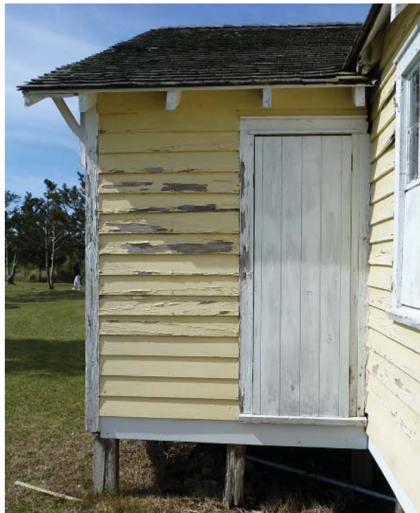
Figure 71. Back door, opening to Room 104.
