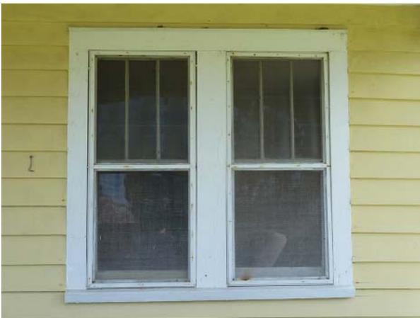
**Figure 73.** Paired three-over-one windows on the front porch.
