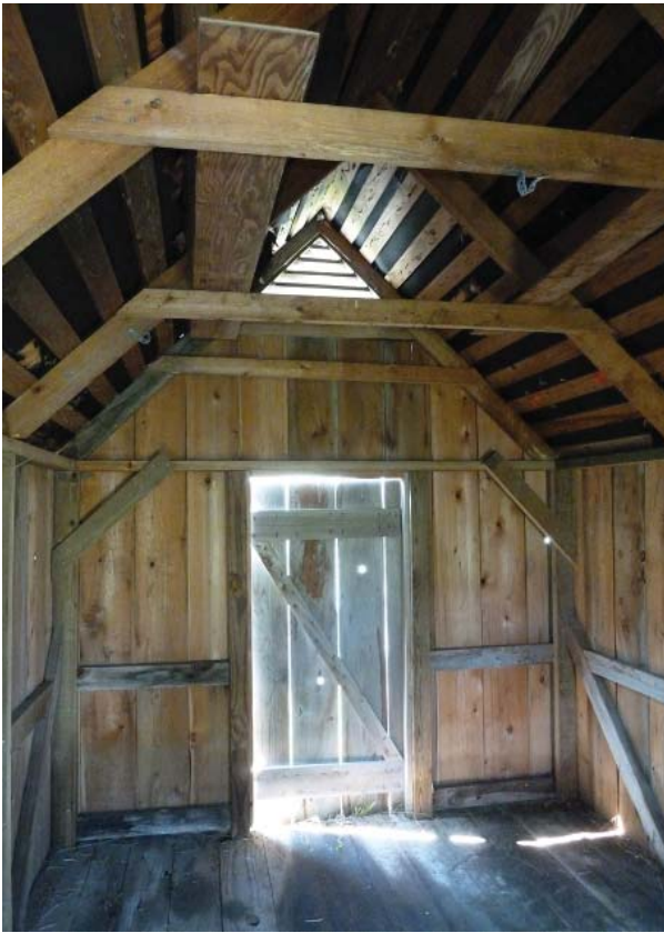
Figure 125. Looking south inside shed.
