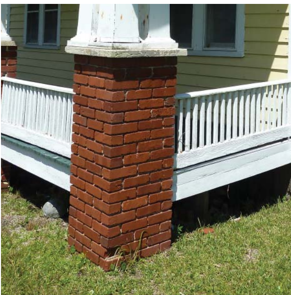
Figure 59. L-shaped pier at southeast corner of front porch.
