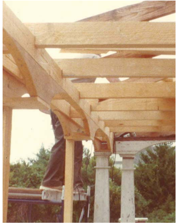
Figure 35. Replacing porch roof framing, 1979. (CALO Polaroid album)
