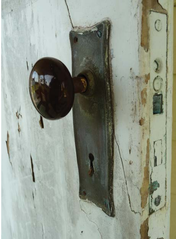
Figure 72. Lock set at front door.
