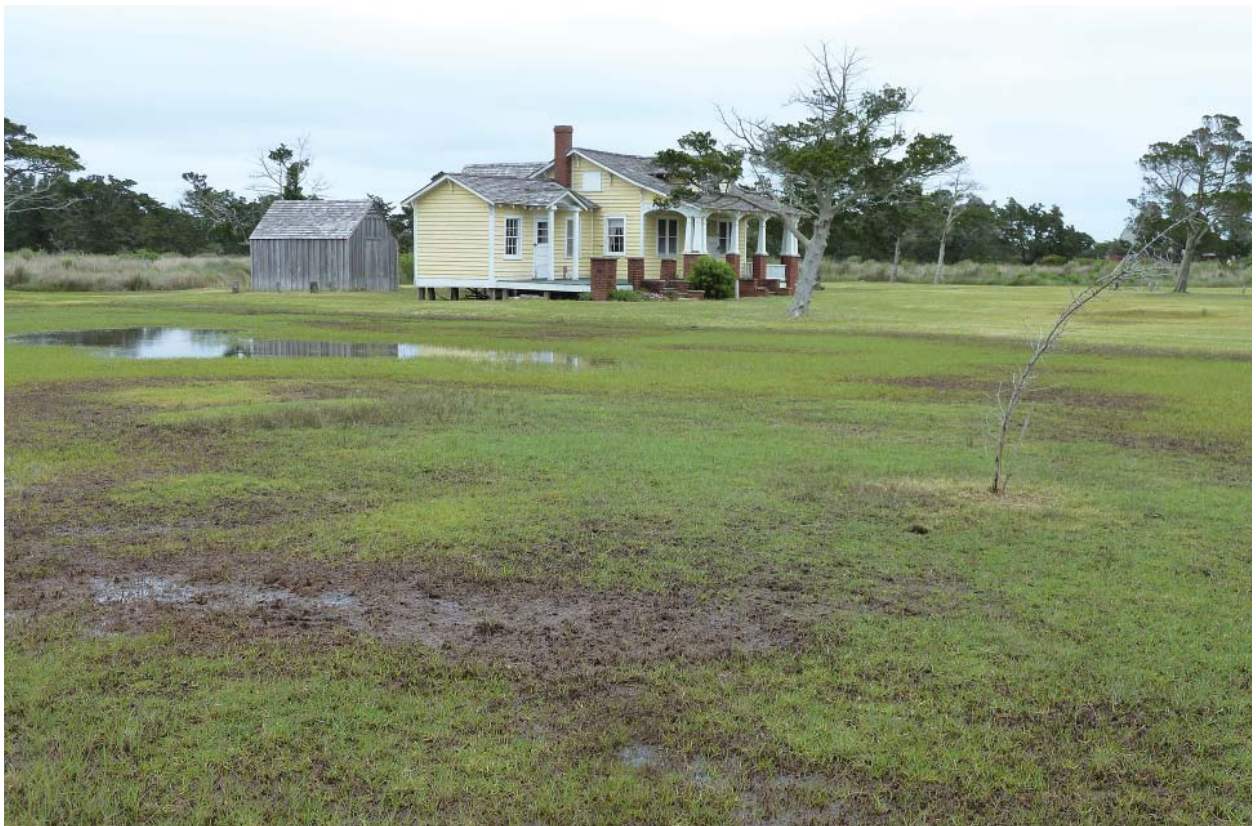
Figure 54. Typical site conditions on the west side of the house.
