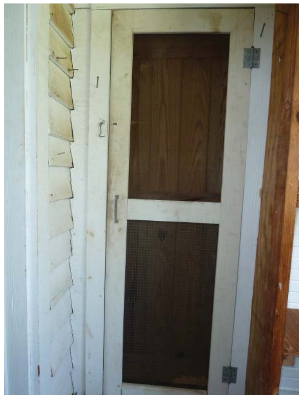
Figure 104. View of interior screen door in Room 104.
