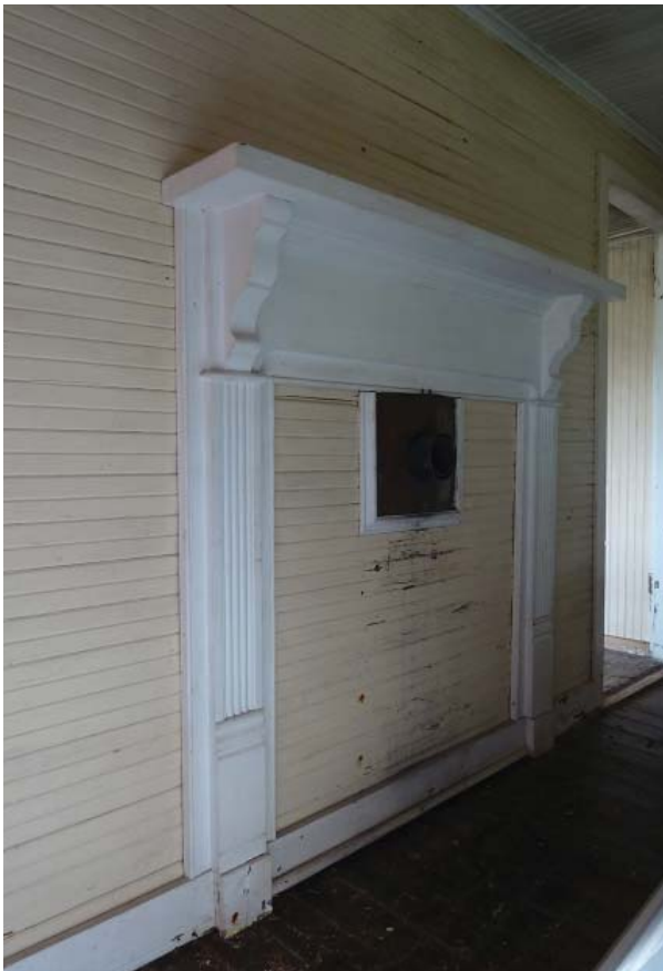
Figure 92. Mantel and stove flue in Room 101.
