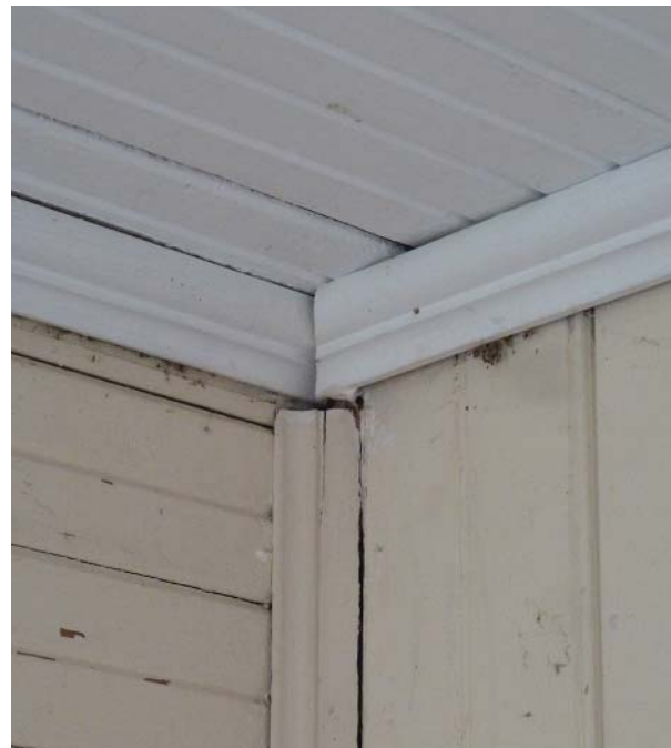
Figure 96. Typical woodwork in Room 101.
