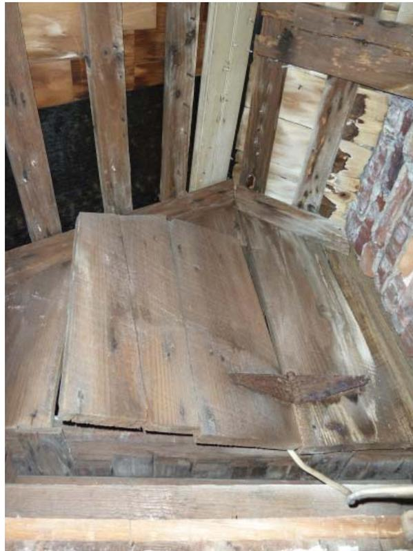
**Figure 18.** Vertical-board siding of the exterior of the original main block, covered when the west wing was brought up and attached. Shown is a door cut into the siding to lead from attic of wing to attic of main block. (2014 photograph)
