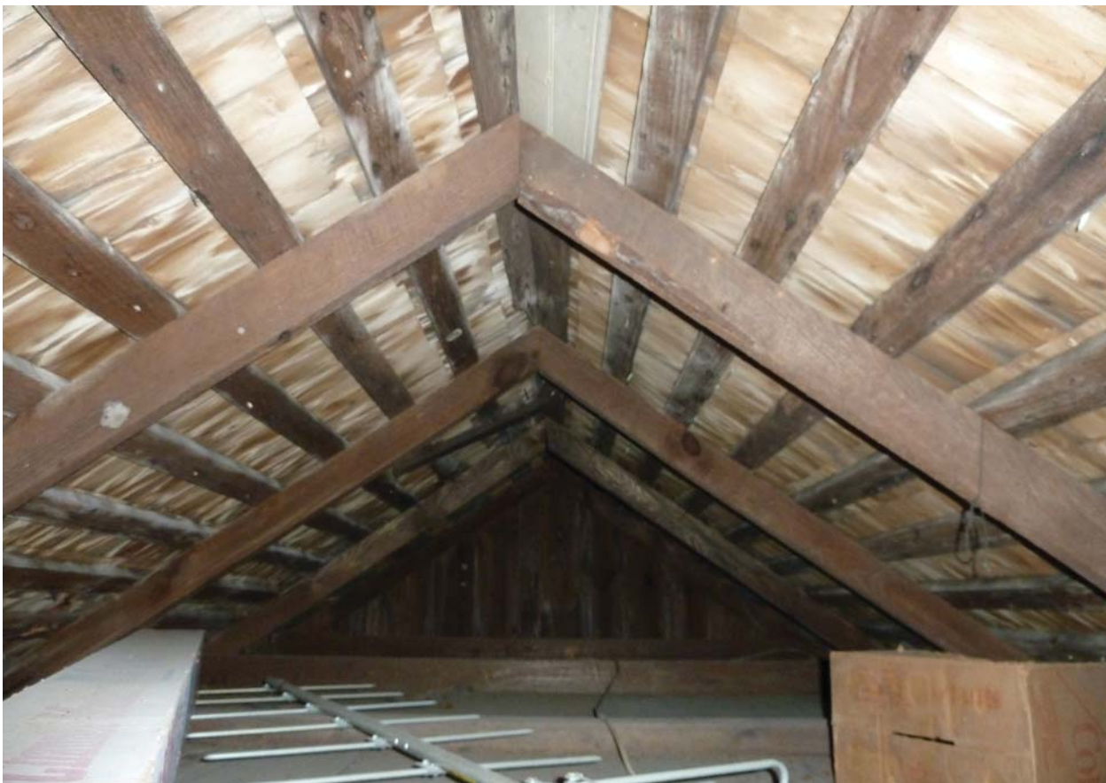
Figure 65. Looking west in attic of kitchen wing.
