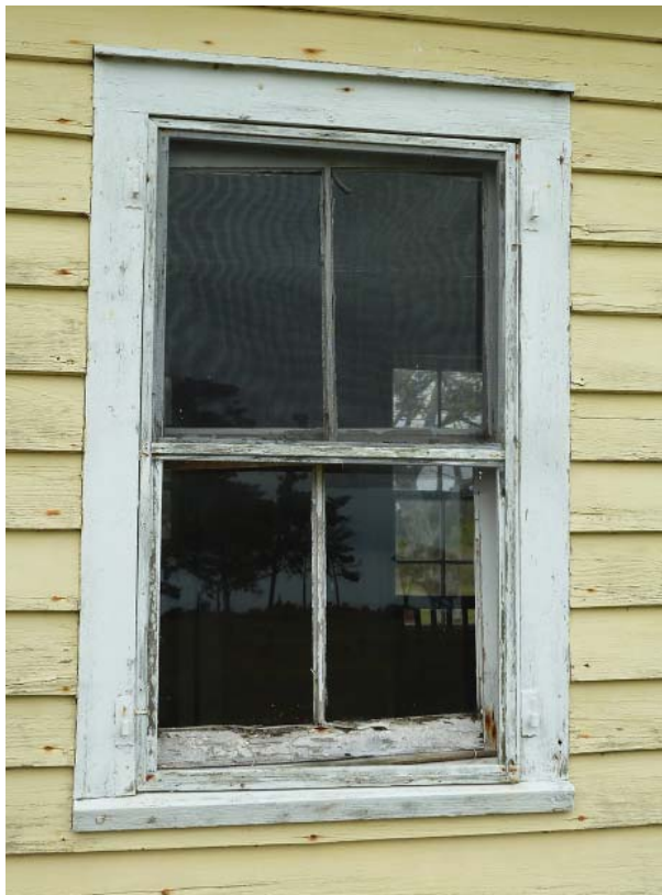
Figure 75. Two-over-two window on the north side of the kitchen wing, the earliest intact window in the house.
