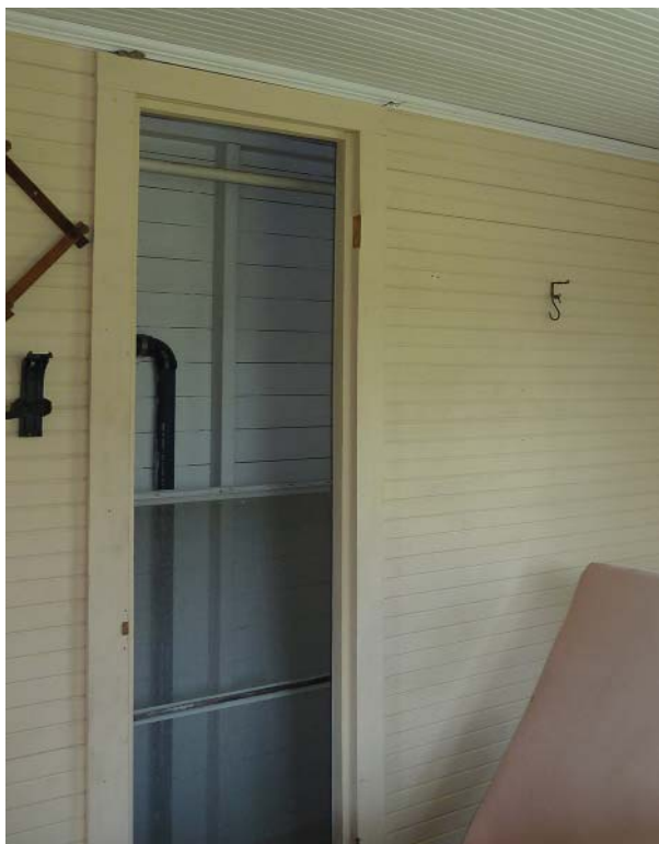
Figure 98. Doorway between Rooms 102 and 103, now blocked by the shower in Room 103.
