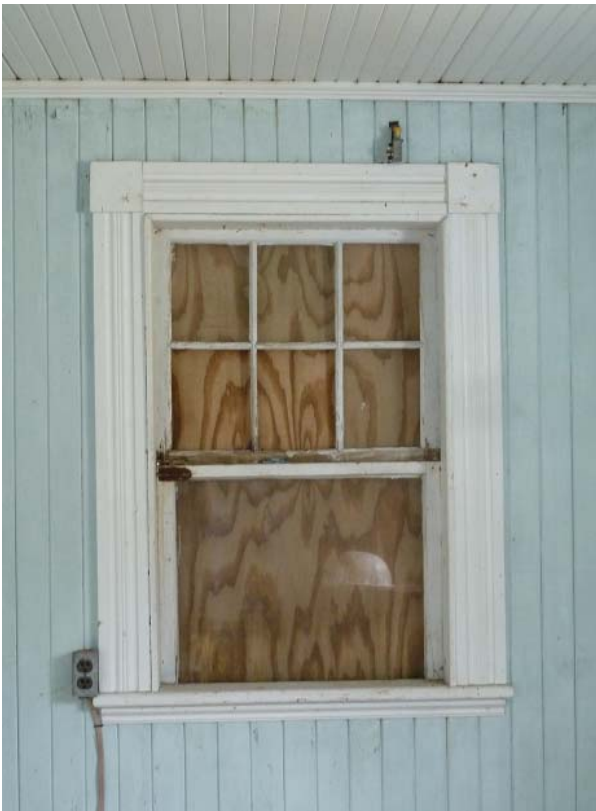
Figure 105. North window showing typical casing and corner blocks used at windows and doors in Room 105.
