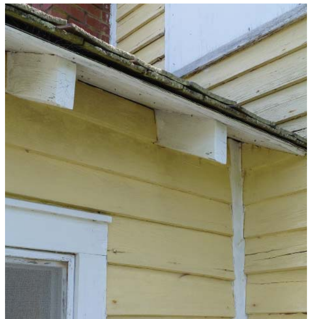
Figure 81. Typical exposed rafter tails.
