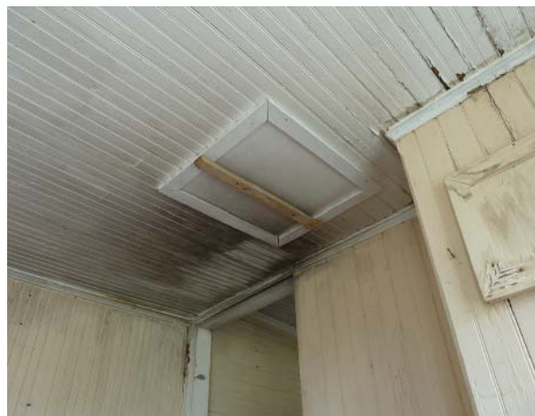
Figure 114. Attic hatch in northeast corner of Room 106.
