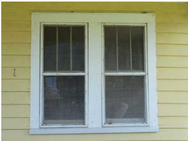
Figure 73. Paired three-over-one windows on the front porch.
