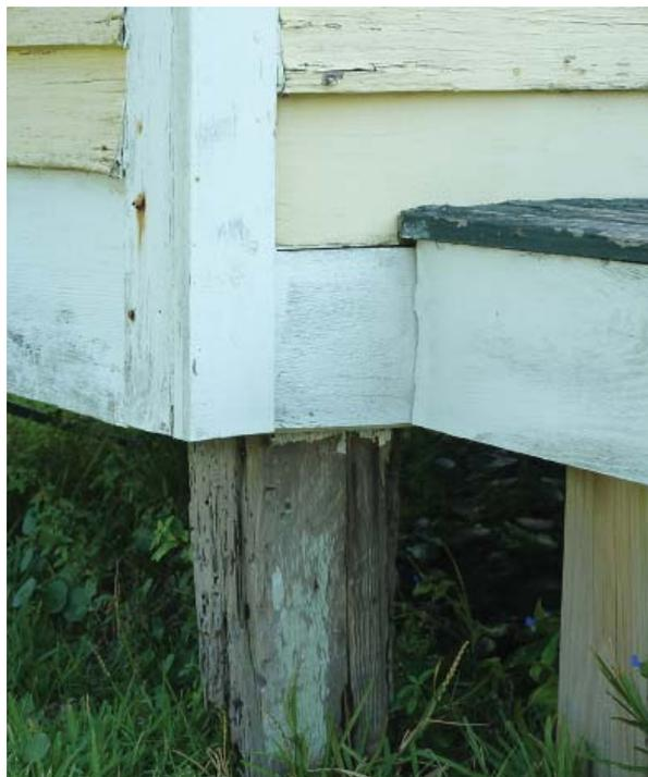
**Figure 83.** Typical vertical corner boards and the two widths of skirt board found on the house.
