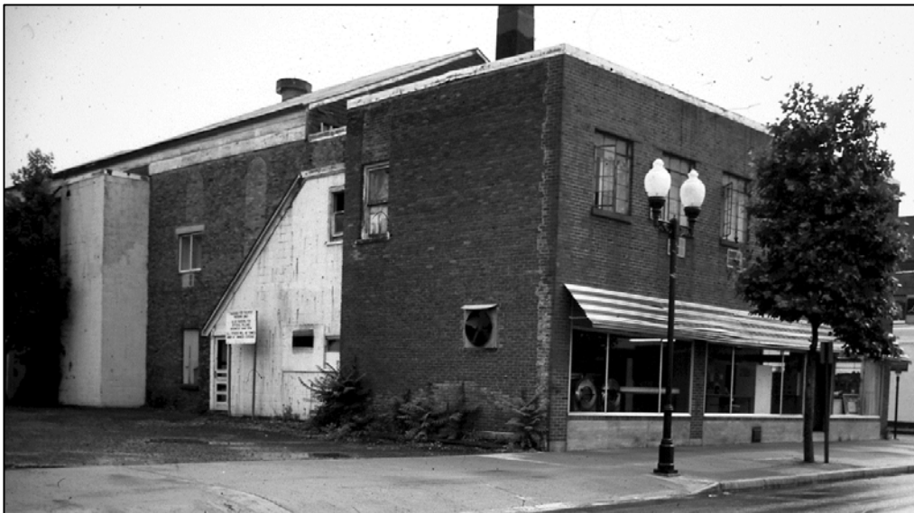
Figure 24. Seneca Falls Laundromat/Wesleyan Chapel from the southwest corner as it appeared when the NPS acquired the property. The gable roof delineates the section of the structure containing the remnants of the Wesleyan Chapel. Courtesy Women's Rights NHP.
