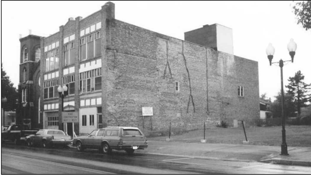
Figure 22. Seneca Falls Village Hall, c. 1991, after the Strand Theater, located to the rear of the adjacent lot, was demolished. Courtesy Women's Rights NHP.
