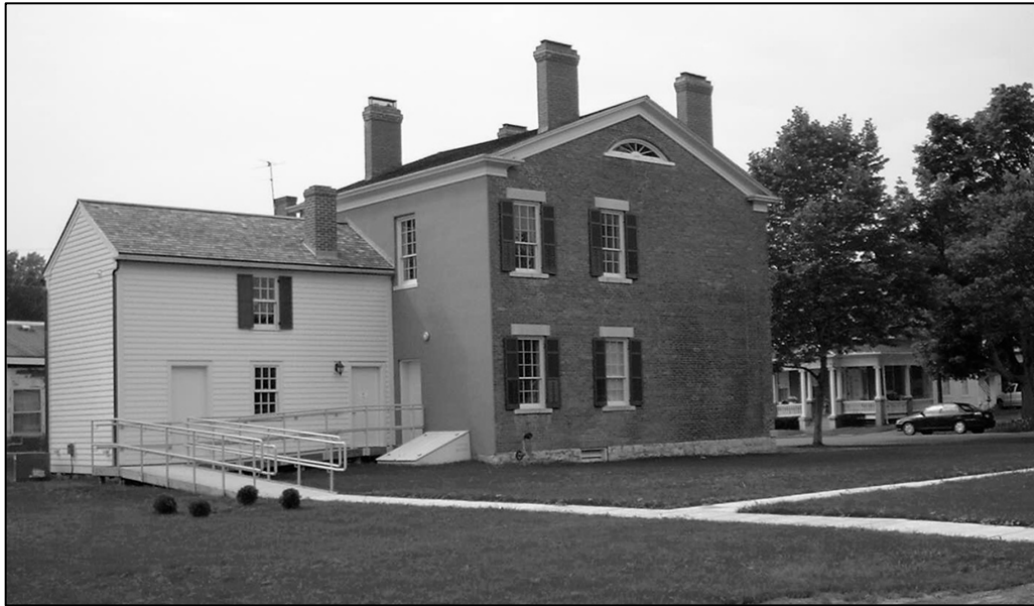
Figure 52. M'Clintock House with reconstructed south wing, 2004. Courtesy Women's Rights NHP.
