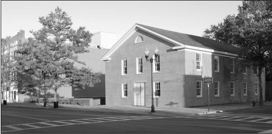
Figure 57. The Wesleyan Chapel Site, front façade and east side. Park Visitor Center in the left background. October 2010. Photograph by Rebecca Conard.
