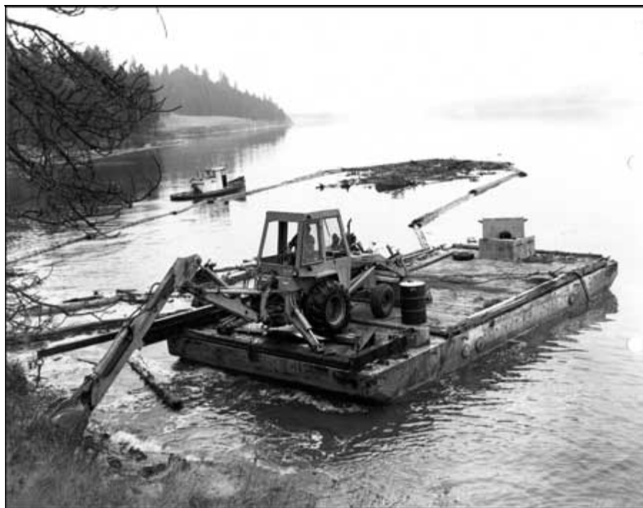
Barge with backhoe and extension boom removing beached debris, and small tug pulling sweep boom, 1976. Photo courtesy of National Park Service, Lake Roosevelt National Recreation Area (file D3217 [old 1023] Report for Cleanup of 1967 Flood Debris, box 3 of 3, LARO #95, Cat. #3250, LARO.HQ.PAO).
