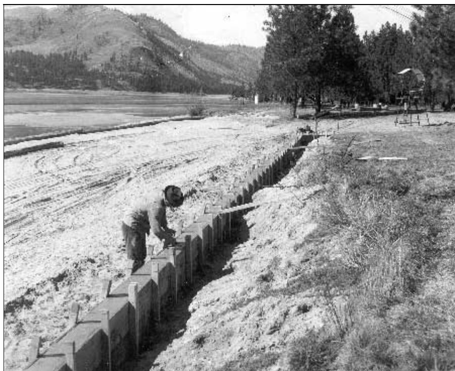
Building a concrete retaining wall at Evans Beach, early 1960s. Gabions and metal-sheet piling have also been used to reduce erosion at developed sites. Photo courtesy of National Park Service, Lake Roosevelt National Recreation Area (LARO.HQ.MENG).
