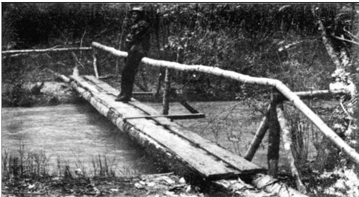
(top) The Sheep Camp Shelter was constructed by Alaska Youth and Adult Authority honor camp inmates in 1963. It served as a camping spot and day use area until 1993, when NPS personnel completed the laying out of a new campground, half a mile south of the shelter. (bottom) Footbridge typical of the Dyea end of the trail, 1968. (Mark Bollinger photo, KLGO SC #1627 (top); Alaska DNR, "The Chilkoot Trail, Trail of '98," 5)
