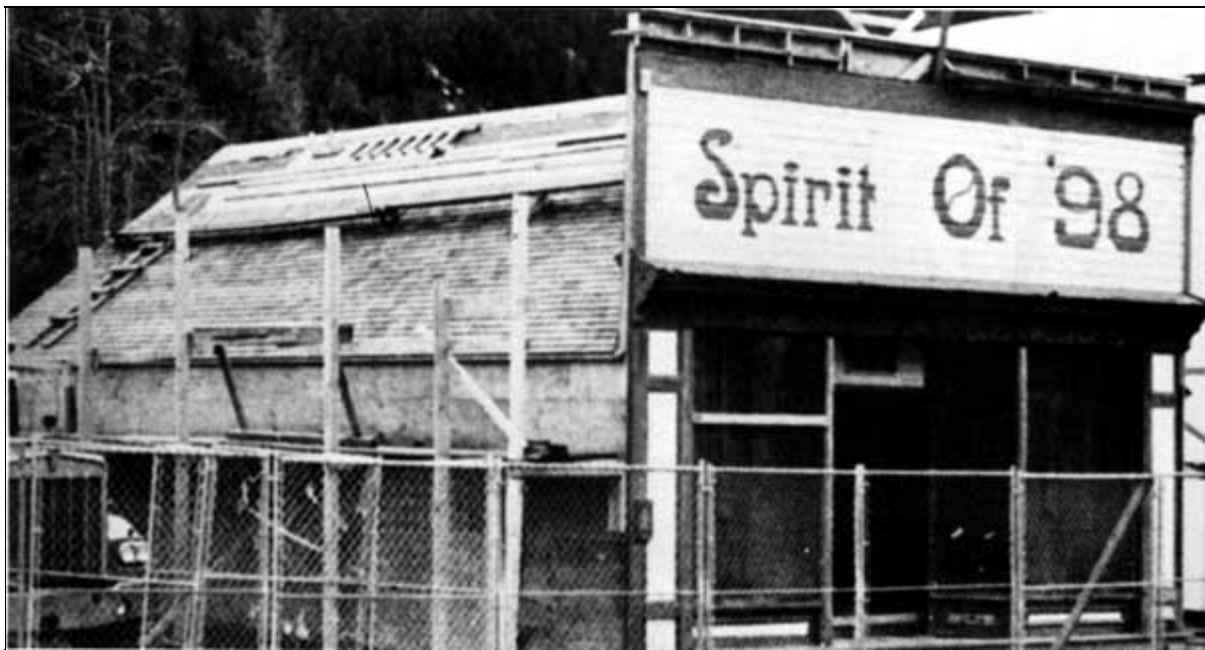
(top) The Arctic Brotherhood Hall served as the park's visitor center from 1979 through 1983. This photo, looking north, shows Skagway Garden Club member Marcia Healy watering the flower boxes along the boardwalk. (bottom) The NPS construction crew began to rehabilitate the Boss Bakery building in the summer of 1985. It completed its work in 1986, and the building was leased in 1987. ( Jeff Brady Collection (both photos) )
