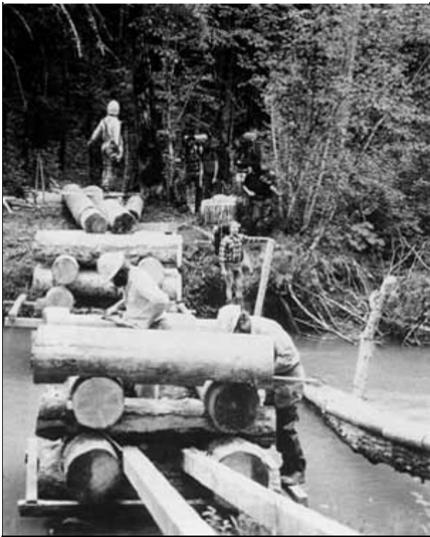
(left) During the 1960s and 1970s, historical artifacts such as horseshoes were more numerous than they are today. (right) NPS crews have been maintaining the Chilkoot Trail since 1979. In 1982, one of the crew's largest tasks was the construction of a log bridge at 6-1/2 mile, between Finnegan's Point and Canyon City. (W. E. Garrett photo, in National Geographic Magazine , June 1965, 801 (left); David Cohen photo, KLGO SC #1931 (right))
