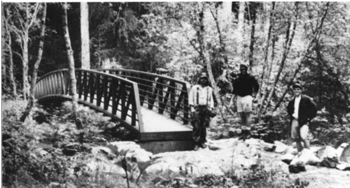
(top) At Mile 11 of the Chilkoot Trail, periodic floods had destroyed several wooden bridges. To solve the problem, NPS personnel decided to erect a suspension bridge at the site. The photo was taken in 1982, the year the bridge was completed. (bottom) In 1991, the Chilkoot Trail maintenance crew completed a 90-foot long steel truss bridge at 1-1/2 mile, one of several major trail improvements. Bridge workers (l-r) included Roy Nelson, Jerry Watson, and Mike Beierly. ( David Cohen photo, KLGO SC #2042 (top); John Warder Collection (bottom) )
