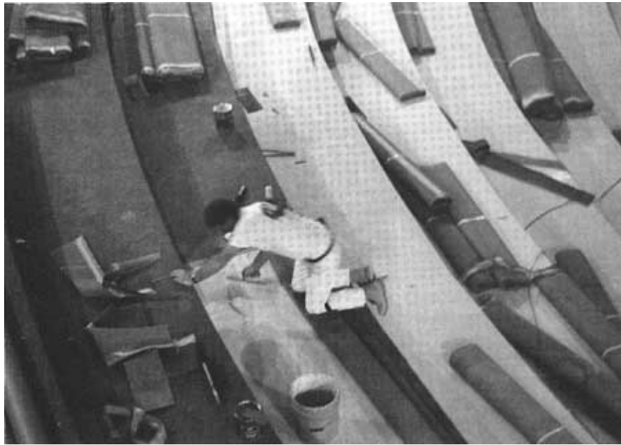
Carpeting the tiered seating area, 1992. NPS photo, courtesy Dave Caselli.
