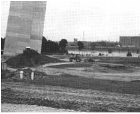
Earth removal, August 21, 1990.
