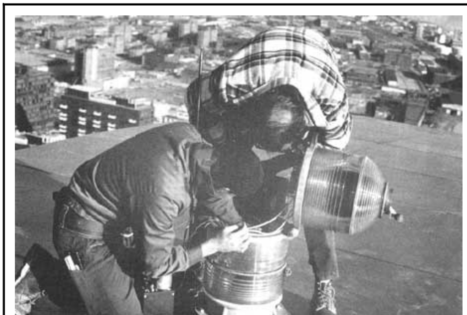
ATS Crew Foreman Harry Breitenstein replaces the aircraft warning light on the top of the Arch, October 1976. NPS photo by Norman Messinger.
