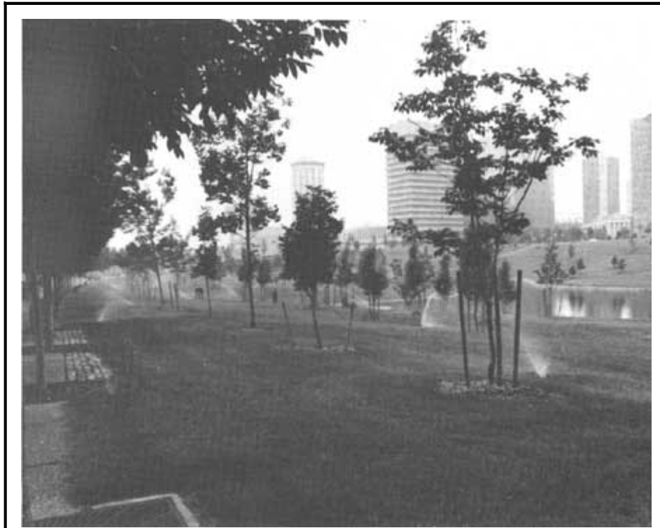
The irrigation system with sprinkler heads functioning. Photo courtesy John Weddle.
