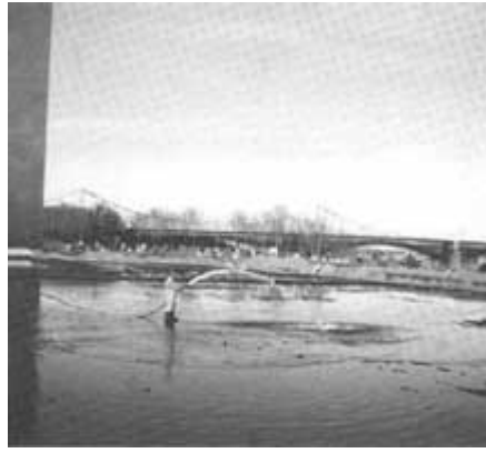
Testing for water-tight qualities, November 26, 1990.
