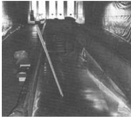
Asbestos removal, January 9, 1991.
