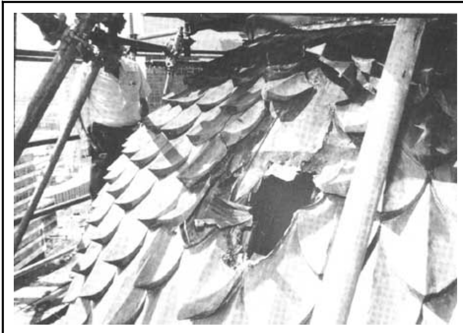
Fire investigation, June 1979, showing the hole chopped in the roof of the lantern and the exterior scaffolding. NPS photo by Norman Messinger.
