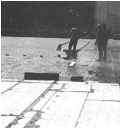
Installation of Pave-Prep, November 2, 1990.
