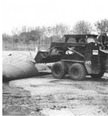
Removal of old waterproofing material, November 7, 1990.
