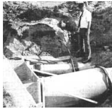
Dave Caselli examines exposed pipe, October 5, 1990.
