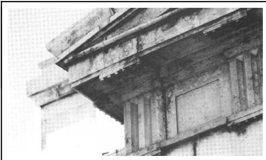
Deteriorated cornice, Old Courthouse, 1978. *NPS photo.*
