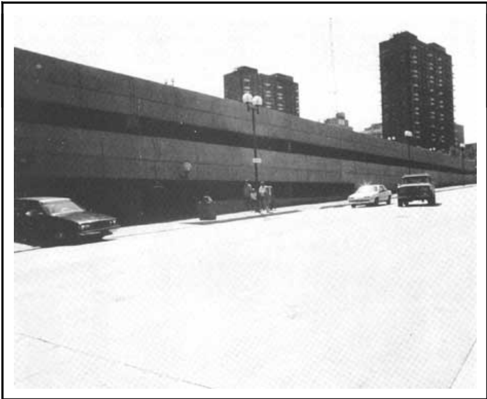
The completed Gateway Arch Parking Garage, from Washington Street on the north side of the Arch grounds, April 1987. NPS photo.
