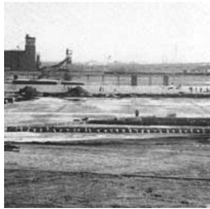
New installation of waterproofing material, February 2, 1991.
