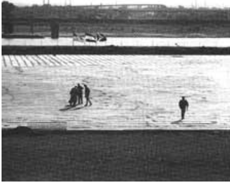
The exposed visitor center roof, October 24, 1990.
