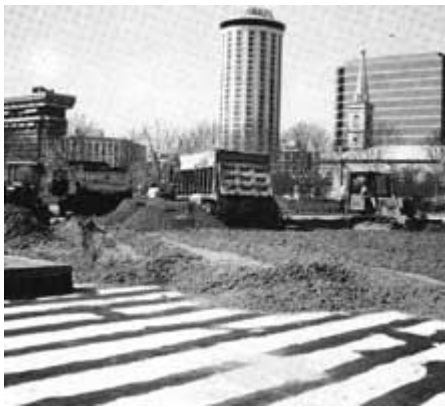
Replacing soil, visitor center roof, April 1, 1991.
