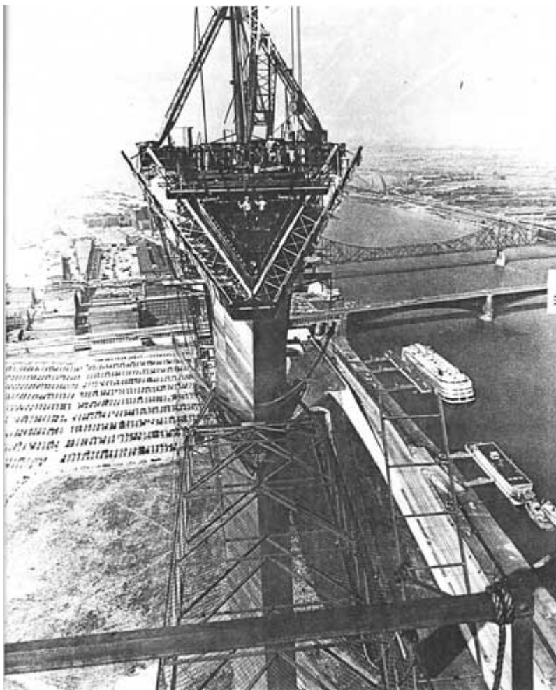
The Arch's triangular sections are composed of stainless and plate steel, concrete and steel tendons.
