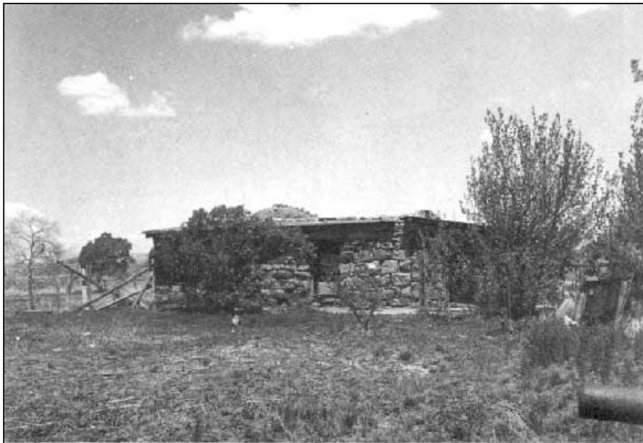
Figure 26. Stone Residence (Bunkhouse), HB-5, in about 1965. This structure, located in the southwest corner of the compound, is used today only for storage. It could possibly be rehabilitated as another residence, or as quarters for visiting NPS employees. NPS photo, HUTR Neg. 117.
