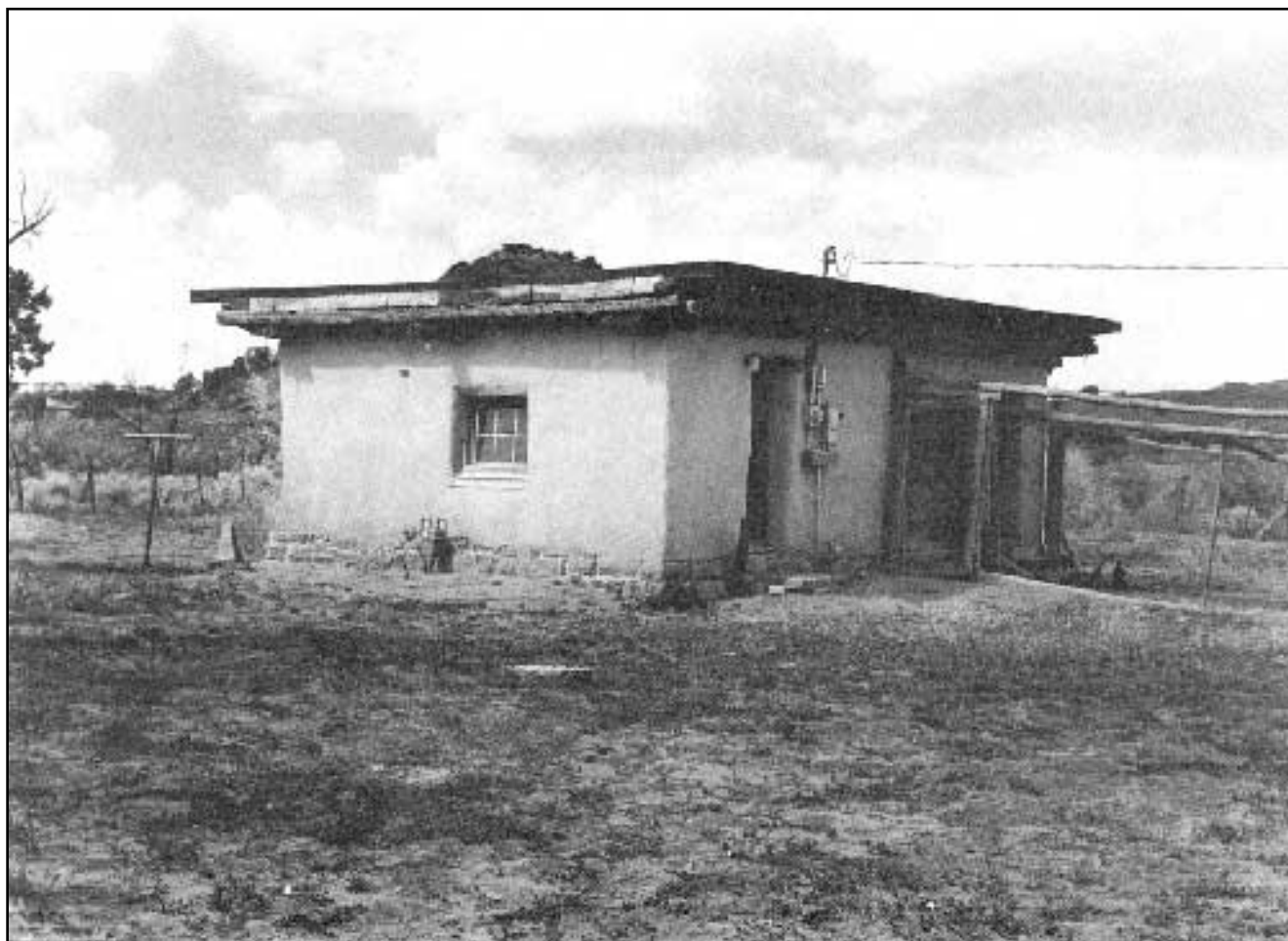
Figure 31. The Adobe Utility Building, HB-8, the chicken coop, as it looked in October, 1991, with a few resident chickens. A Manchester photo.
