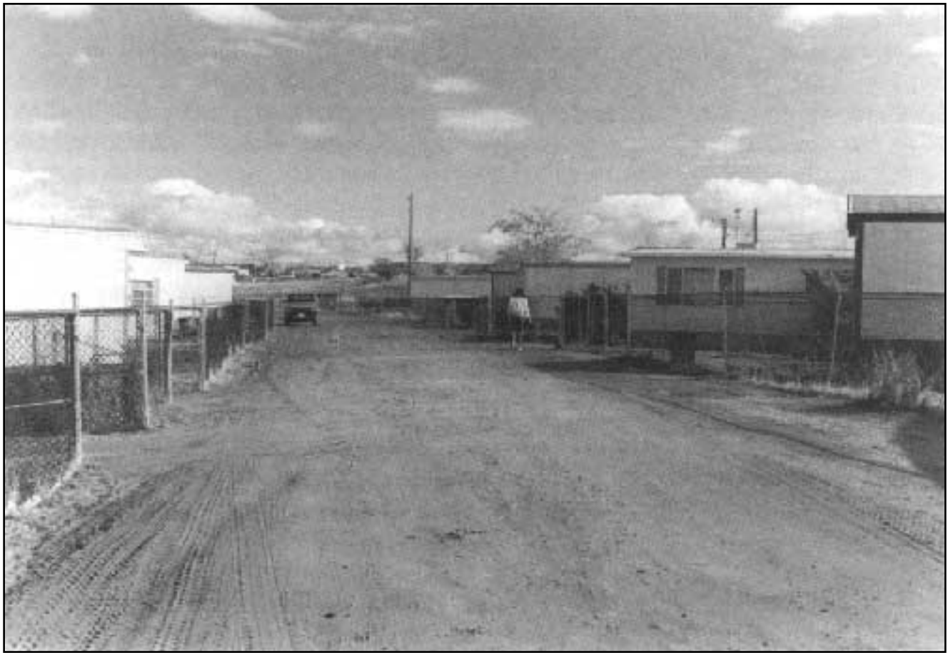
Figure 48. Employee housing at Hubbell Trading Post NHS. NPS photo by E. Bauer. HUTR Neg. R73#24.
