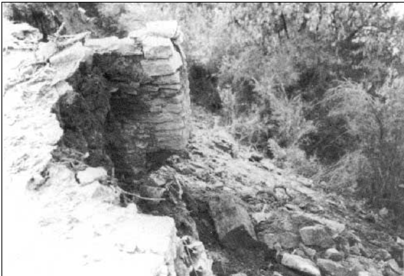
Figure 40. A corner of Wide Reed Ruin in December of 1971. This photograph illustrates some of the damage done to the site by erosion along Pueblo Colorado Wash. NPS photo by E. Bauer. HUTR Neg. R76#23.
