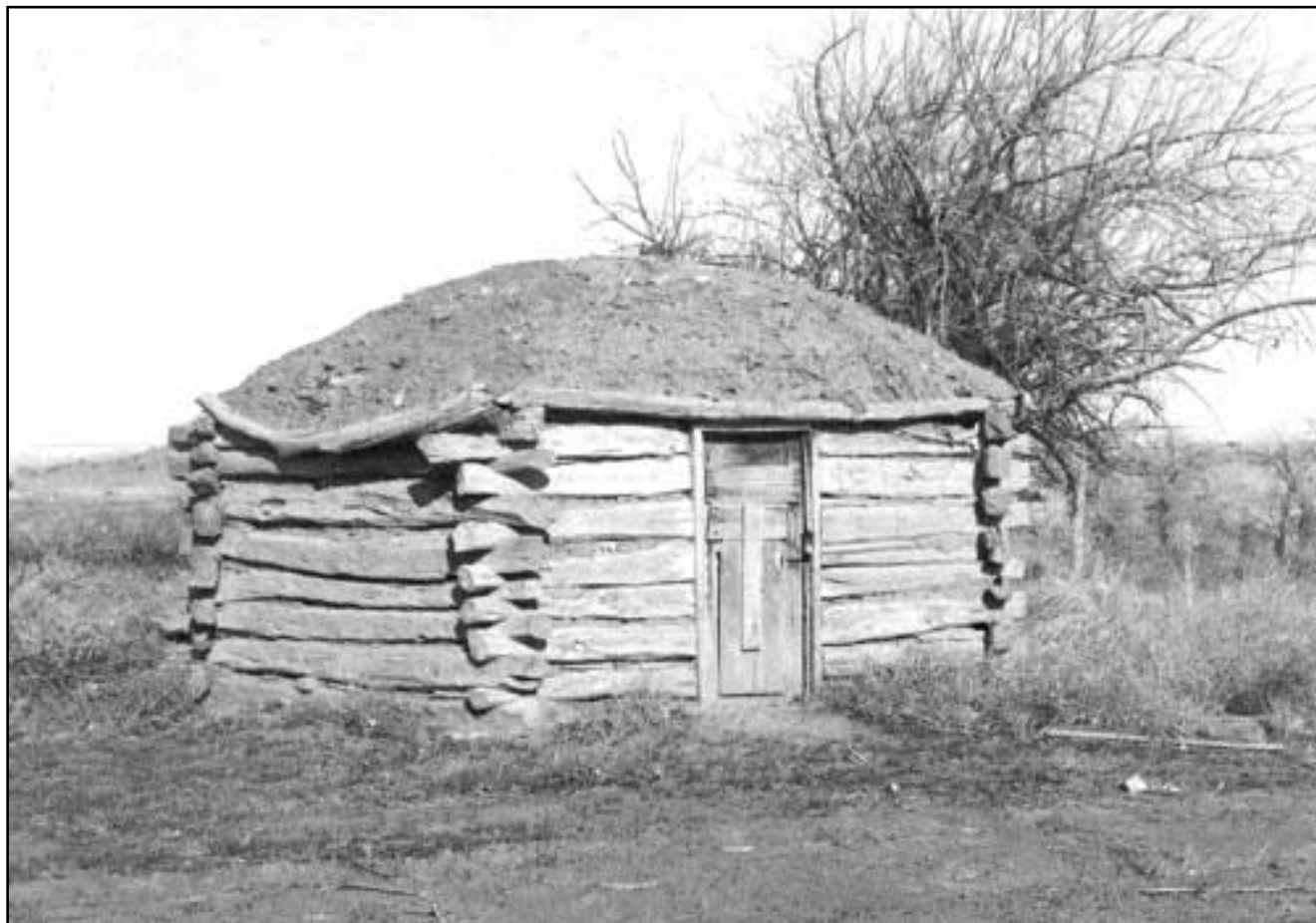
Figure 33. The Hogan-in-the-Lane, HB-11, was probably built in the 1950s by Friday Kinlicheenie for his personal quarters. There were other hogans at the trading post, apparently all north of the main buildings. NPS photo, April, 1966, HUTR Neg. 171.
