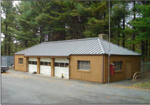
FIGURE 9. MAINTENANCE FACILITY, THE BLUFFS
