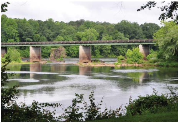
FIGURE 42. View from tour stop overlook of modern Highway 49 bridge and Miller Bridge piers (background). NPS photo.
