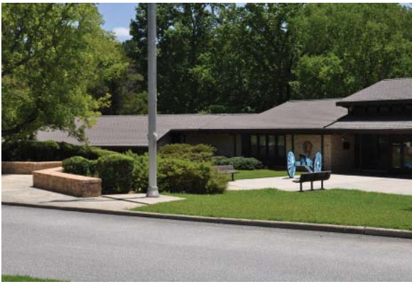
FIGURE 31. Entrance Area. NPS photo.
