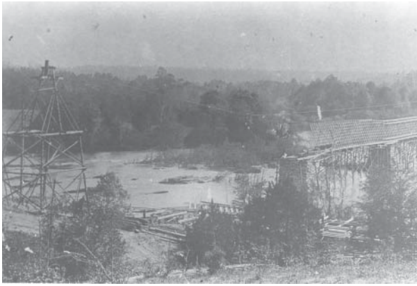
FIGURE 20. Construction of Miller covered bridge, c.1907. HOBE Archives.
