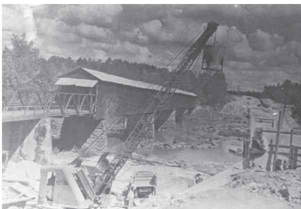
FIGURE 21. Construction of Highway 99 bridge next to Miller covered bridge, c. 1955. HOBE Archives.
