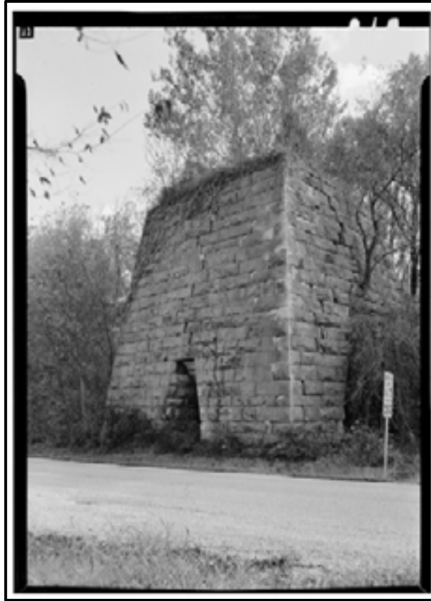
Figure 2.4. Bear Spring Furnace, located in Stewart County, similar to Great Western Furnace, Library of Congress.
