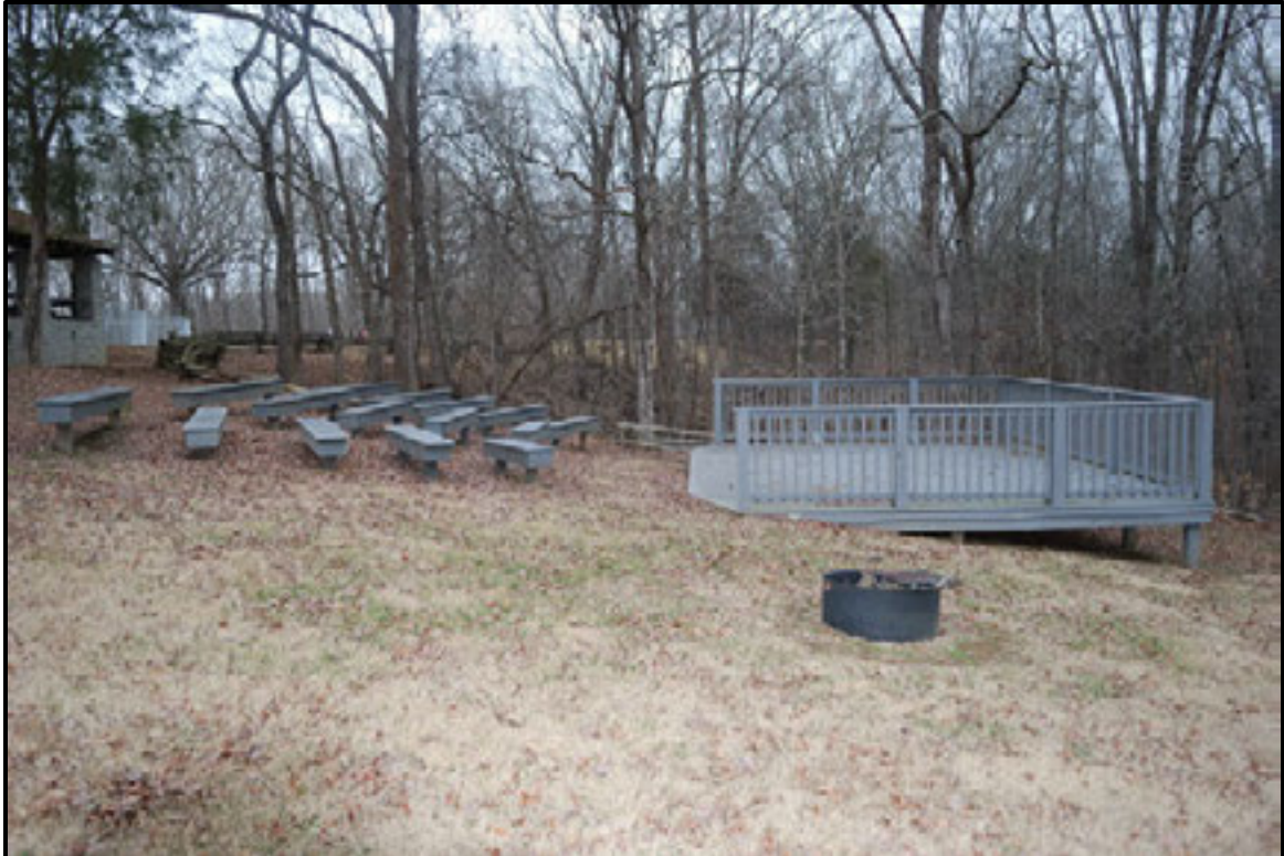
Figure 7.126. View of amphitheater.
