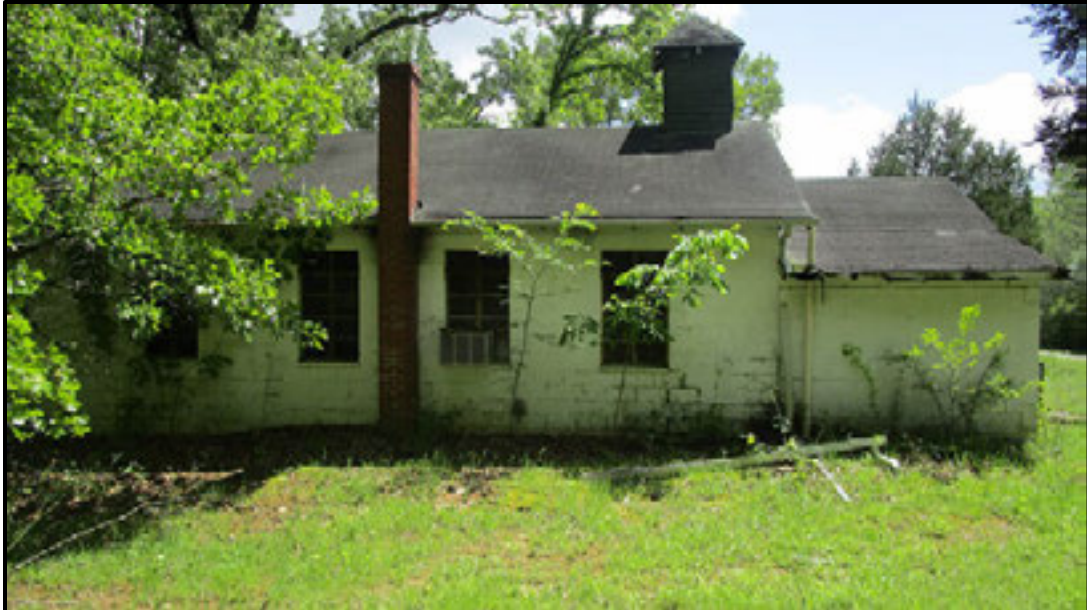
Figure 7.153. St. Paul United Methodist Church, north elevation.
