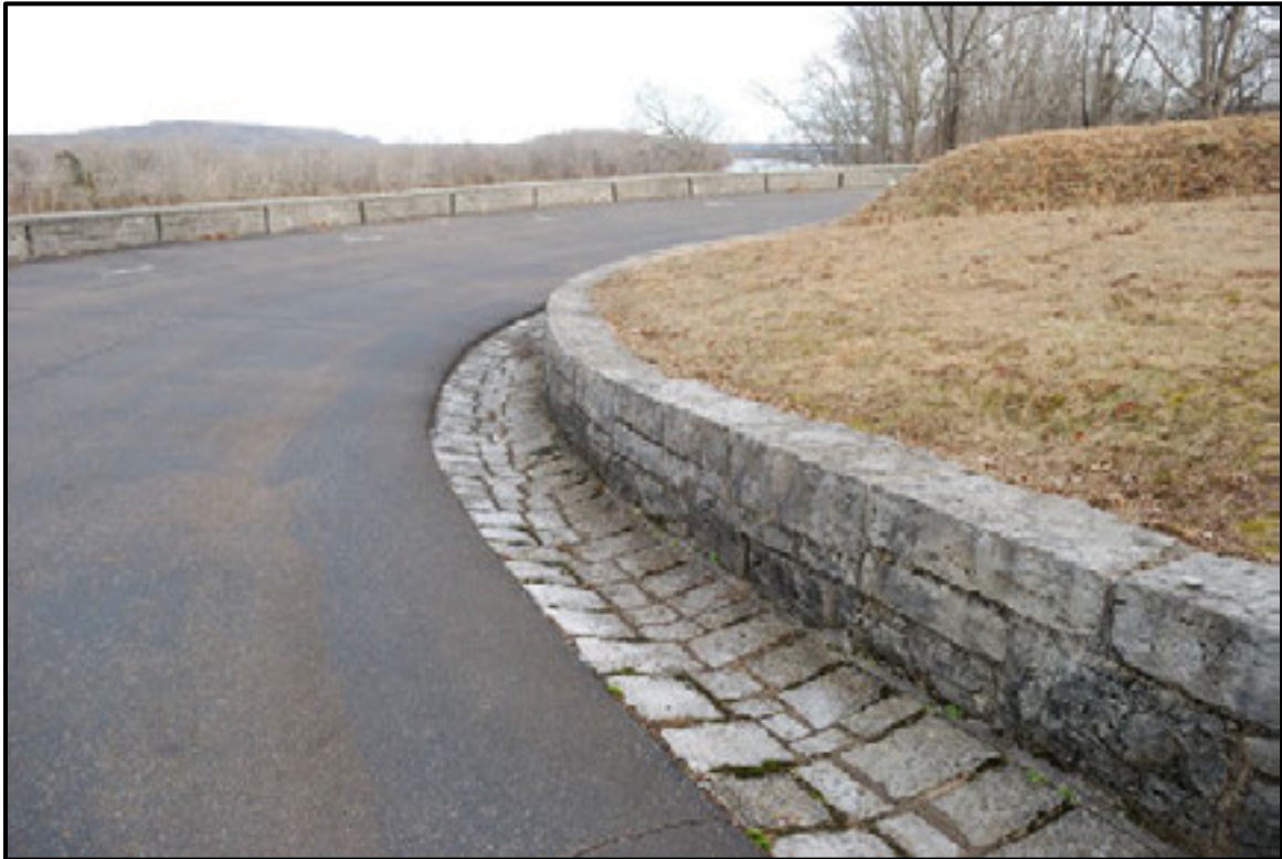
Figure 7.119. View of stone swale and retaining wall at Upper River Battery.
