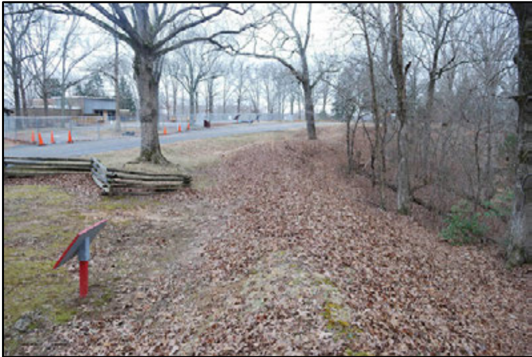
Figure 7.24. Segment 12 near the visitor center; this portion of the berm is more eroded and lower.
