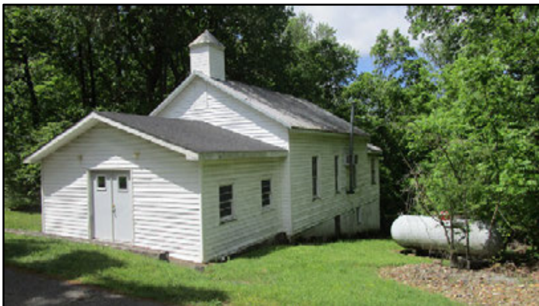
Figure 7.157. East Oak Grove Baptist Church, south and east elevations.
