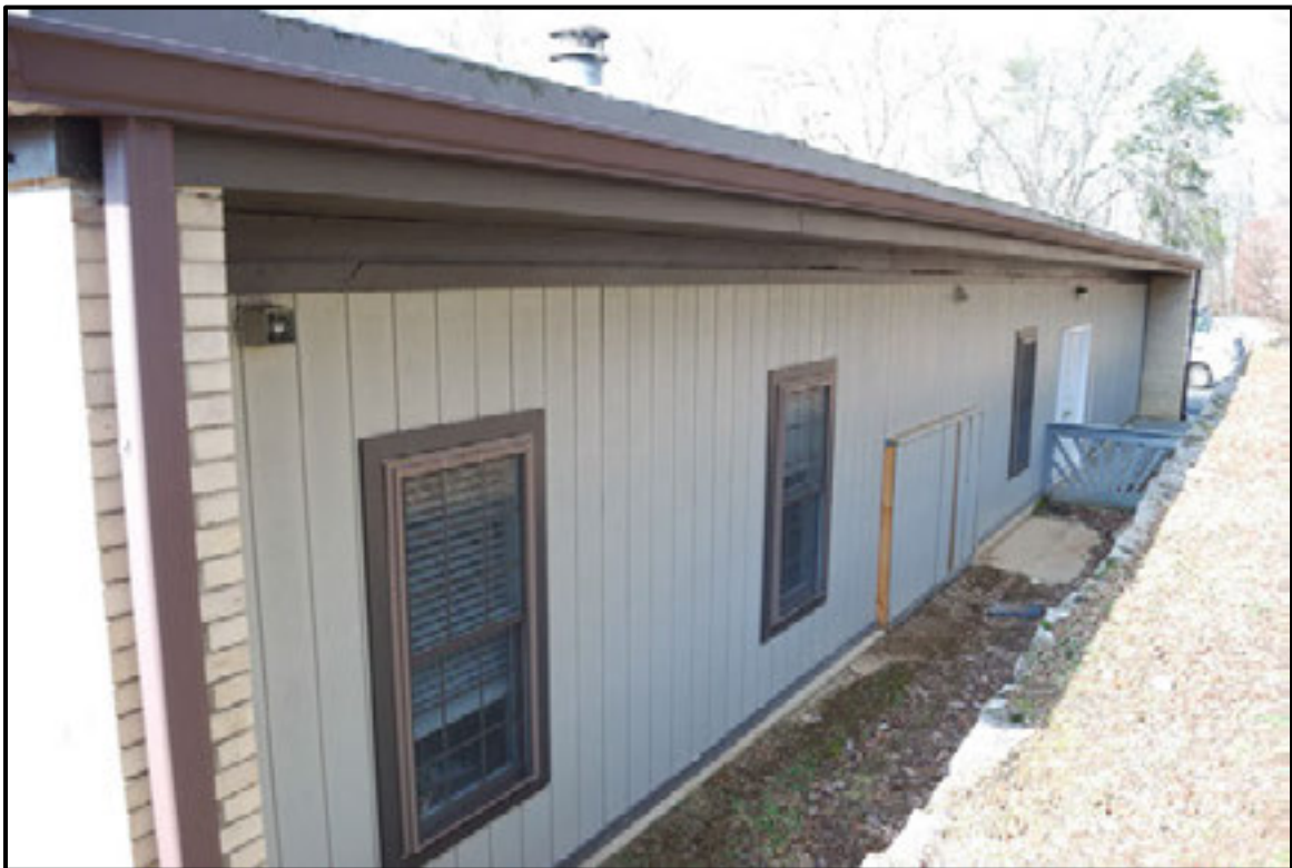
Figure 7.93. Rear (northeast) elevation of ranger station.
