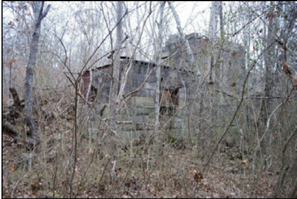
Figure 7.145. View of outbuilding (Resource G).
