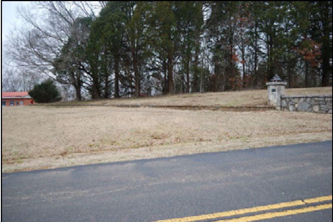
Figure 7.98. View of secondary retaining wall.
