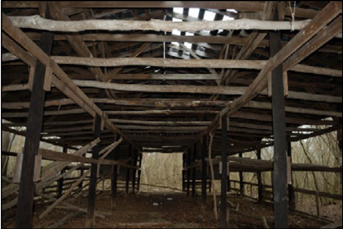
Figure 7.136. Interior view of barn (Resource B).
