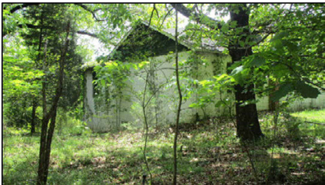
Figure 7.155. St. Paul United Methodist Church, rear (east elevation).
