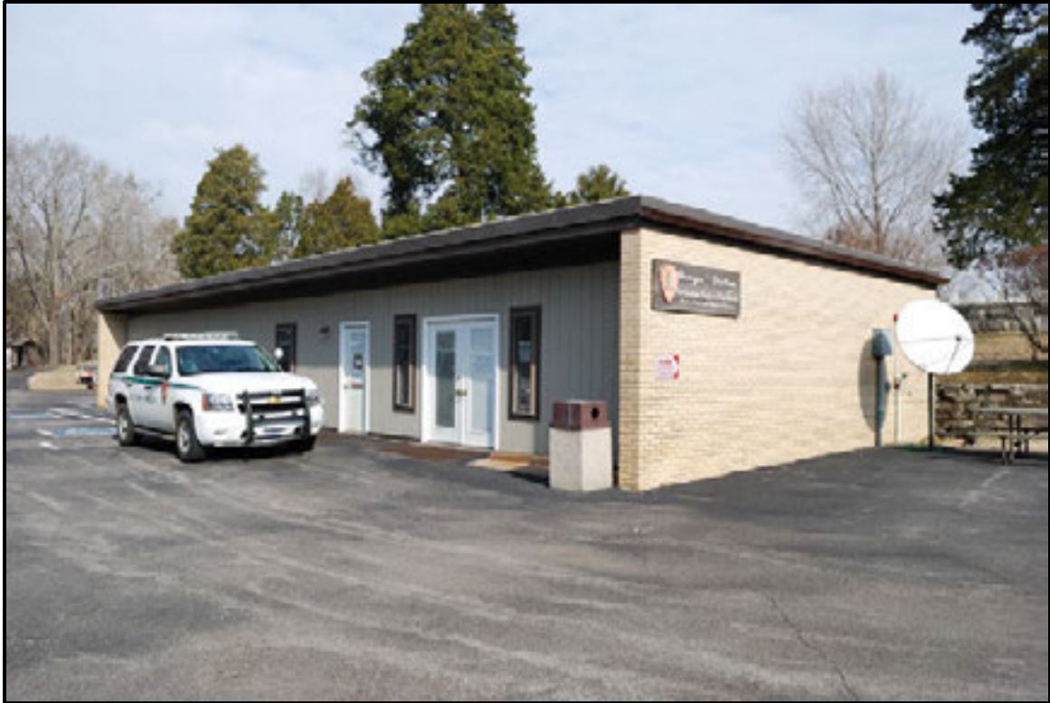
Figure 7.92. Façade (southwest) and southeast elevations of ranger station.
