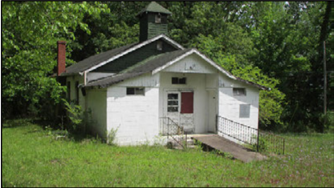
Figure 7.152. St. Paul United Methodist Church, façade (west elevation).
