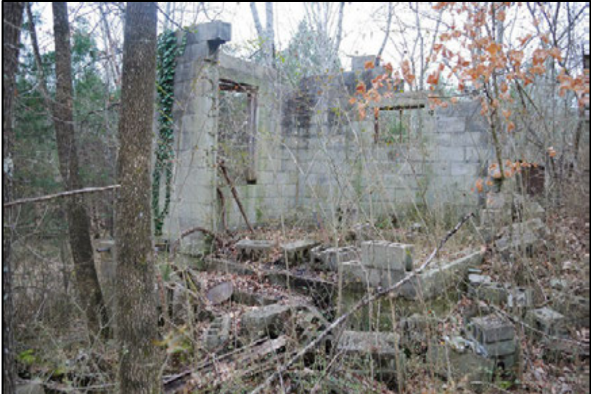
Figure 7.144. View of outbuilding (Resource G).
