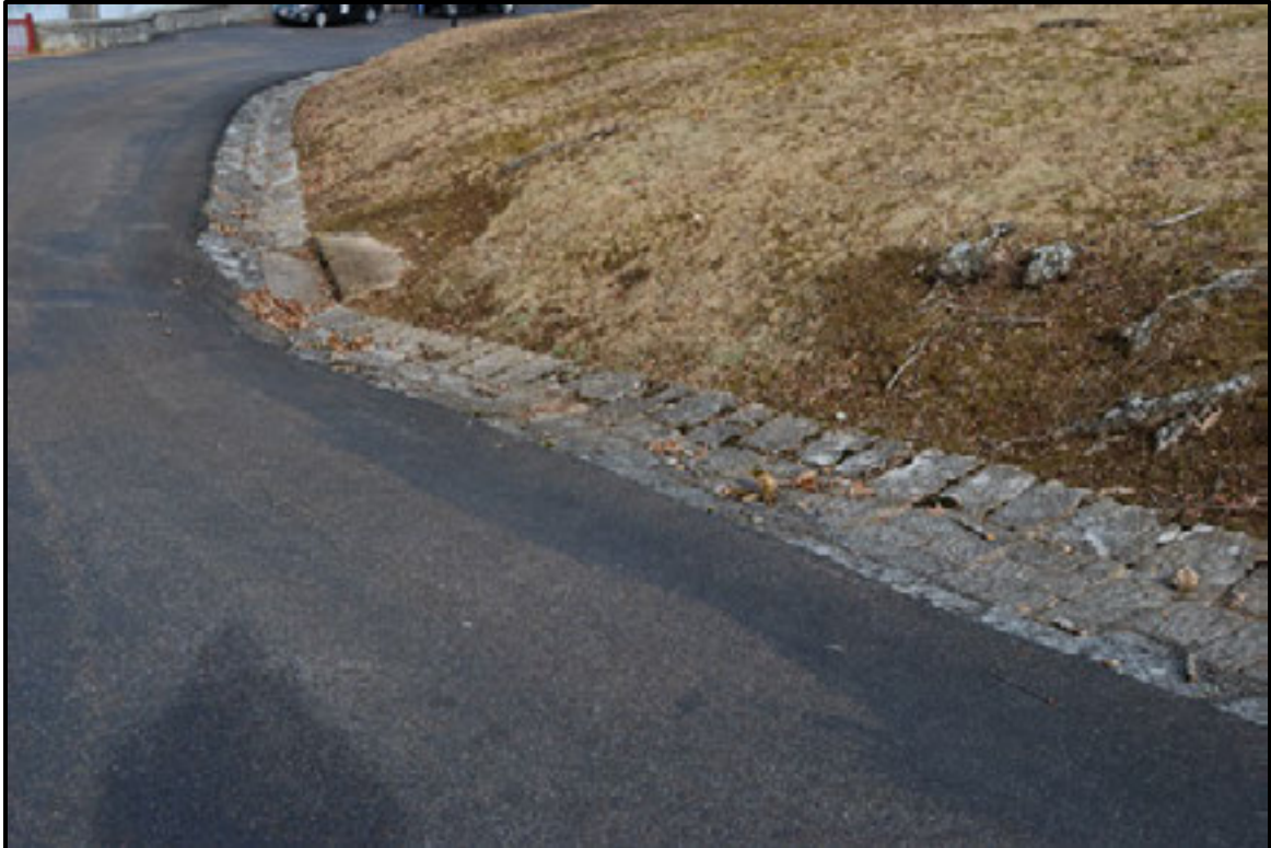
Figure 7.107. View of swale near upper water batteries.
