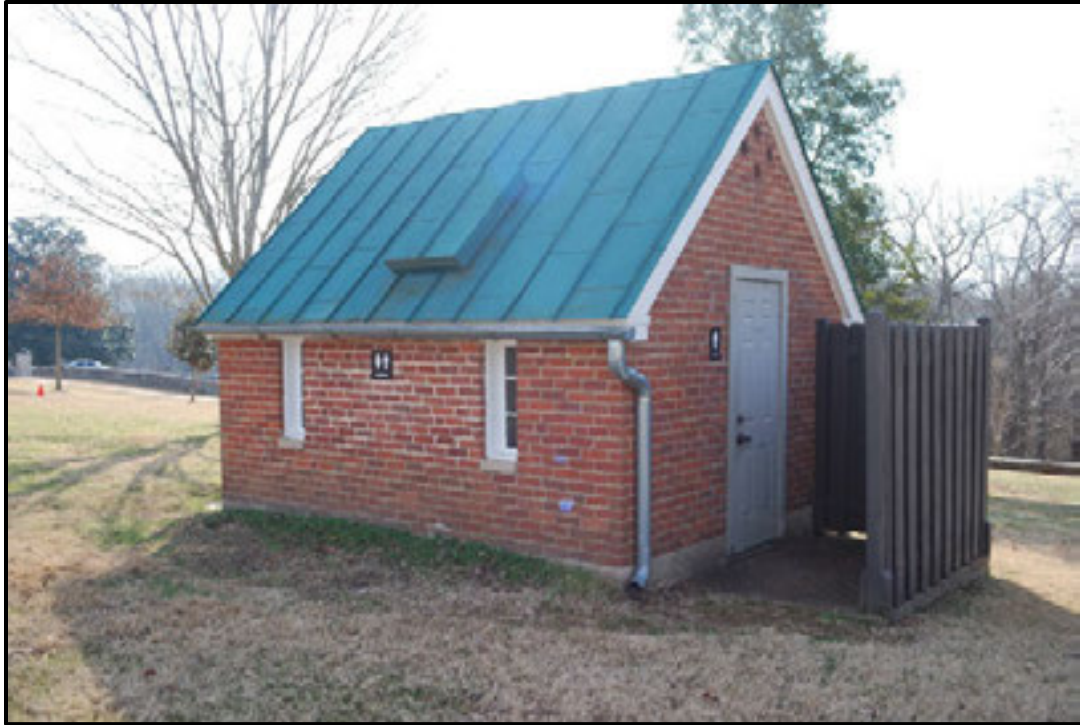
Figure 7.71. Pump House, north and west elevations.
