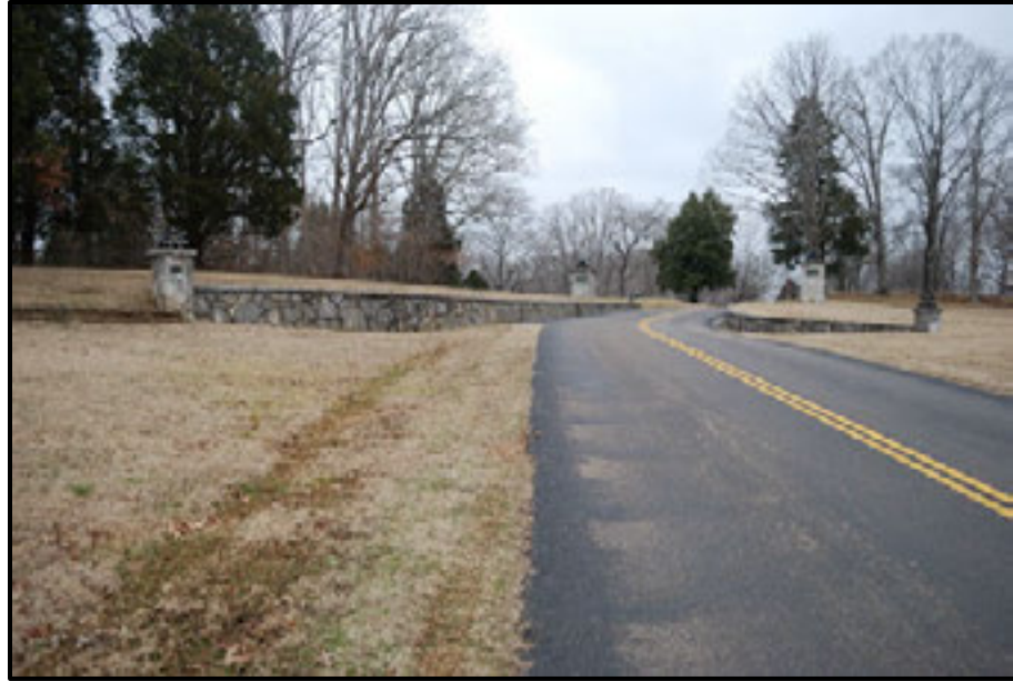
Figure 7.95. Overview of main park entrance.
