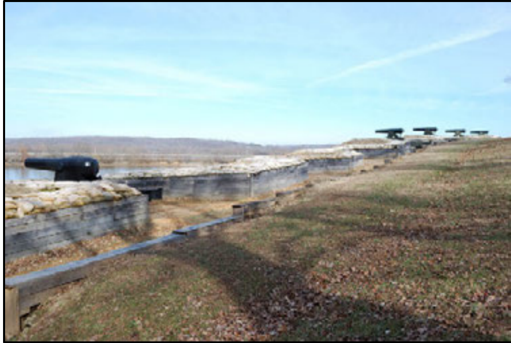
Figure 7.9. Lower River Battery showing ditch behind the retaining wall created by runoff.
