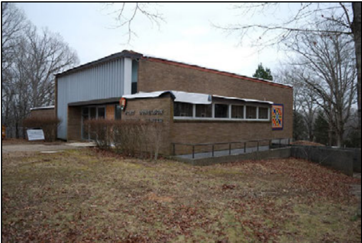
Figure 7.124. Façade and southwest elevation of Visitor Center.
