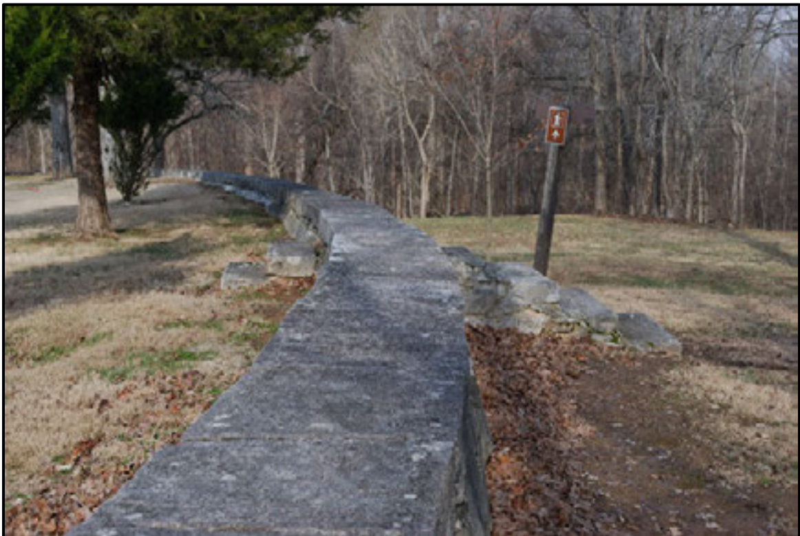
Figure 7.84. View of stile along cemetery wall.
