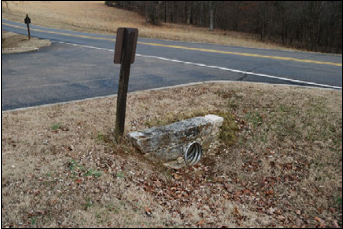
Figure 7.106. View of culvert near intersection of Fort Donelson Park Road and Eddyville Loop Road.
