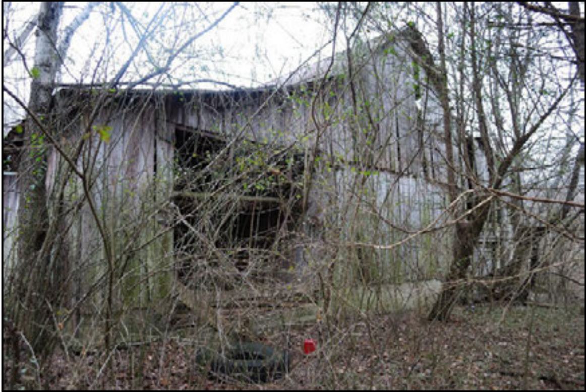
Figure 7.141. Southwest elevation of barn (Resource F).
