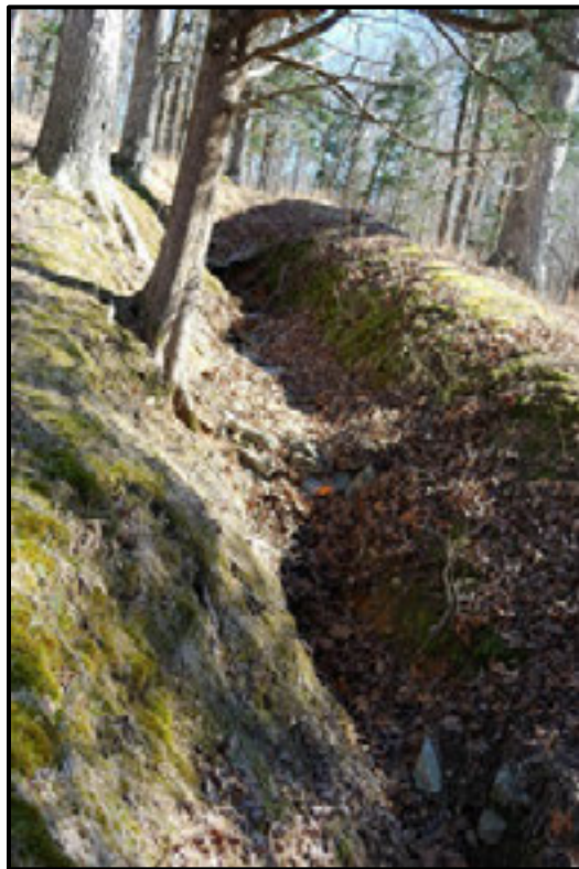
Figure 7.30. Segment 15, water damage in the ditch and rocks placed to slow runoff.
