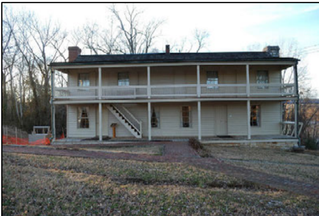
Figure 7.42. Dover Hotel, east elevation.
