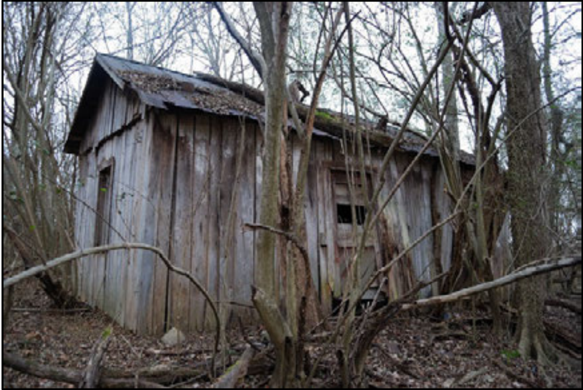
Figure 7.133. West and rear elevation of residence (Resource A).
