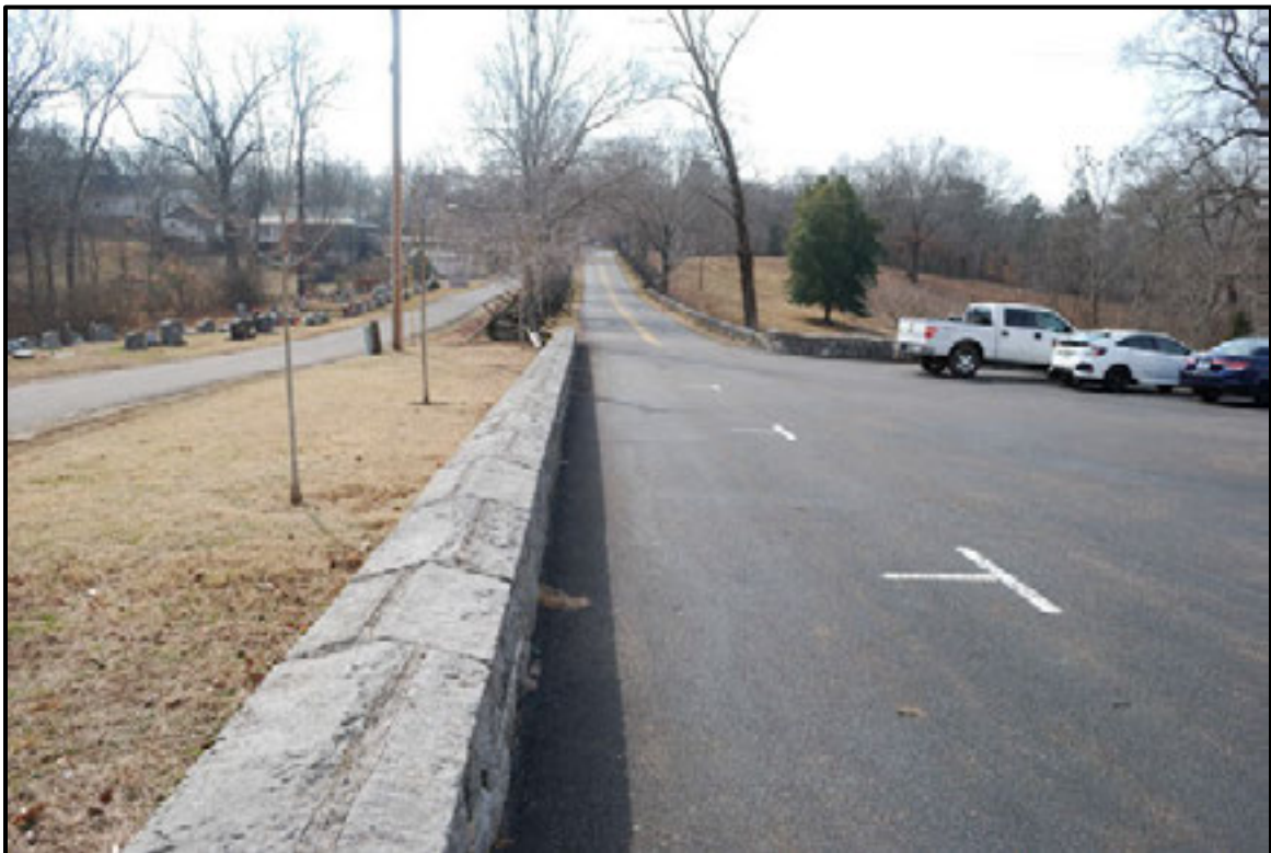
Figure 7.86. Overview of entrance drive from main parking lot.
