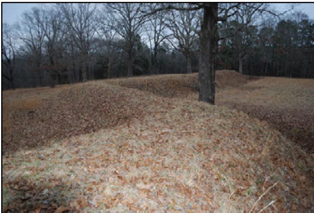
Figure 7.5. Wall of Fort Donelson near Fort Donelson Park Road at the top of the ridge.
