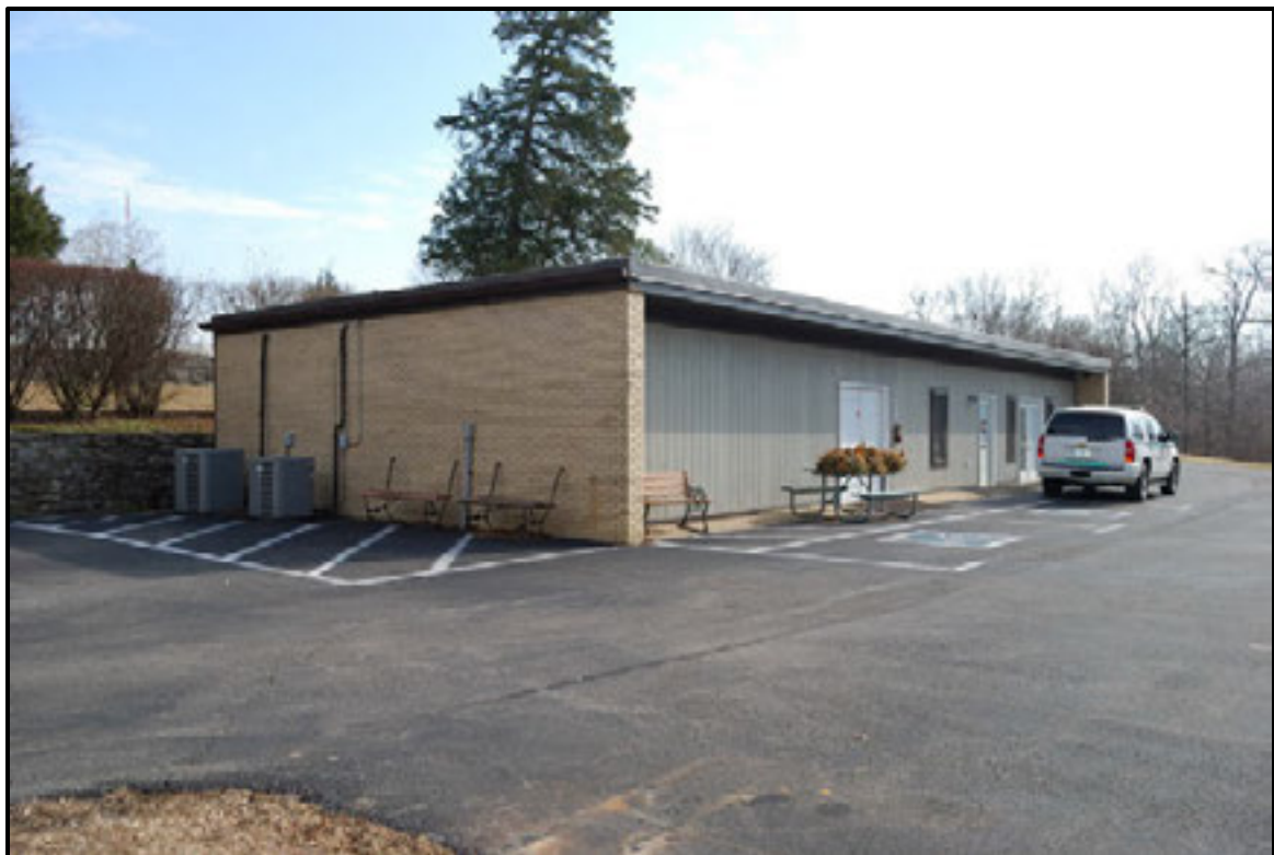
Figure 7.91. northwest and façade elevations of ranger station.
