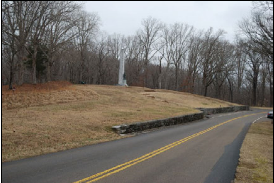
Figure 7.115. Overview of south side of retaining wall.
