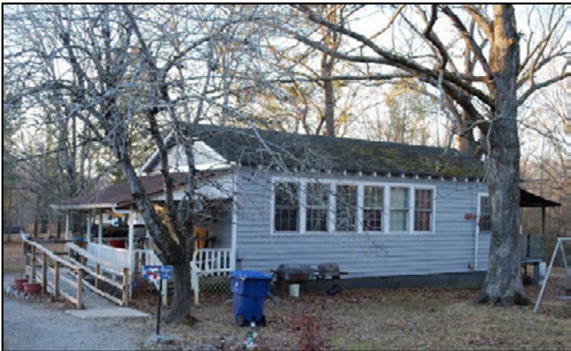
Figure 7.149. Former Dover Colored School, south and east elevations.
