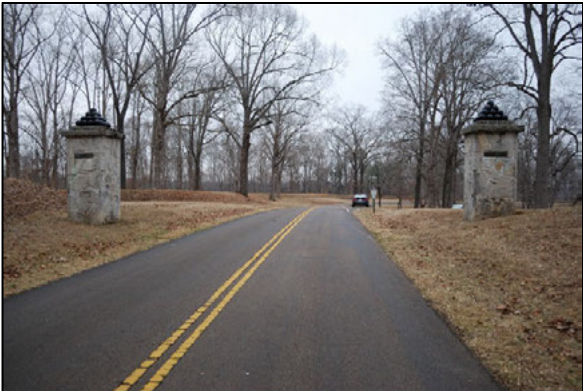
Figure 7.100. Overview of entrance columns.
