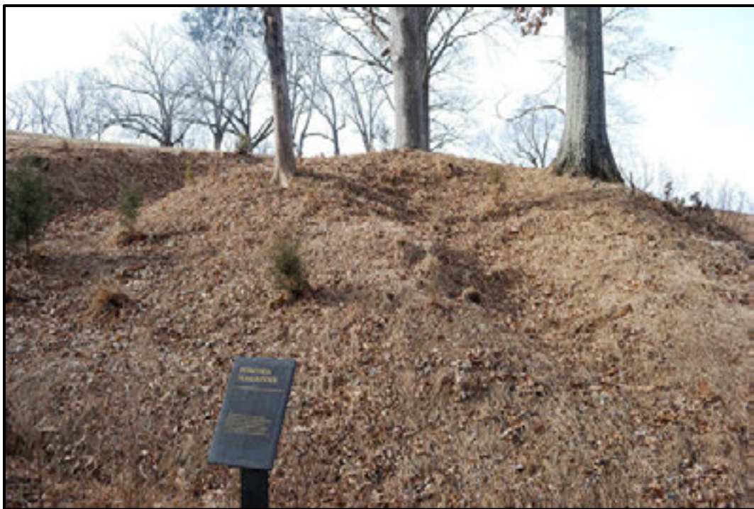
Figure 7.8. The collapsed powder magazine; erosion caused by runoff is clearly visible.
