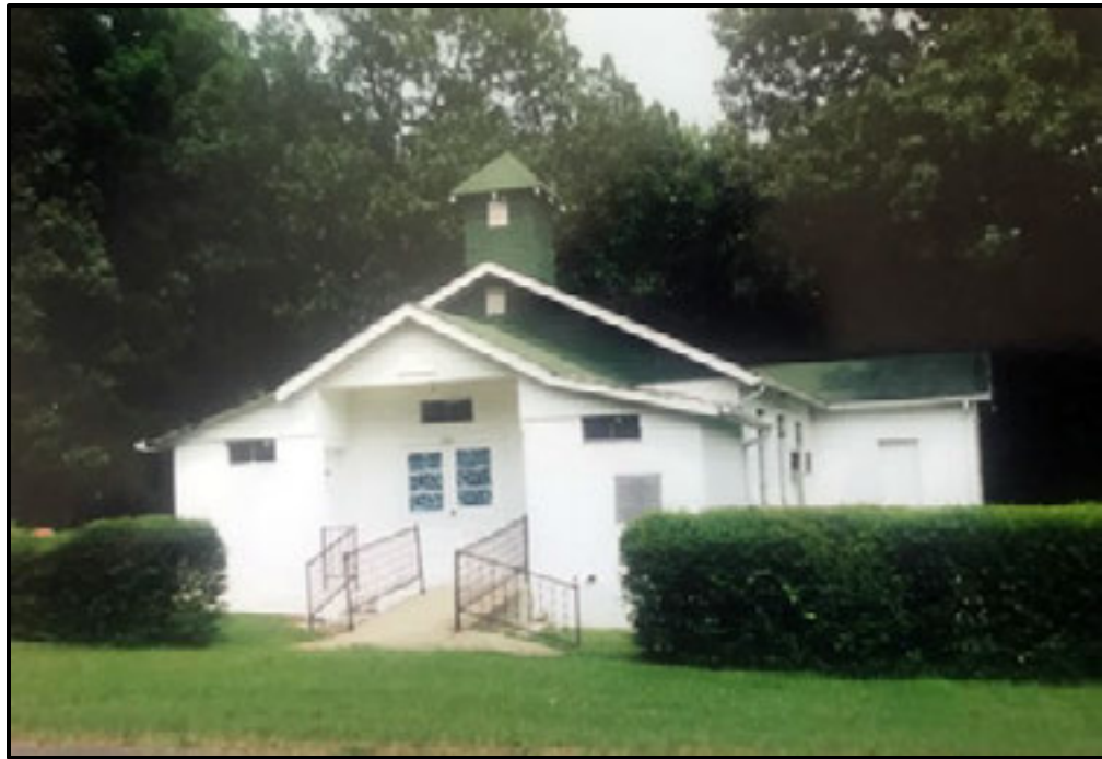
Figure 5.18. St. Paul United Methodist Church, Tennessee Civil War National Heritage Area.
