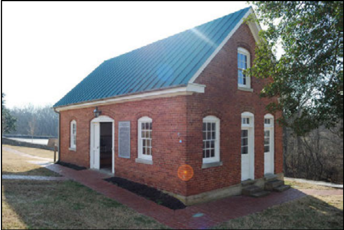
Figure 7.68. Carriage house, façade (north) and west elevations.
