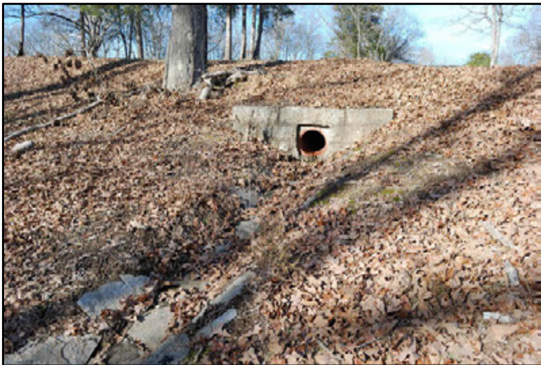
Figure 7.34. Segment 16, drain below parking area at French's Battery.
