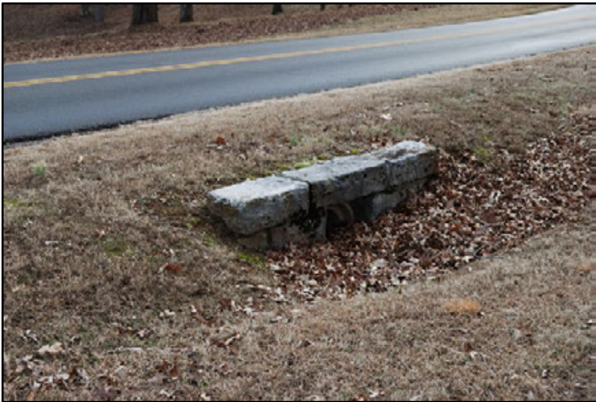
Figure 7.105. View of culvert along Fort Donelson Park Road.
