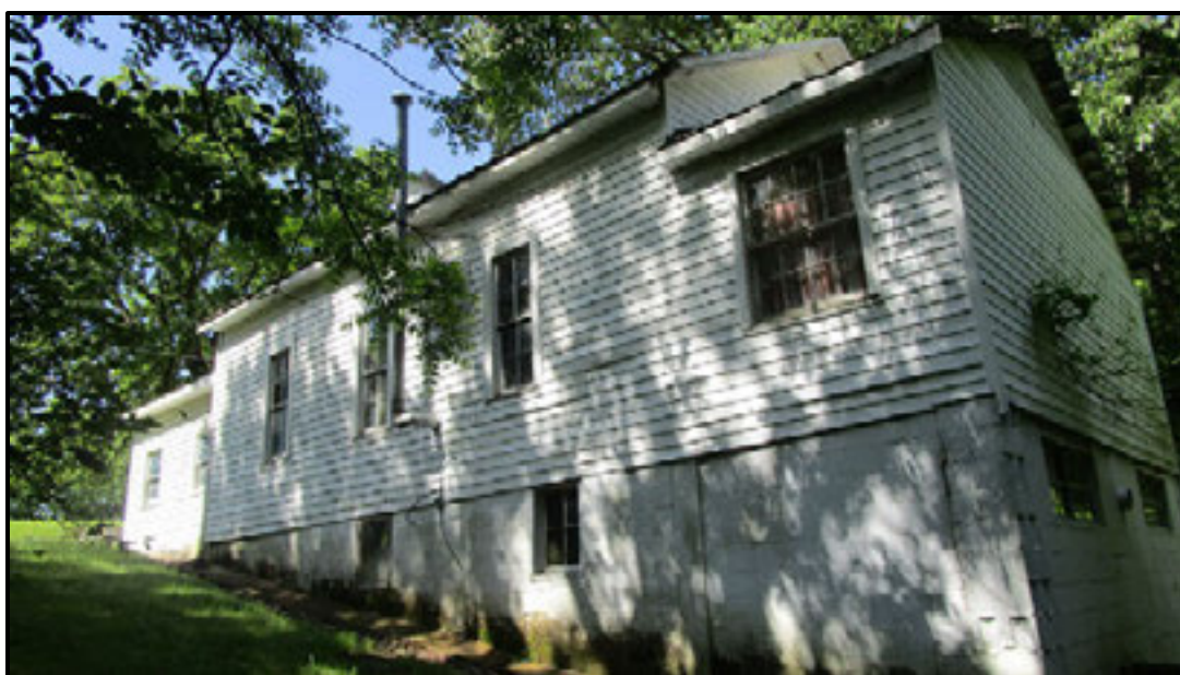
Figure 7.158. East Oak Grove Baptist Church, east and north elevations.
