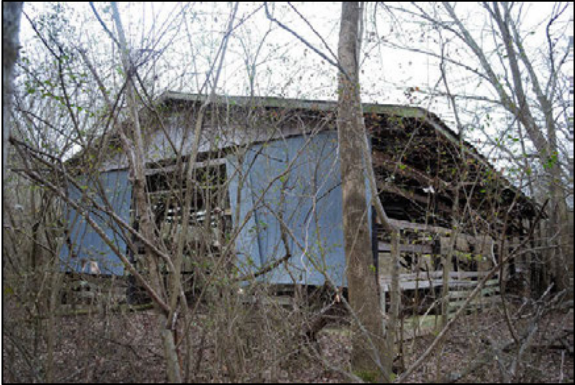
Figure 7.135. South and east elevation of barn (Resource B).
