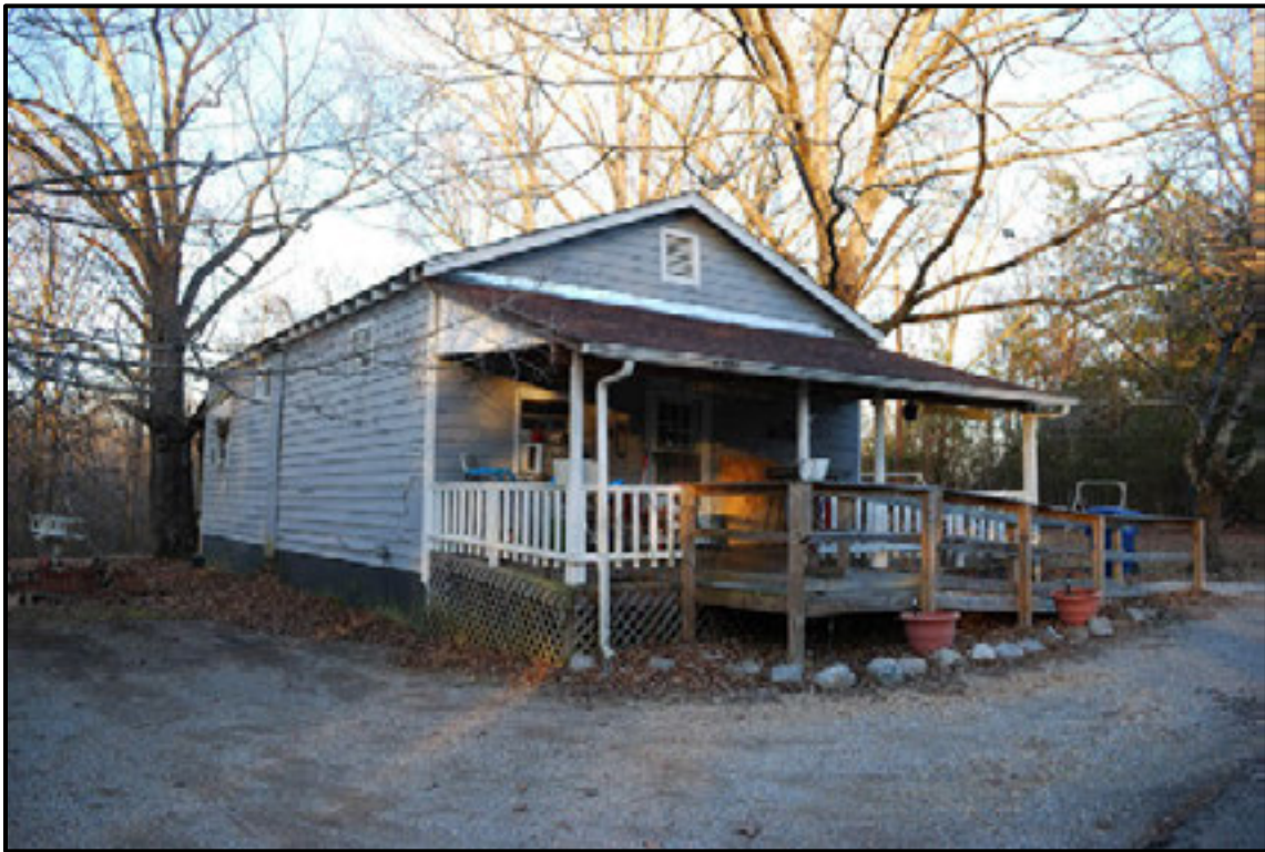
Figure 7.148. Former Dover Colored School, south and west elevations.
