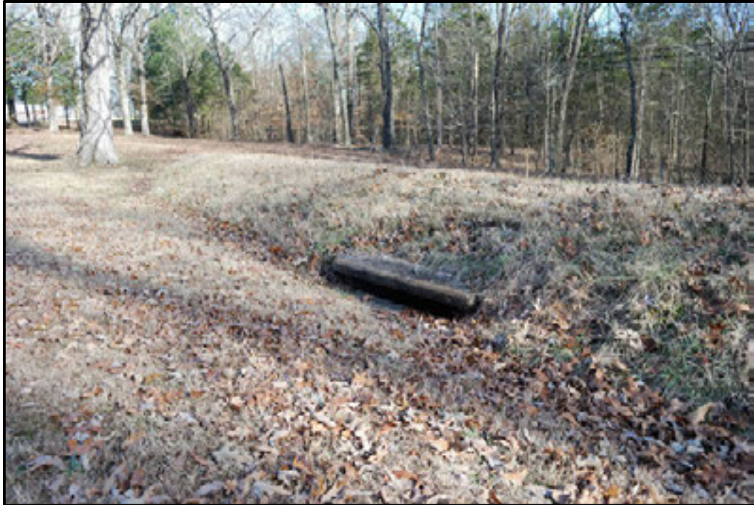
Figure 7.36. Segment 17, concrete culvert installed to aid drainage.
