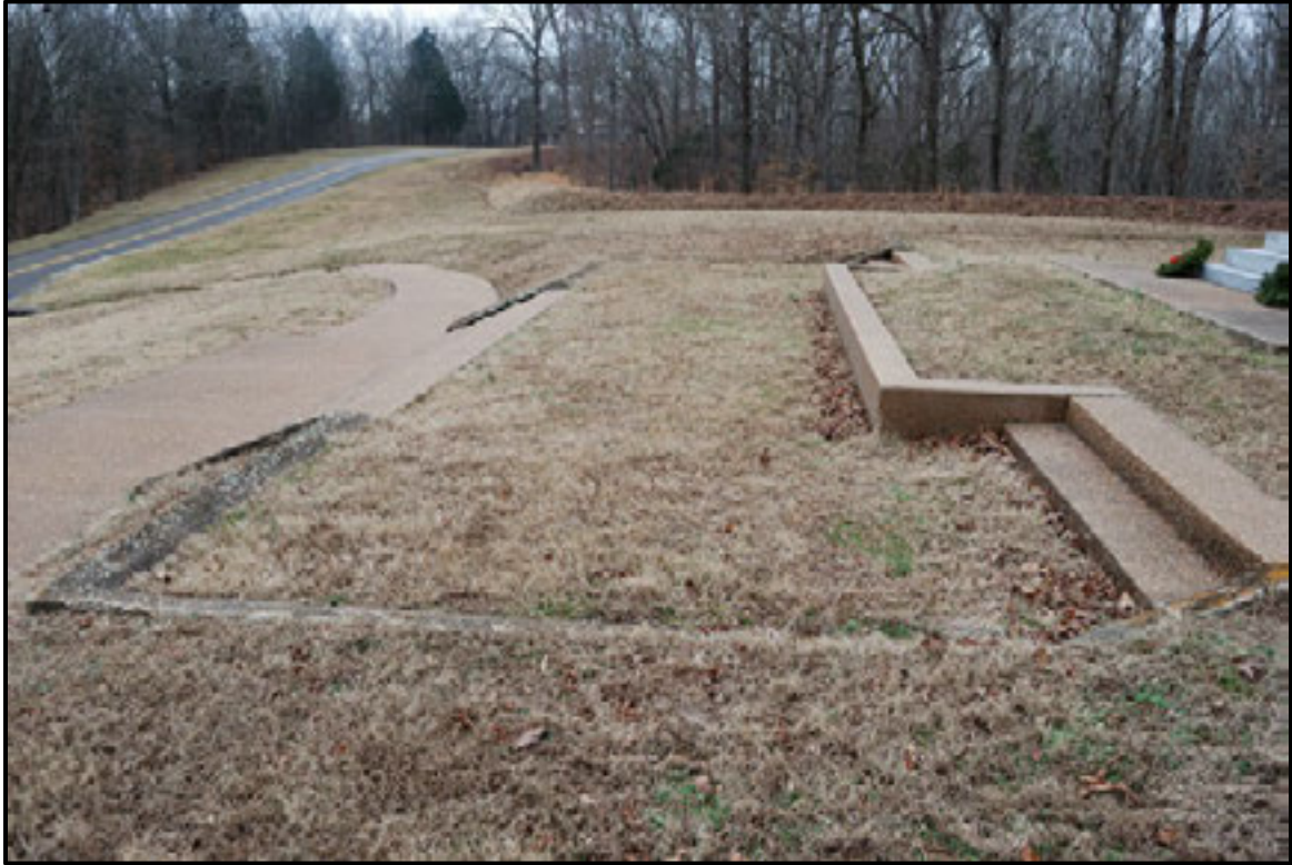
Figure 7.114. View of tiered approach and concrete border.
