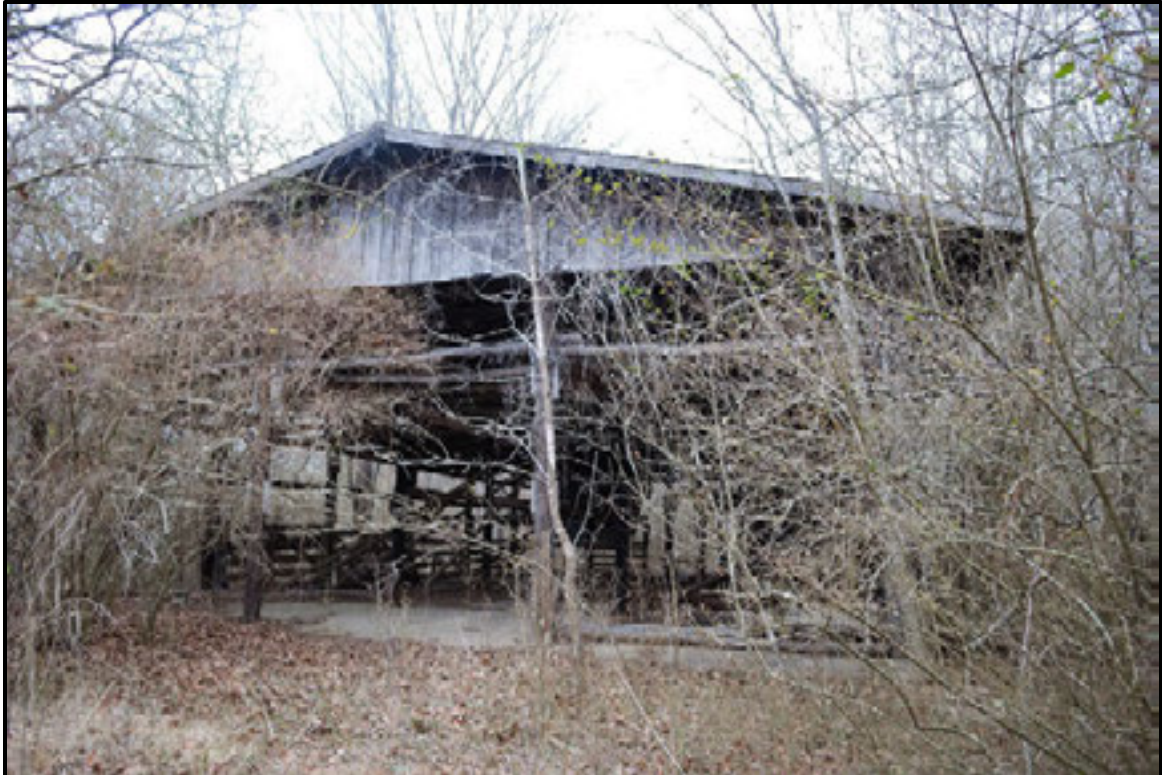
Figure 7.134. North elevation of barn (Resource B).
