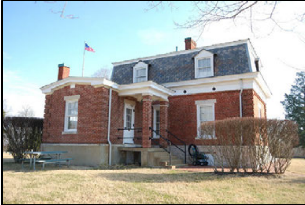
Figure 7.66. Cemetery Lodge, rear (west) elevation.
