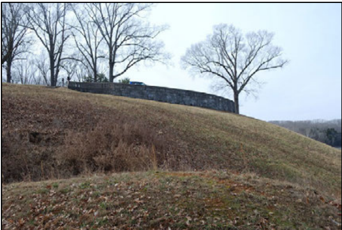
Figure 7.120. Portion of retaining wall facing river constructed below grade.
