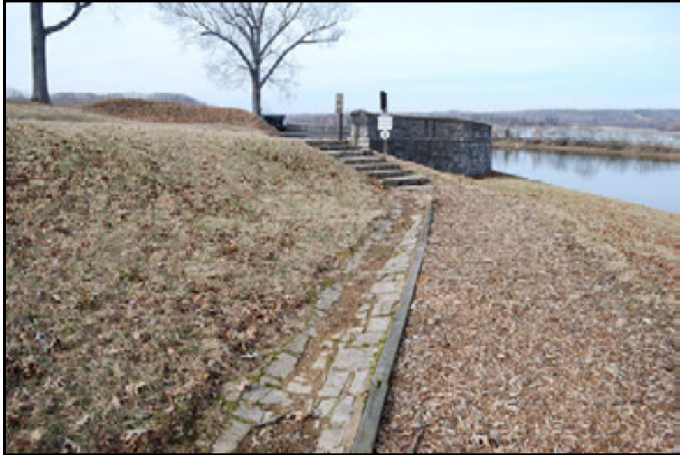
Figure 7.121. View of stone stairs and walkway near Upper River Battery.
