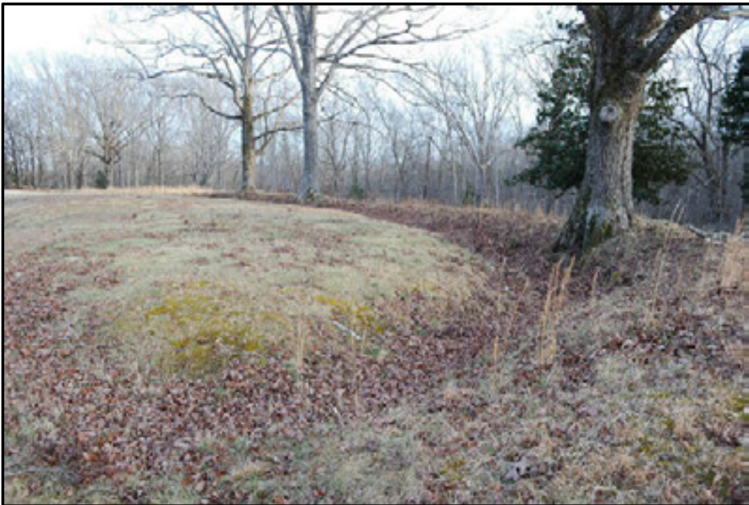
Figure 7.27. Segment 14, a large tree on the berm at the east end of the earthwork.
