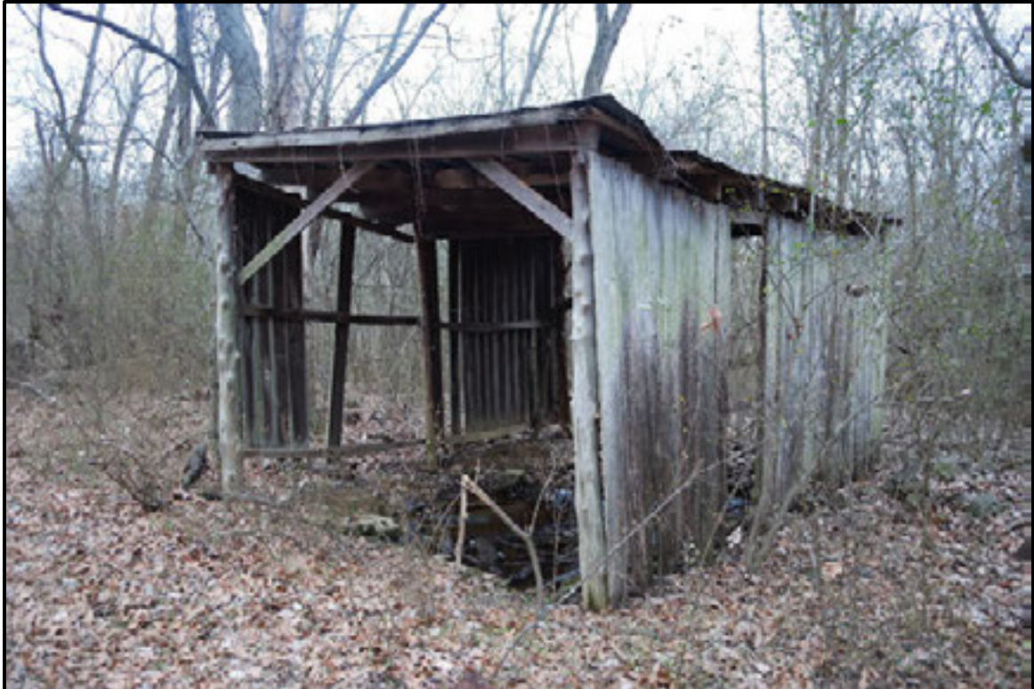
Figure 7.138. View of shed (Resource D).
