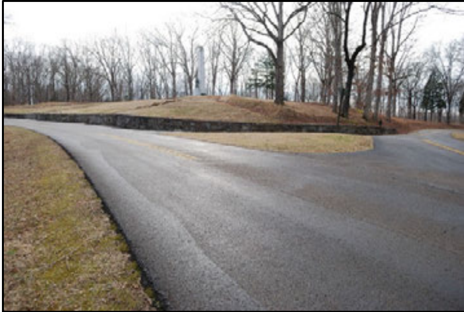
Figure 7.116. Overview of north side of retaining wall.
