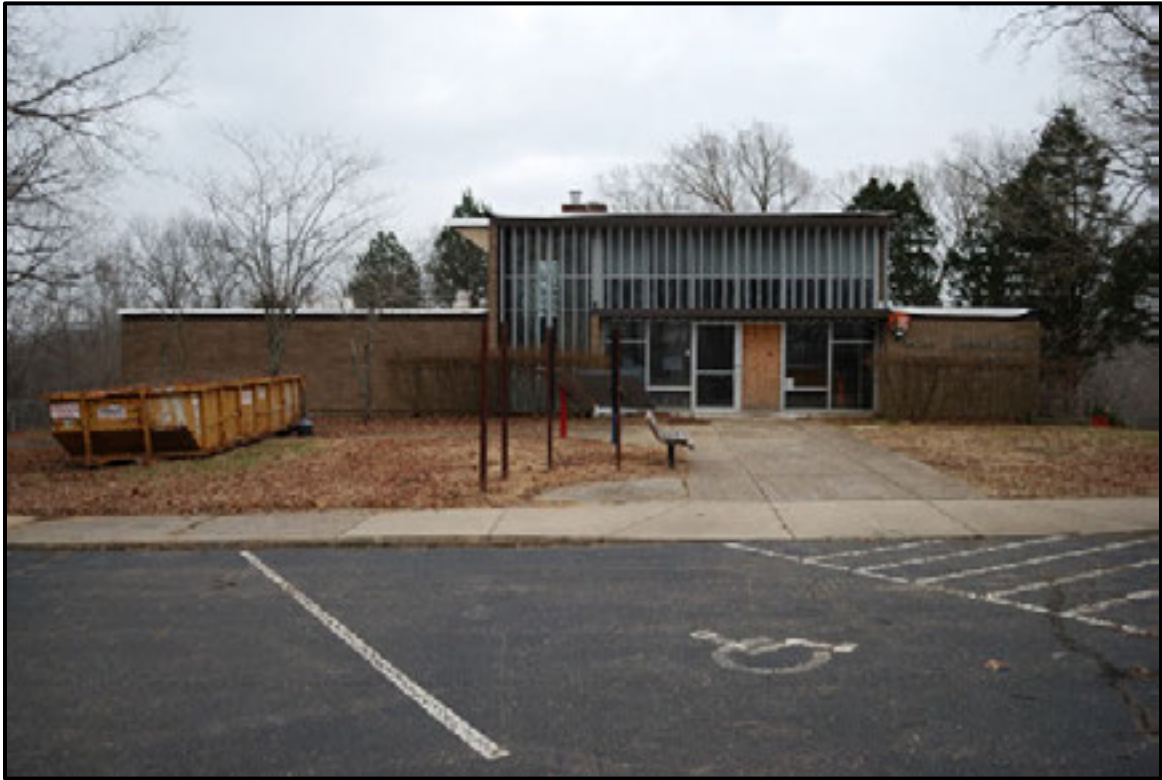
Figure 7.123. Façade of Visitor Center.
