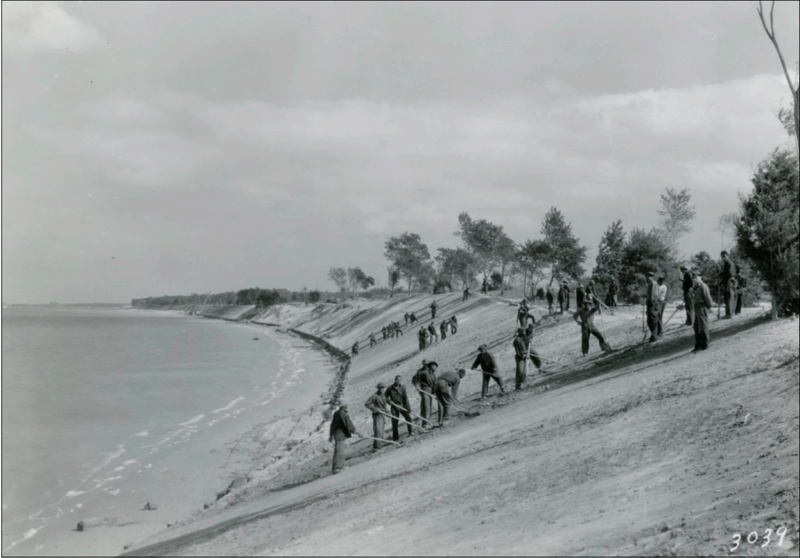
Figure 48. Here, enrollees in Company 2305 grade a sandbank in an effort to control erosion at Colonial National Monument. (Image courtesy of Colonial National Historical Park, Colonial National Monument Parkway Erosion Control, Grading Slope Prior to Placing of Sod to Prevent Soil Erosion, Sept. 1935, COLO 2962_3039).
