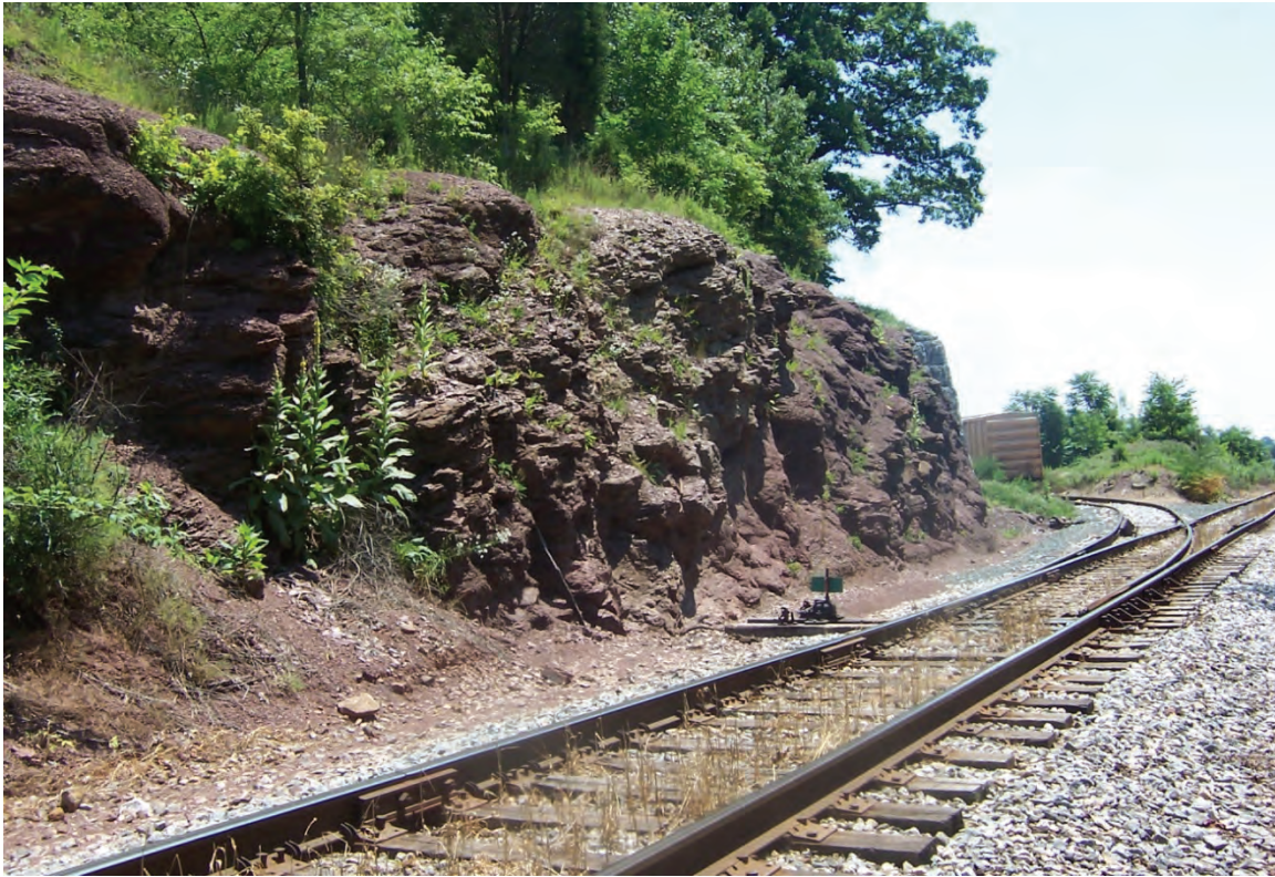
Figure 14. Exposed Sedimentary Strata. The railroad cut in Gettysburg National Military Park exposes strata from the Gettysburg basin. Image provided by Vince Santucci (National Park Service).
