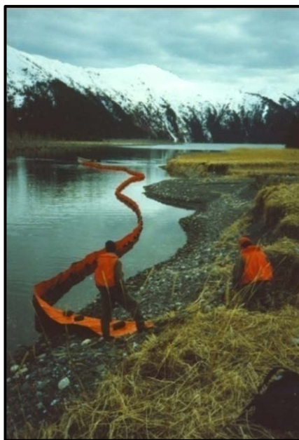
Placing boom to protect salmon streams in McCarty Lagoon; April 4, 1989.
