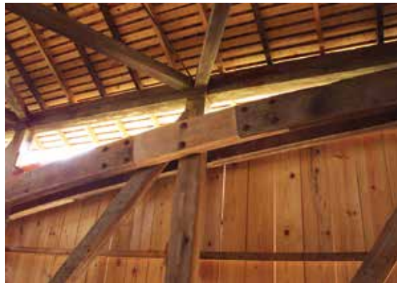
Figure 2.2 c-d A “brooming” compression failure in this arch required replacement of both the arch section and post. The repair salvaged all other sound timbers, and the splice was bolted in place. Comprehensive repairs to the Medora Bridge, IN, enabled the truss to once again carry its share of the load.
