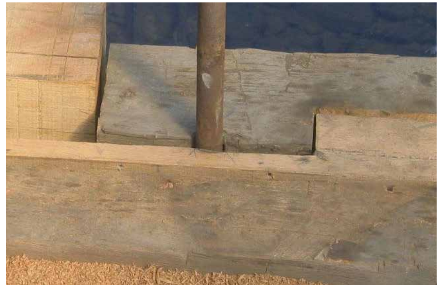
Figure C8.13 Joggle splice repair. SCLA.
