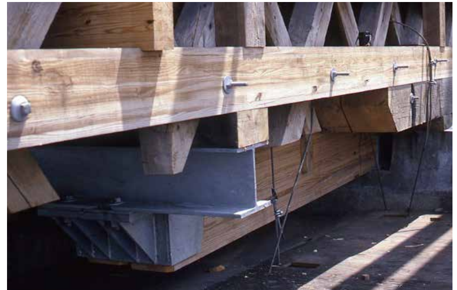
Figure C3.8 White oak bed timber and glulam bolster beam in new concrete footing, supporting truss. James L. Garvin, June 1989.
