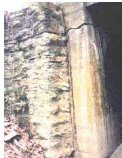
Figure C7.9 Cracks in concrete column and abutment at north end prior to rehab, KTC, ca. 2005.
