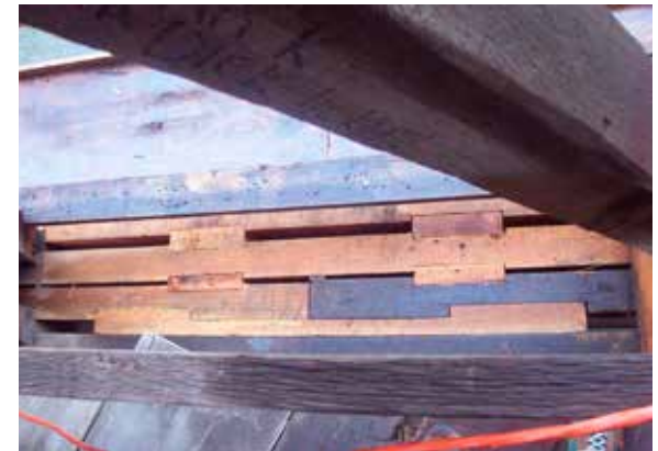
Fig 2.2e Metal bracing saved this rotted joint for years at the Eldean Bridge, OH, until an appropriate repair could be implemented. Figure 2.2f Lower chord timbers and fishplates replaced decayed members in an historically accurate manner.
