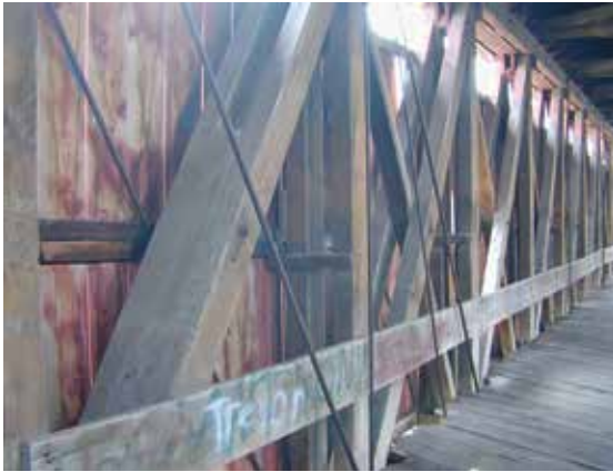
Figure 0.9a-c The 2005 rehabilitation work on the Eldean Bridge in Ohio is a good example of repairing and replacing missing historic character-defining features, and reversing an earlier inappropriate intervention. The 1960s reinforcing rods were removed on the 1860 Long truss, and replaced with wooden wedges driven in at the base of the diagonal counterbraces, thus prestressing the truss as prescribed by Stephen Long.
