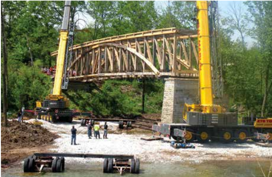
Figure C9.11 Lifting the first (shorter) span into place. Arthur Gatewood, 2010.
