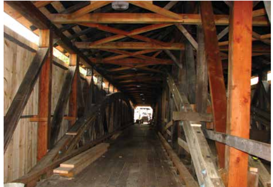
Figure C10.21 New upper lateral bracing and arches on eastbound barrel. William Caswell, September 2012.
