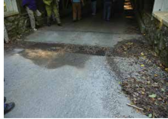
Figure 5.3c-d Storm grates are effective at protecting the bridge deck from runoff, but need to be maintained and cleared of leaves and debris to remain serviceable.
