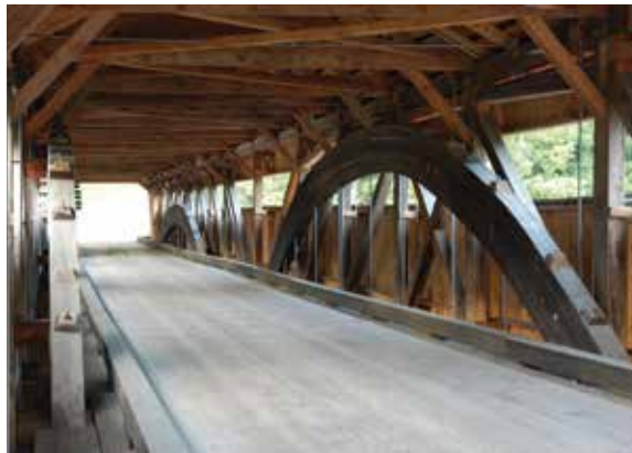
Figure 2.5c-d Riveted steel gusset plates were added in the 1950s at Taftsville Bridge, VT. This non-historical intervention was reversed during rehabilitation with traditional timber sway braces.
