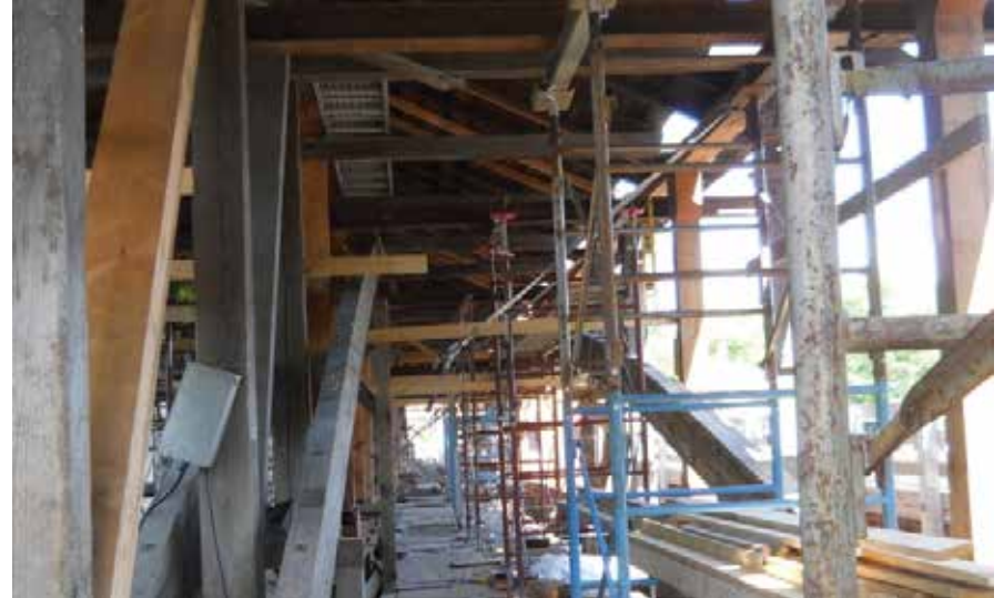
Figure C10.16 Temporary shoring system inside the bridge, looking east on eastbound barrel. Josif Bicja, July 2012.
