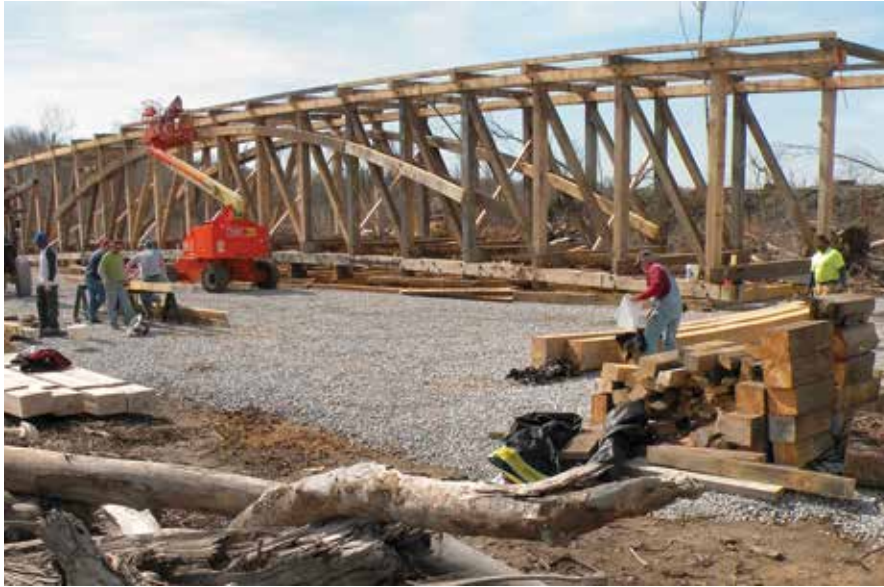
Figure C9.9 Start of framing for one span; blocking provides camber. Double notching visible at tops of posts. Arthur Gatewood, 2010.
