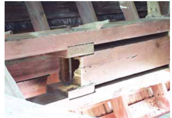
Figure 4.4e-f An example of mold accumulating on the bottom side of an arch member beneath a leaking roof. Below, internal decay found in upper chord timbers due to roof leakage. Both were repaired with limited replacement in kind.
