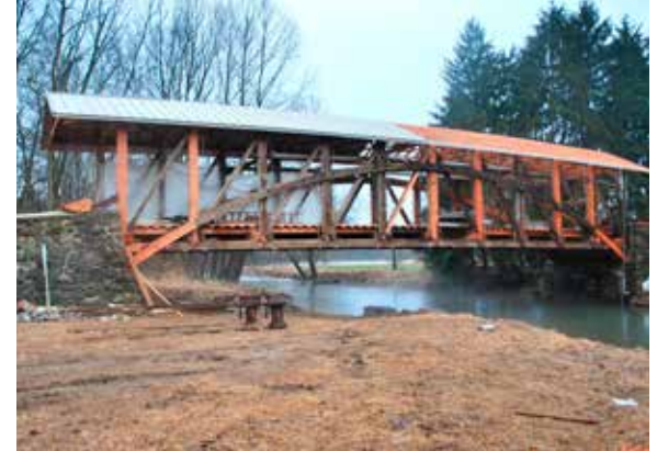
Figure 4.6e-f Decorative rake boards capping the roof overhang, matching shape and paint color in kind at Bowmansdale Bridge, PA. Below, a new standing seam roof being installed above a rehabilitated truss at Forry's Mill Bridge, PA.
