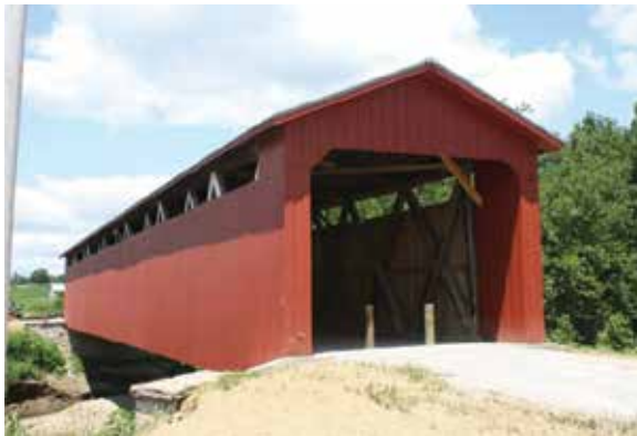
Figure 4.2 a-b Before/after views of the Engle Mill Bridge, OH. When rehabilitating the Smith truss, the bridge team re-sided and repainted in kind, maintaining the same openings to match the original.
