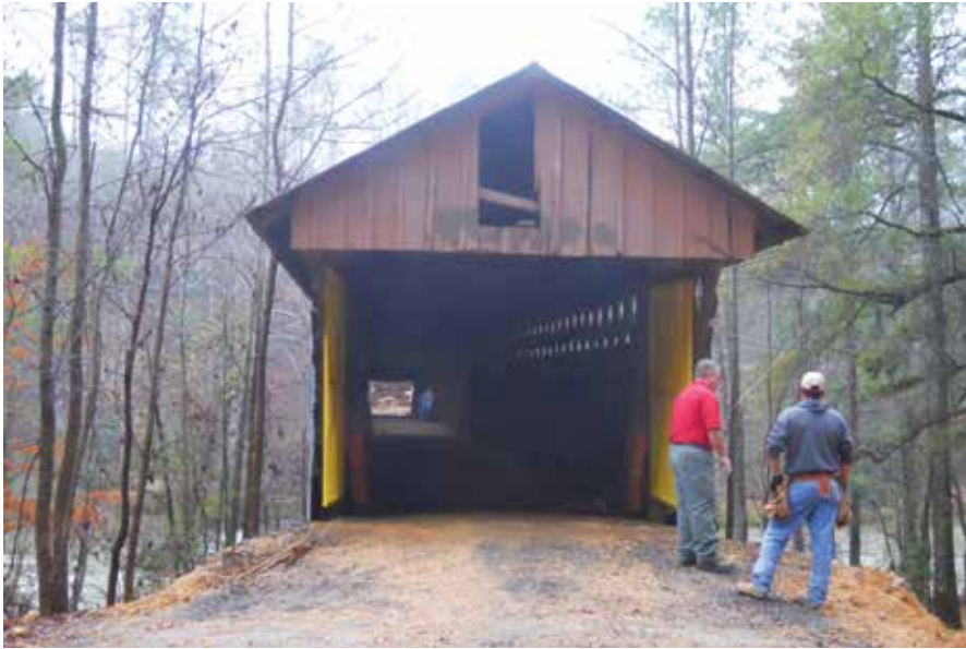
Figure C11.8 Abutment 1 showing gable with missing boards. TranSystems, 2012.
