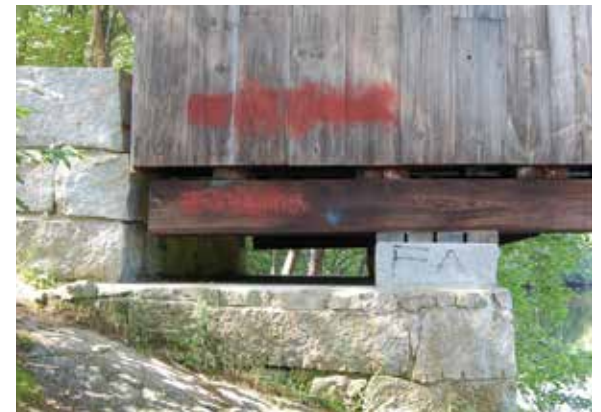
Figure 3.2e-f A circle of scour around a center pier at Medora Bridge, IN. Below, a bolster beam for a Town lattice truss at Henniker Bridge, NH. It sits on a granite pedestal, with spacer blocks below and on top, which allows for easy maintenance and good air circulation.
