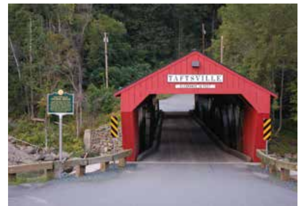
Figure 5.3e-f Repair and replacement of an approach sometimes requires replacement of the entire abutment and flooring system, such as at Knox Bridge, PA. Below: New steel-backed timber guardrails and historical marker after the reconstruction of the approach at Taftsville Bridge, VT.
