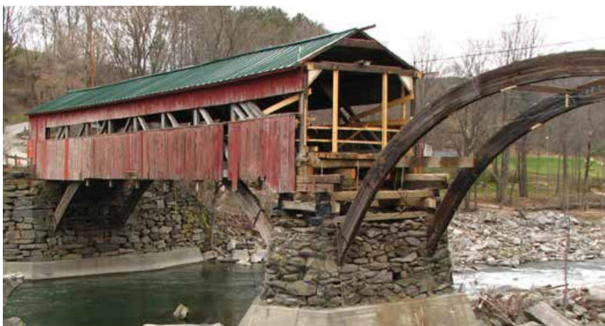
Figure 0.5a-b Vermont's Taftsville Bridge suffered major damage from Hurricane Irene in 2011. While one span needed to be completely rebuilt, a large percentage of the original hand-hewn truss members were salvaged and retained during the rehabilitation project.
