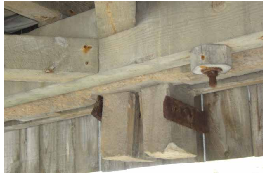
Figure C10.7 Typical split tail end of verticals at Node N12 (north truss). Josif Bicja, August 2007.
