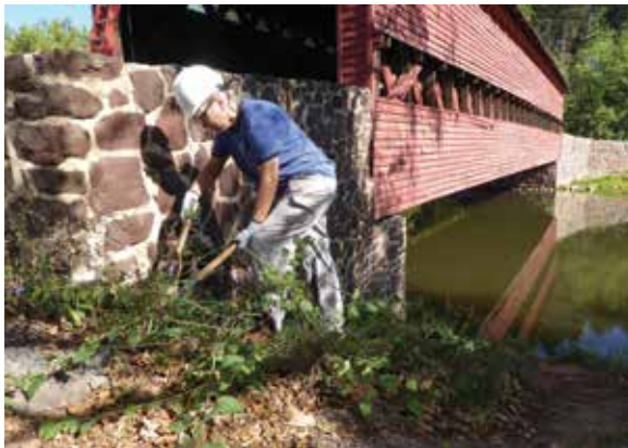
Figure 5.2a-b All traffic and safety signage should be placed in a prominent location, be clearly visible, and far enough away as to not detract from the appearance. Signage too close is not recommended. Below: Protecting the abutment by clearing the wingwall of invasives.
