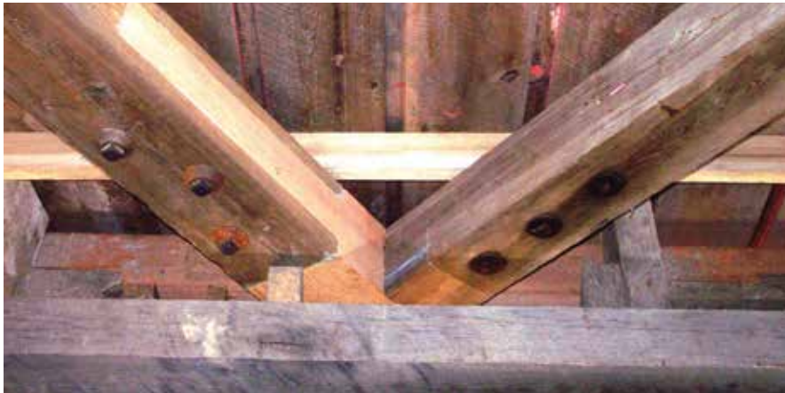
Figure C2.7 Timber repairs using new Douglas fir (left) were conspicuous. Those using salvage from original timbers (right) were nearly invisible. The Douglas fir repairs, having weathered a few years, are now less noticeable. J. A. Barker Engineering, 2004.
