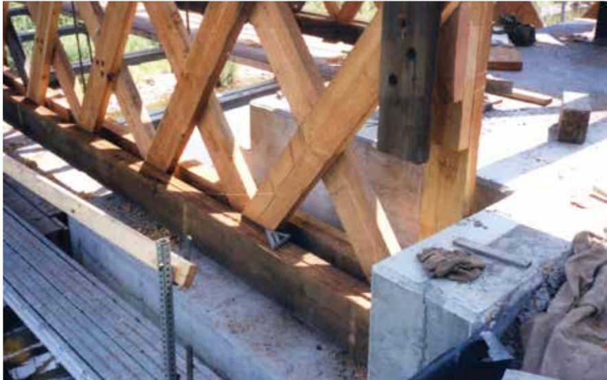
Figure C4.4 New concrete caps with pockets for longer trusses were installed on the abutments. DCDPW.
