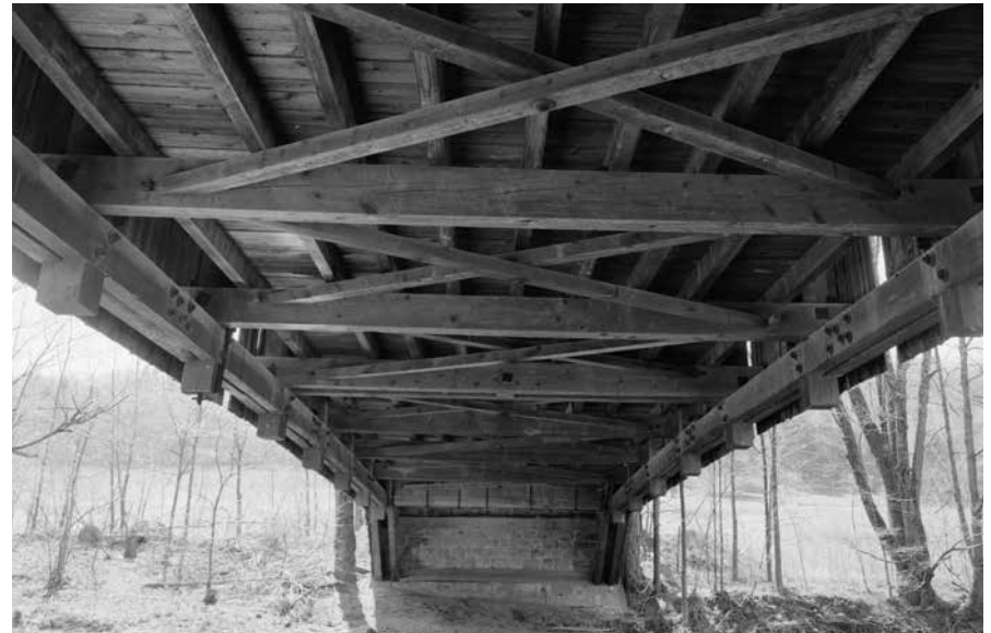
Stringer joists, laid parallel to the lower chords, sit atop the floor beams to support the deck.
