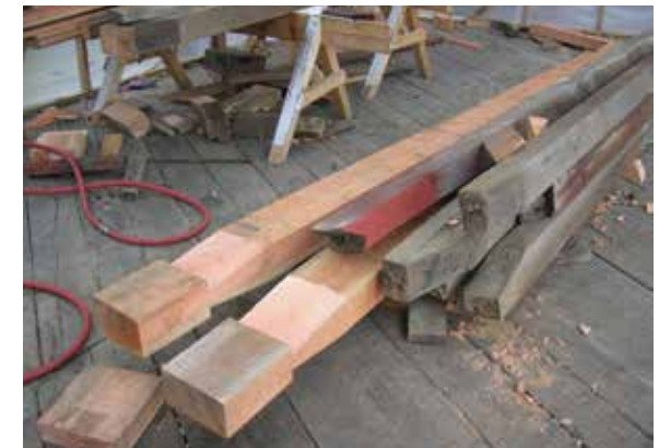
Fig 2.3e-f Replacement posts and diagonal braces at the Eldean Bridge, OH, matching the original craftsmanship of the historic Long truss.
