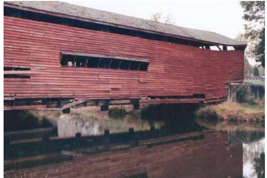
Figure C5.4 View of the bridge four years before the rehabilitation project. Failures in the lower chord contributed to the noticeable negative camber. W. Earl Simmers, 2005.
