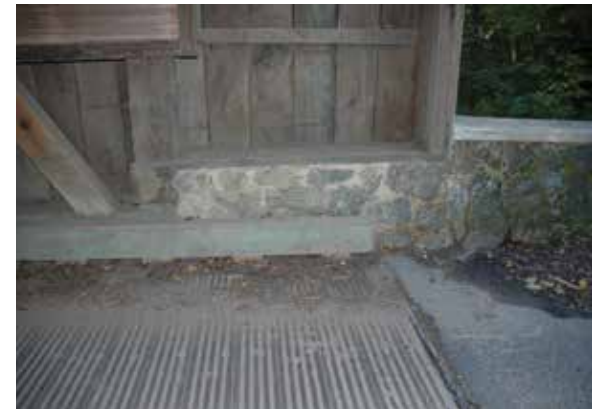
Figure 2.6e Diagonal decking found at Rinard Bridge, OH. Figure 2.6f Nail-laminated decking is typically not a historically correct treatment and should be replaced in most cases (unless it was the original decking system).
