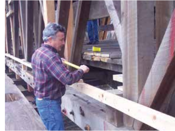
Figure 0.9a-c The 2005 rehabilitation work on the Eldean Bridge in Ohio is a good example of repairing and replacing missing historic character-defining features, and reversing an earlier inappropriate intervention. The 1960s reinforcing rods were removed on the 1860 Long truss, and replaced with wooden wedges driven in at the base of the diagonal counterbraces, thus prestressing the truss as prescribed by Stephen Long.
