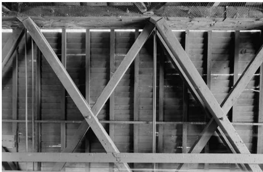
Paired, vertical iron tension rods in a Howe truss.
