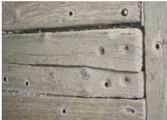
Figure 2.6c-d Newly installed longitudinal decking (running plank) at Forsythe Bridge, IN. Below, even a weathered and worn floor system should be inspected carefully to see if it could perform as required. Repairs and/or additional fasteners might preserve the floor's rich visual record of service.
