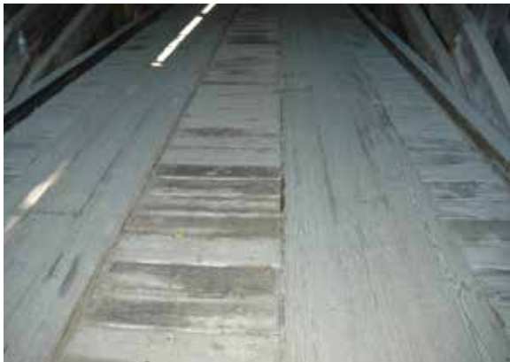
Figure 2.6a Transverse deck plank, laid below a curb and rub rail at Zumbrota Bridge, MN. Figure 2.6b Running boards act as a sacrificial wear surface, are often installed to accommodate heavier traffic, prolong the life of the decking, and can also act as a speed deterrent.
