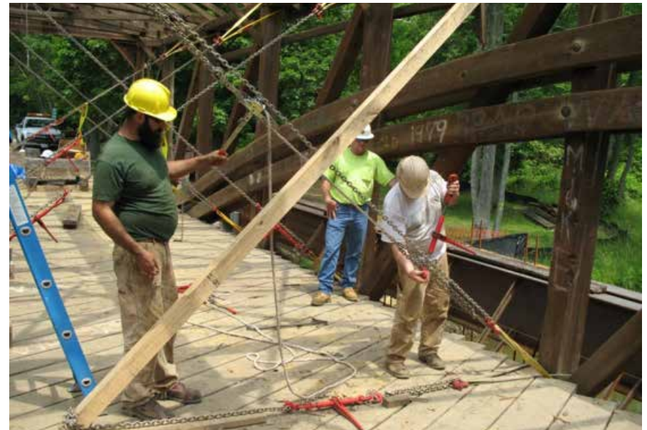
Figure C5.7 Cross chains installed to straighten the bridge in plan. Also note the deck planks are laid diagonally. The diagonal configuration was not original, and they were returned to a perpendicular arrangement later in the project. Jeremy Mauro, 2009.
