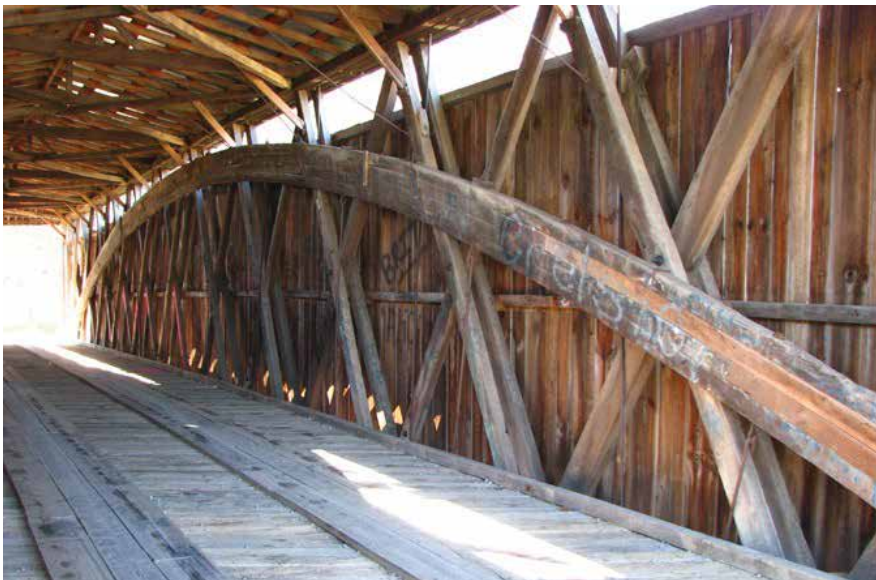
Figure C7.12 View of completed truss and deck, restored to its original geometry and camber. William Caswell, 2011.
