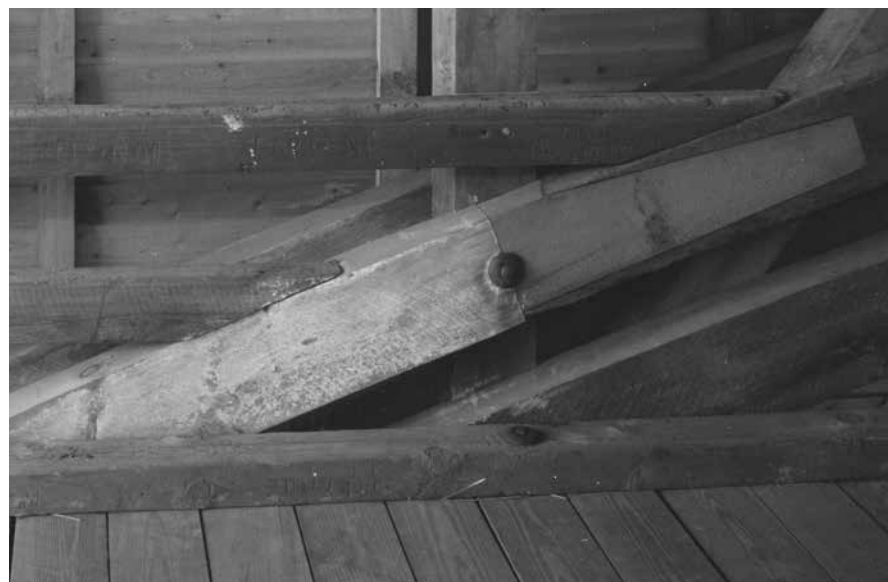
A splayed scarf joint repair abuts a replacement arch leaf. Both Burr-arch segments are secured with a single through bolt.
