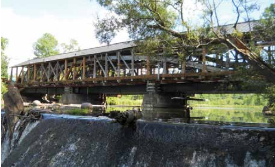
Figure C10.14 Downstream bridge elevation shored during construction, looking south. Two steel beams were installed on the underside of the bridge and fitted between timber cribbing at the piers. Josif Bicja, July 2012.
