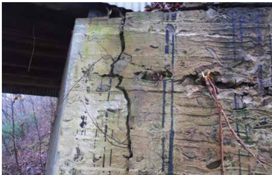
Figure C11.14 Wide crack in abutment 4 breastwall. TranSystems, 2012.
