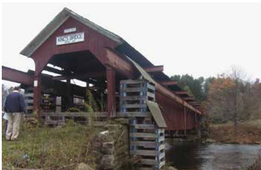
Figure C8.2. Bridge before rehabilitation with stabilization falsework in place at east portal. SCLA.
