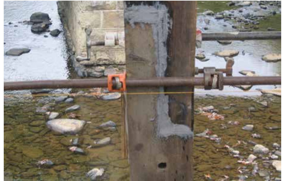
Figure C8.12 GFRP post repair. SCLA.
