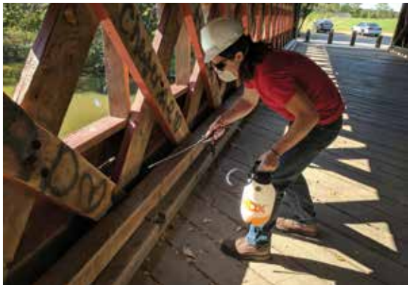
Figure 6.2a-b Sprinkler hose and solar panels protecting the Arthur A. Smith Bridge, MA. Below, spraying fire retardant on timbers as a fire prevention measure.
