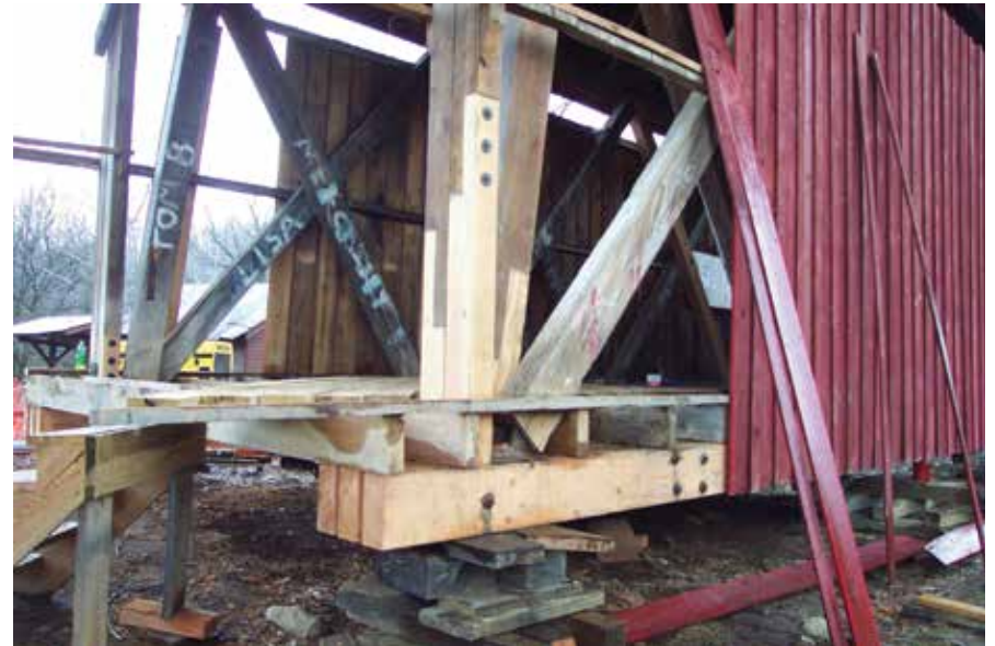
Figure C2.8 Decay at the bearings required extensive reconstruction. At the southwest corner, shown here, the two shorter lower chord timbers were replaced, while new ends were spliced onto the longest chord timber, both end posts, and a diagonal. J. A. Barker Engineering, March 2004.
