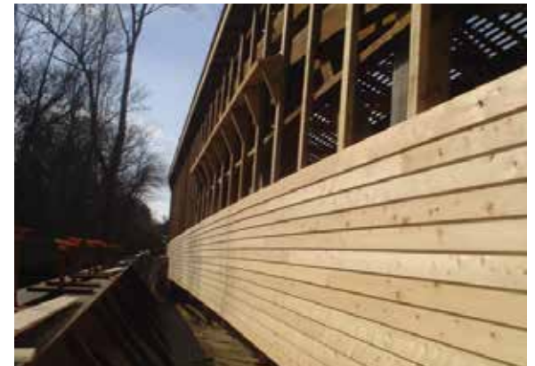
Figure 4.3e-f Replacement cedar siding in process of being applied to vertical nailers at Gilpin's Falls Bridge, MD. Above, pieces are individually trimmed to fit the shape of the portal. Below, note how the lap siding follows the camber of the bridge.
