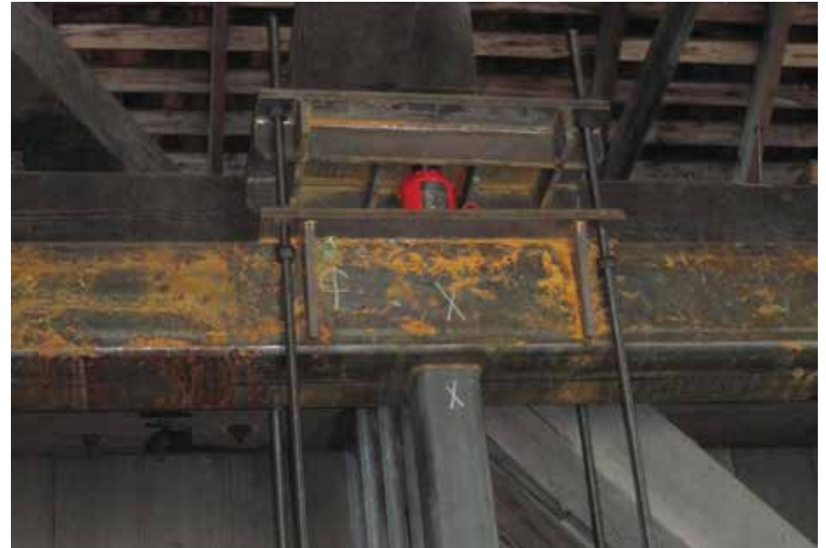
Figure C6.7 One of twenty 50-ton jacks on temporary steel truss used to lift the bridge to proper camber, 2013.
