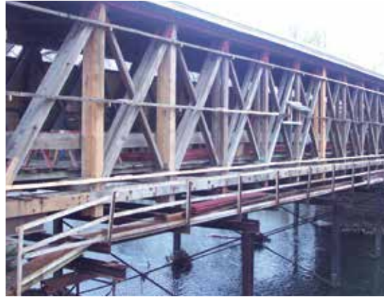
Figure 0.9a-c The 2005 rehabilitation work on the Eldean Bridge in Ohio is a good example of repairing and replacing missing historic character-defining features, and reversing an earlier inappropriate intervention. The 1960s reinforcing rods were removed on the 1860 Long truss, and replaced with wooden wedges driven in at the base of the diagonal counterbraces, thus prestressing the truss as prescribed by Stephen Long.
