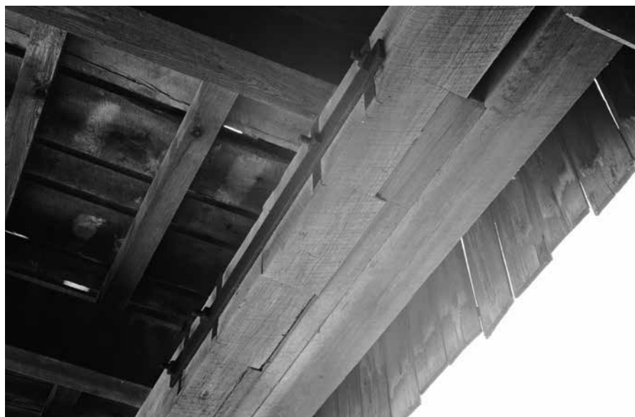
A tension splice with iron straps, strengthened with a shear key, connects two abutting sections of a bottom chord.
