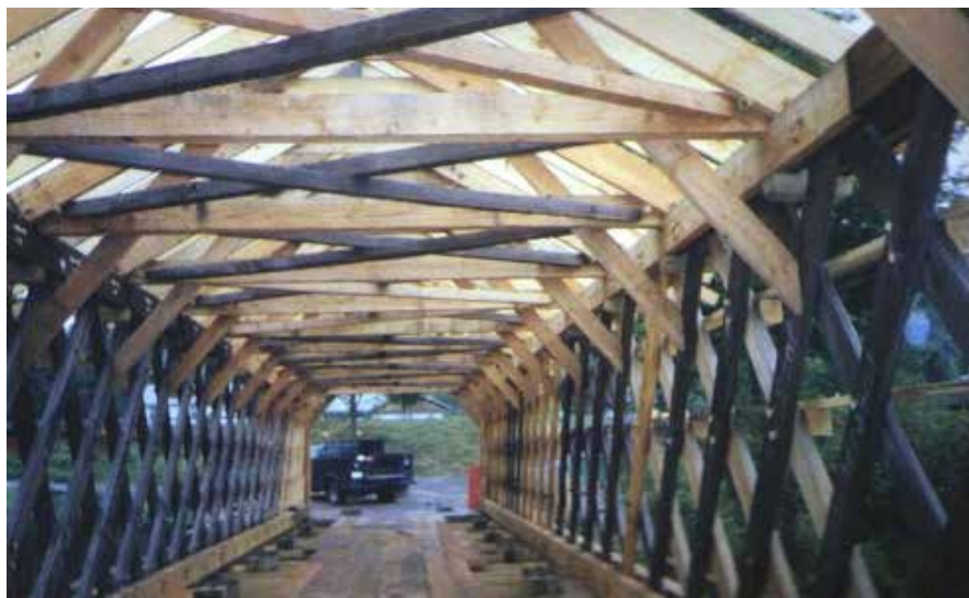
Figure C4.8 Most of the original upper lateral members were retained, but the tie beams and knee-braces were replaced with stronger components. Traditional wooden peg connectors and matching timber wedges were used, similar to those in the original construction. The darker upper lateral members are original. DCDPW.
