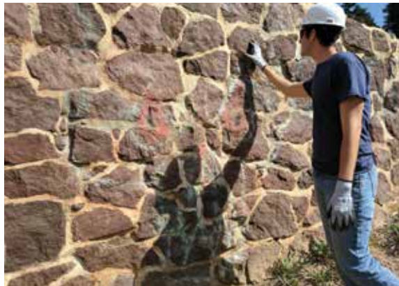
Figure 5.2c-d Original timbers with historic markings should be preserved as part of the historic fabric of the structure. Below: Graffiti from vandalism may be removed with a gentle cleaning through a low power pressure wash. A commercial stone mortar sealant can be applied to ease future graffiti removal.
