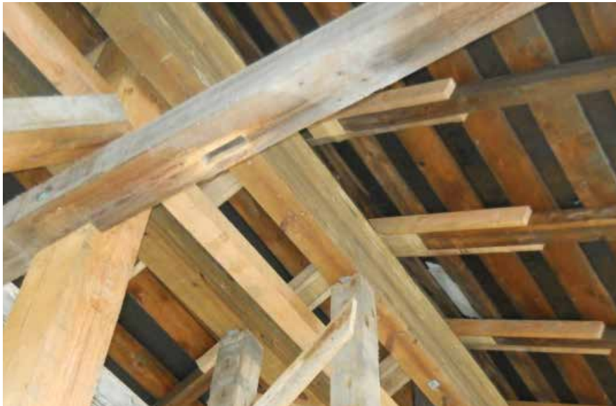
Figure C10.18 Typical sistered roof rafters. Josif Bicja, July 2012.
