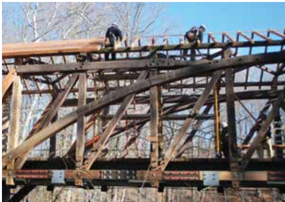
Figure 4.6a-b New roof rafters and purlins at Gilpin's are framed prior to receiving cedar shingles. Below, a harnessed crew laying out purlins prior to nailing cedar shake shingles at Jericho.
