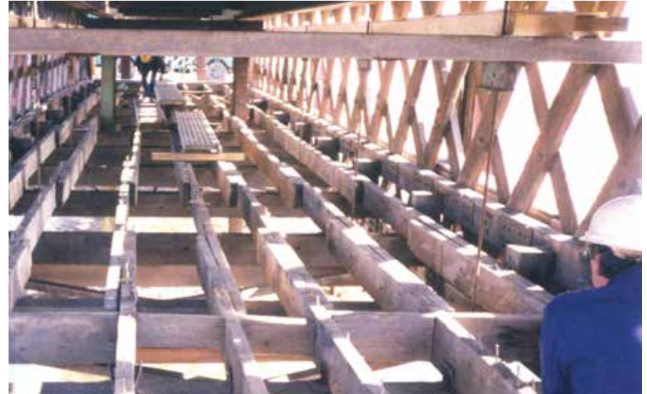
Figure C4.5 The 1976 floor system has been partially removed. The near edge of the floor is the transverse nail laminated decking. The longitudinal stringers are obviously not uniformly spaced. DCDPW.
