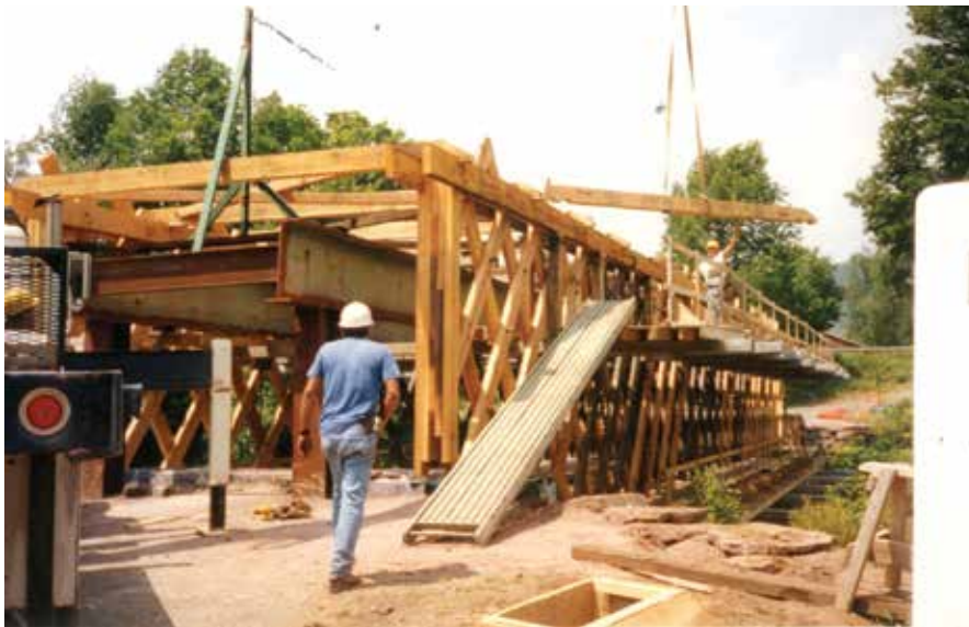
Figure C4.3 Prior to the start of the 2001 rehabilitation, a steel falsework system with adjustable work platforms was installed. This photograph shows the falsework and the installation of new tie beams. Delaware County Department of Public Works (DCDPW).
