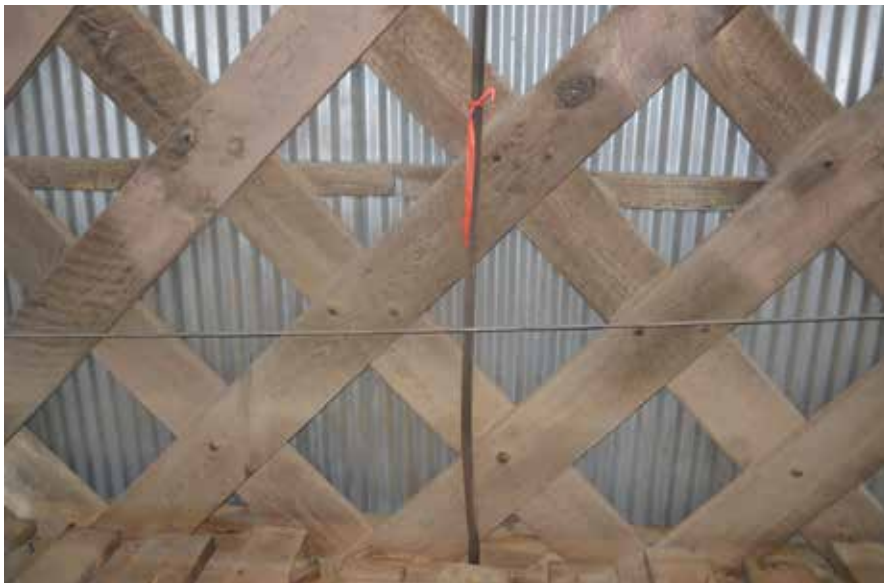
Figure C11.11 Span 3, south (right) side with bent hanger rod 1. Condition also observed at north hanger rod at floor beams 5 and 6. TranSystems, 2012.
