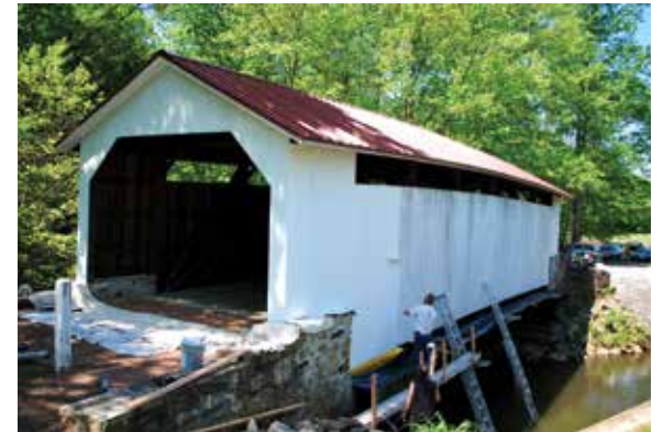
Figure 4.2e-f Local volunteers apply a fresh coat of bright white paint to the timber railings protecting the truss at the Esther Furnace Bridge, PA. Below, a new coat of white paint is applied to the exterior of the Henninger Farm Bridge, PA.
