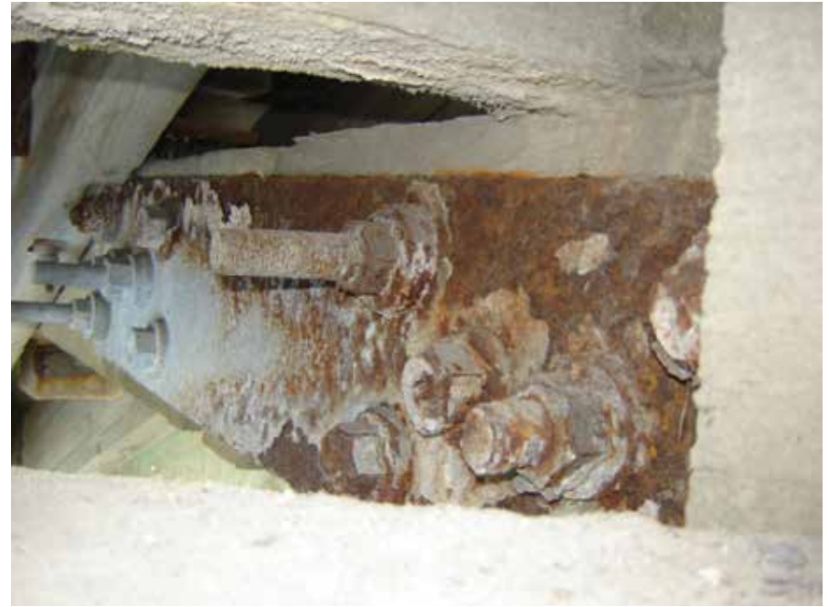
Figure C10.5 Severely corroded splice plate of interior truss at west span. Josif Bicja, August 2007.
