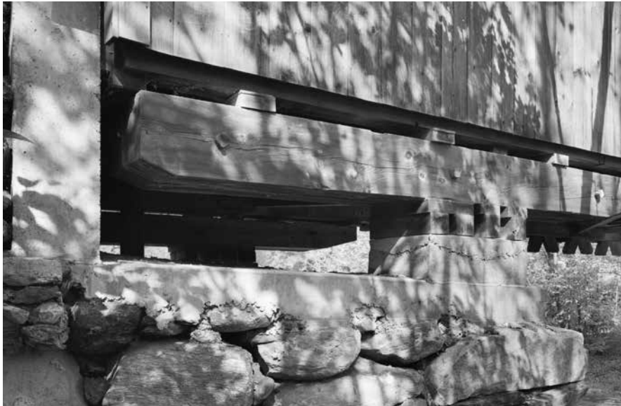
Bolster beams supporting a Town lattice truss. Note the bearing blocks used as spacers beneath the lower chord.
