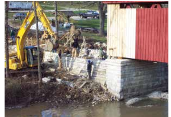
Figure 3.3e-f Reconstructing the dry-laid wing wall behind the abutment at Cataract Bridge, IN. The reconstructed wall matches the original in composition, color and texture, while improving its strength.
