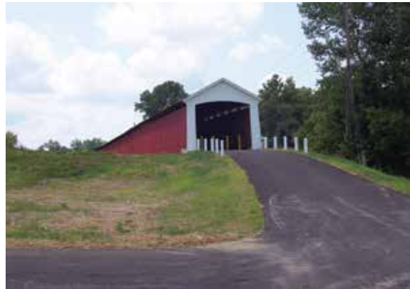
Figure 5.3a-b This deteriorated country approach road at Medora Bridge, IN, required regrading and new paving to maintain the alignment of the historic approach.
