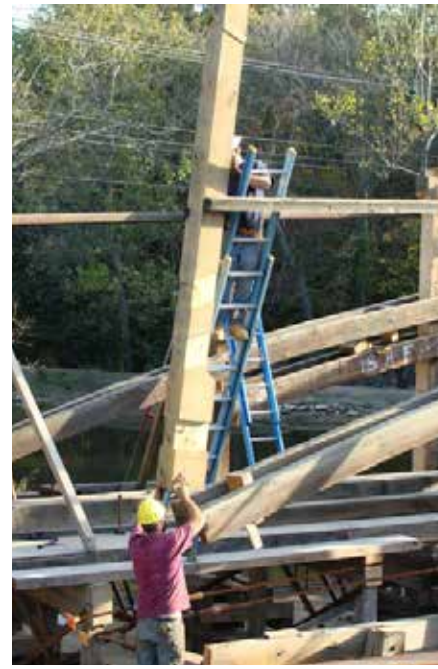
Figure C5.8 Tim Andrews (top) and Jeremy Woodliff (below) guide a new end post into position. A crane, not shown in the photo, is lowering the post. Tim Andrews, 2009.
