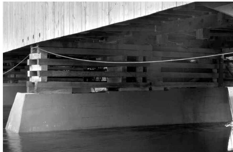
Replacement timber cribs sit atop concrete piers to support the Pulp Mill Covered Bridge, VT.
