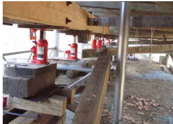
Figure 1.3c-d Using come-alongs to correct the raked truss geometry and negative camber at Gilpin's Falls Covered Bridge, MD. Below, after the crew moved the Cataract Bridge, IN, off its abutments, they used bottle jacks to gradually restore camber beneath a replacement lower chord.
