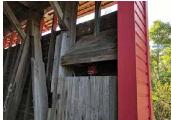
Figure 6.2c-d Emergency fire suppression system placed beneath the bridge out of view of the main truss; fire alarm housing subtly tucked inside a shelter panel at Utica Mills Bridge, MD.
