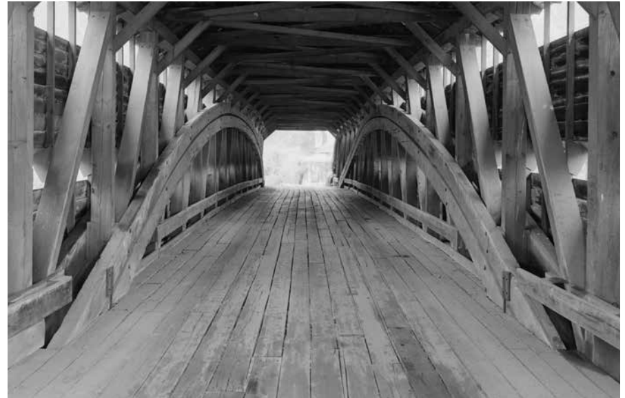
A second layer of longitudinal floor-planked bridge deck serves as the wearing surface for this Burr-arch truss.
