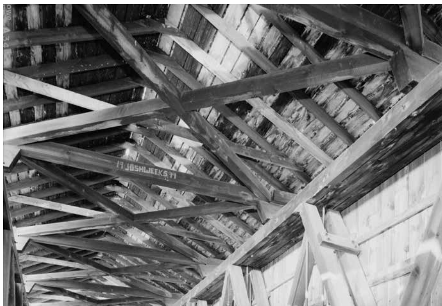
An upper lateral bracing system, with a series of knee braces at every tie beam.
