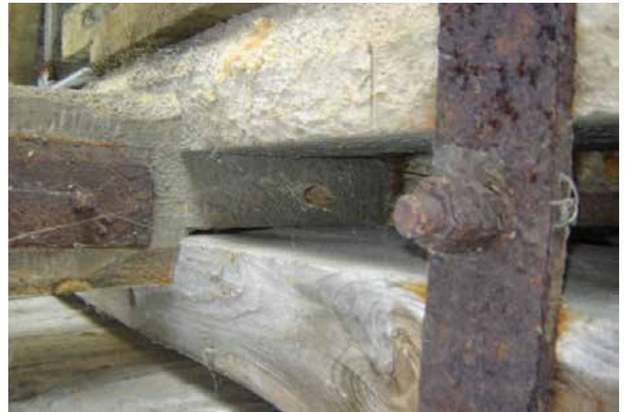
Figure C10.8 Notched end of vertical at connection with bottom chord at Node N4 (north truss).
