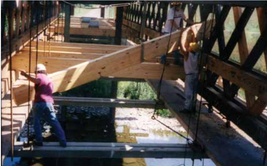
Figure C4.6 New transverse glulam floor beams were carefully threaded through the lattice opening-satop the lower bottom chord. DCDPW.
