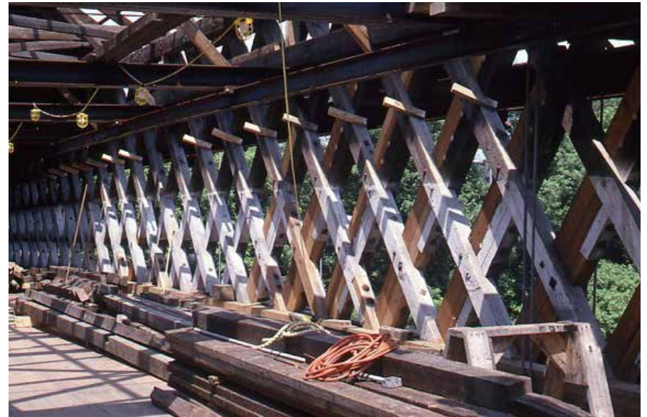
Figure C3.5 Town lattice sistering. James L. Garvin, June 1989.
