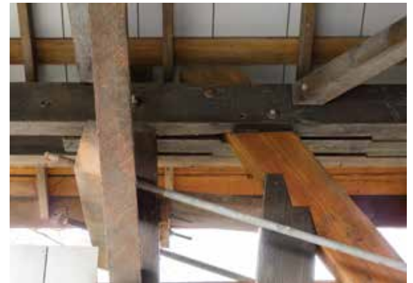
Figure 2.5e-f An example of a loose diagonal brace with traditional stepped notches in need of adjustment. Below, a replacement tension diagonal matches the double-stepped connection of the original post in a Smith truss at Rinard Bridge, OH.
