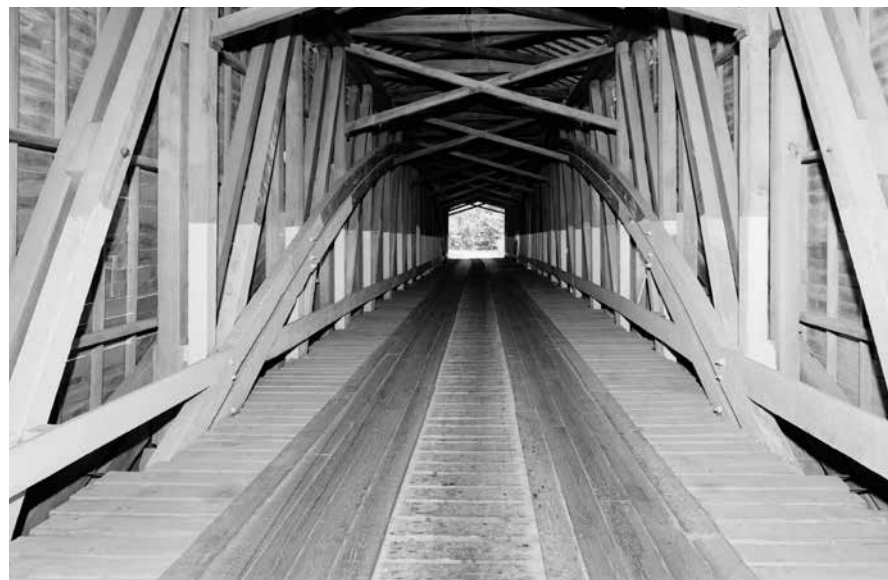
Running planks laid atop transverse decking provide an added layer as a wearing surface.
