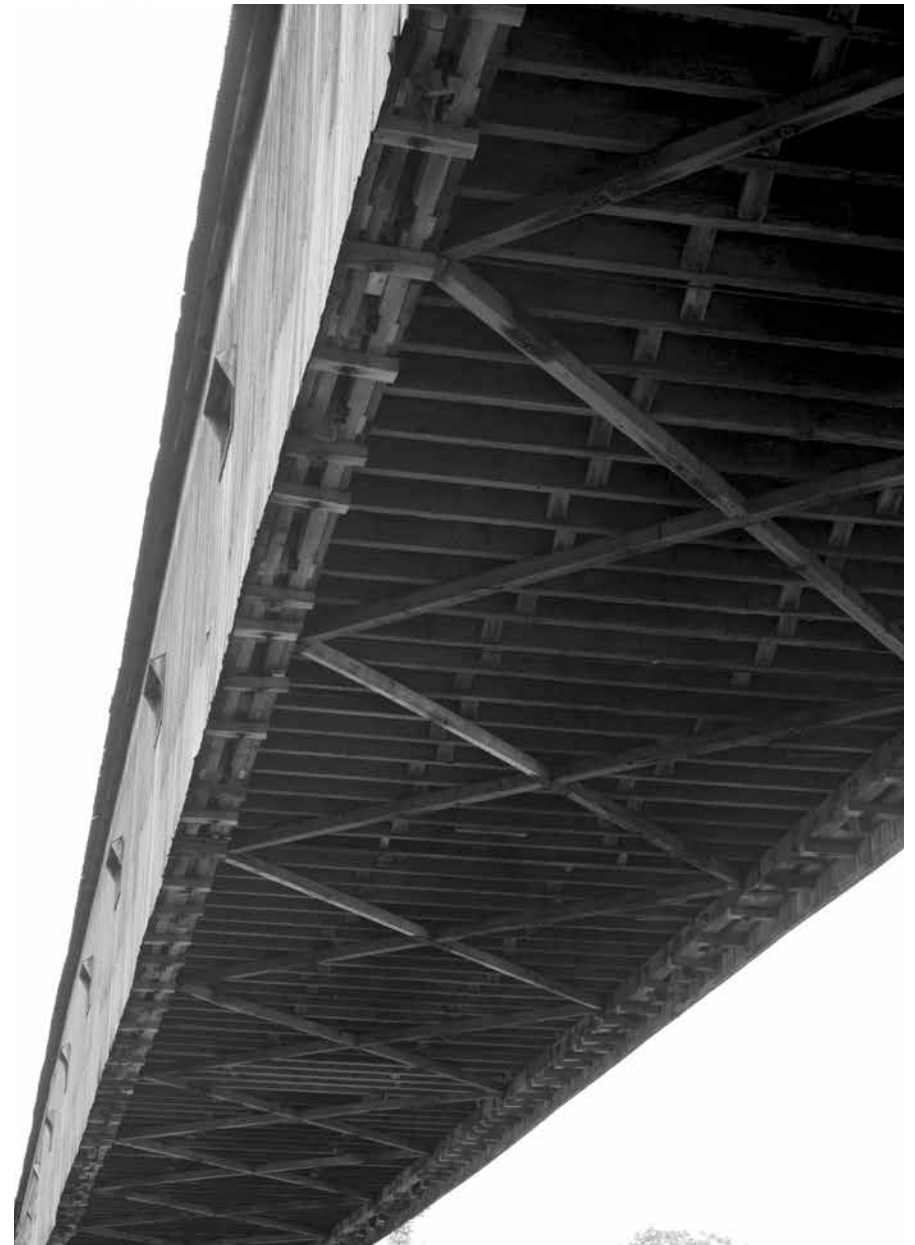
Figure C3.2 View inside bridge showing notched lattice truss, prior to being closed. HAER NH-8-10, Jet Lowe, 1984.
