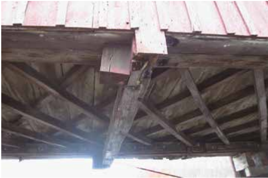
Figure C8.4 Lattice floor joist system, and lower tie beam added after original construction. SCLA.
