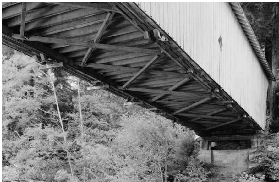
Bottom chords, lower lateral bracing, and floor joists support this Smith truss.
