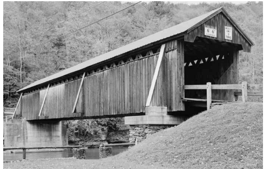
Flying buttresses or outriggers outside the trusses help control the vertical alignment of the bridge.
