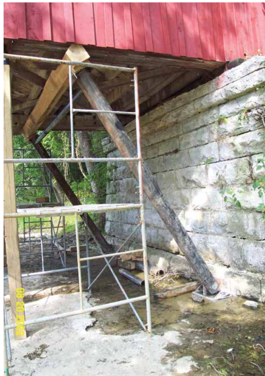
Figure C2.4 Temporary shoring installation. J. A. Barker Engineering, August 2002.
