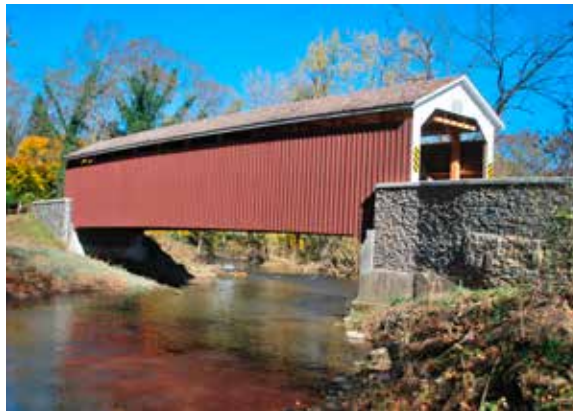
Figure 4.6c-d After the Siegrist's Mill Bridge, PA, was lost in a flood, the replacement Burr-arch truss was replaced in kind. Above, using a bucket lift to install the replacement shingle roof. Below, the bridge shown fully sheathed.
