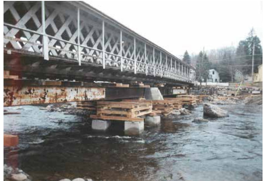
Figure C1.8 Shoring underneath bridge. Sean T. James, 1998.
