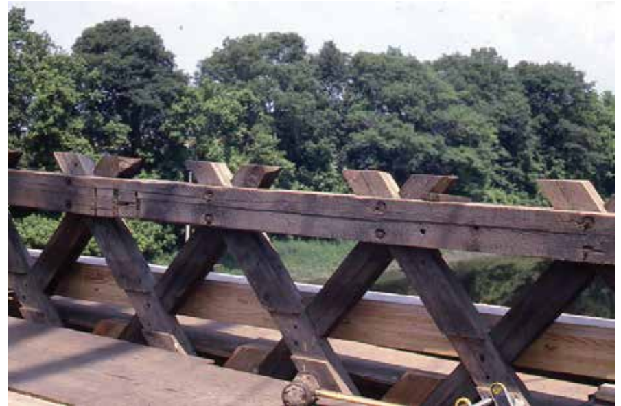
Figure C3.4 Above central pier, showing removal of Chord 3. James L. Garvin, June 1989.
