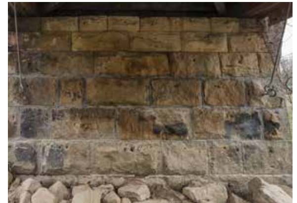
Figure 3.4e-f Chinking (filling joints with small stones) rather than the introduction of mortar is the proper rehabilitation method for a dry-laid wall. Below: Preserving the original stonework at Rinard Bridge, OH. The hold down rods (an original design feature) have been replaced in kind, which helps keep the bridge in place during a flood event.
