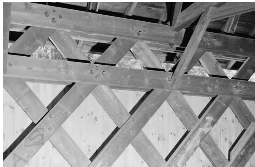
Treenails are paired at lattice intersections, and in a diamond pattern at the upper and lower chords.
