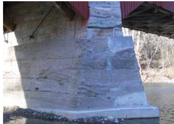
Figure 3.4c-d Structural failure due to cracking in the center pier at Deers Mill Bridge, IN. The crack was patched and a new concrete apron poured underneath to stabilize the pier.
