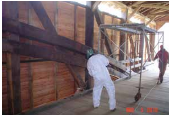
Figure 4.2c-d Conducting an inspection to assess the condition of the siding and painted surface. Below, a technician wears a protective suit and uses a high pressure sprayer to apply fire retardant to the truss and interior siding.
