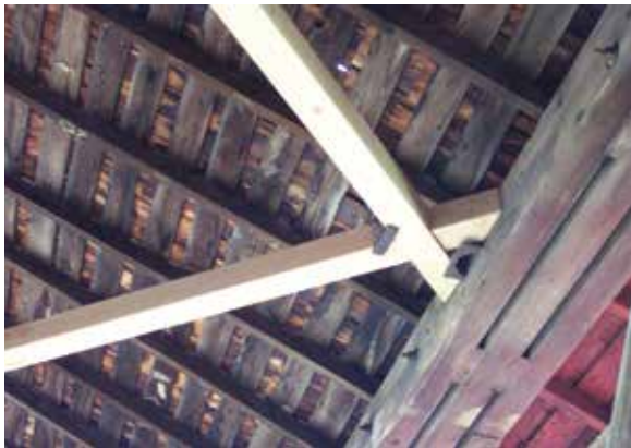
Figure 2.5a-b Original upper lateral bracing members of the Smith truss at Cataract Bridge ,IN, had rotted due to a leaking roof. They were replaced in kind, keeping the original hardware.
