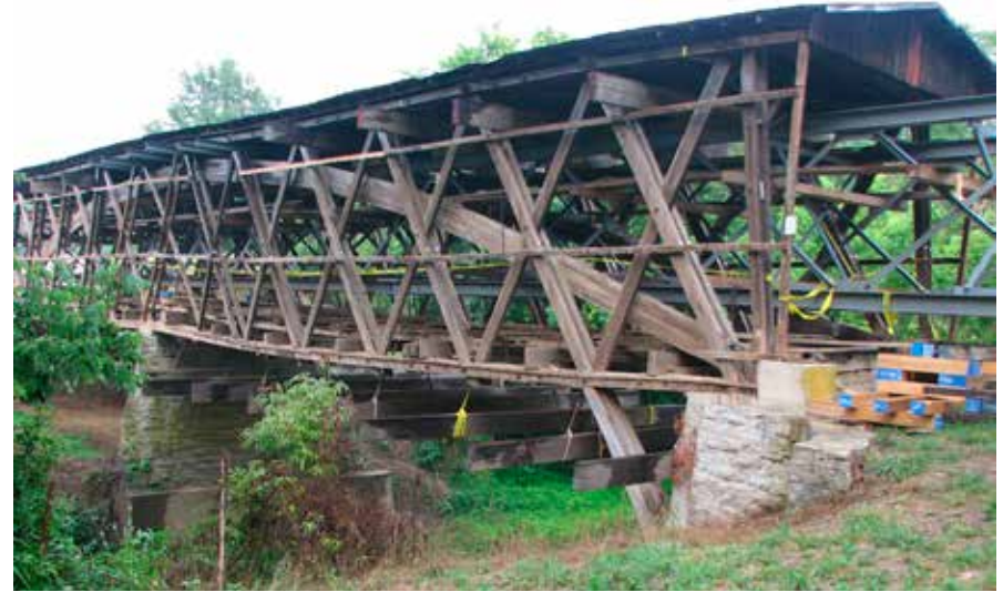
Figure C7.5 View of shoring system, with steel truss through bridge, with horizontal needle beams supporting the top chord. Note negative camber, which measured up to 21." William Caswell, 2007.
