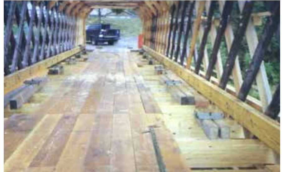
Figure C4.7 Staggered longitudinal deck planks have been installed; these were then covered with hardwood running planks. Note the darker lattice elements, which are original. DCDPW.
