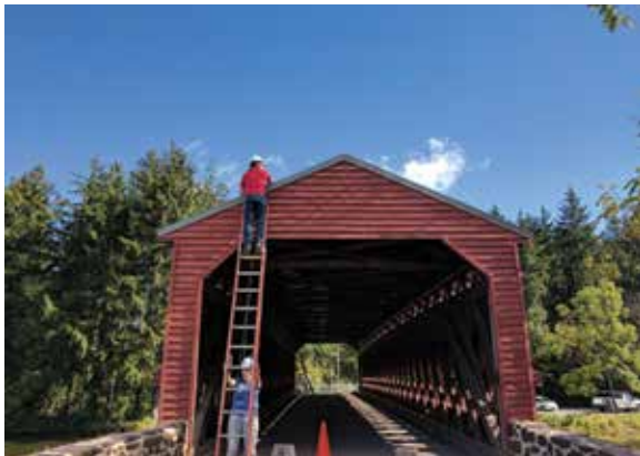
Figure 4.4a-b Scraping off mud dauber nests to keep roof and truss components free from infestation. Above, an engineer performs a periodic inspection of the roof covering.
