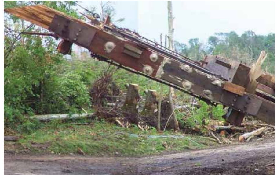
Figure C9.6 Pulling the bridge out of the water. Previous repairs included liberal use of epoxy adhesives, making it impossible to reuse these lower chord timbers. James Barker, J.A. Barker Engineering, Inc., 2008.
