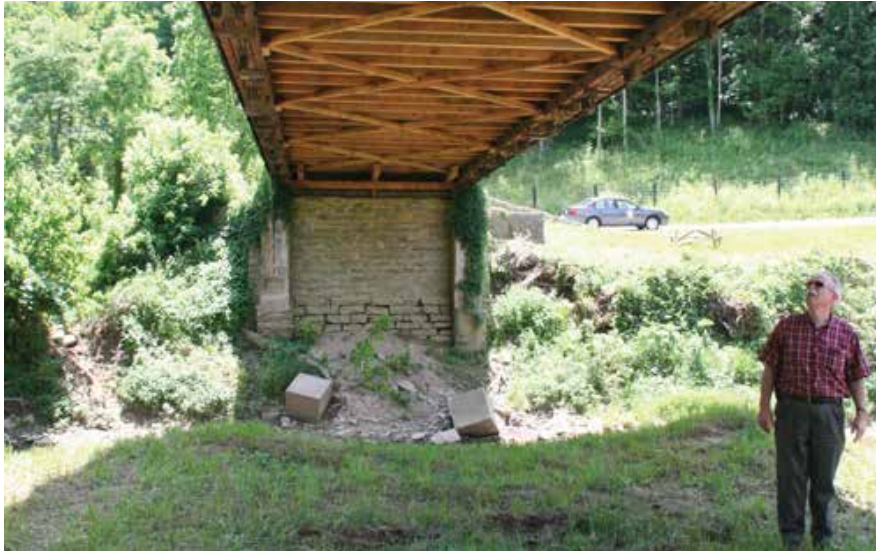
Figure C7.11 Patrick Kennedy inspects the rehabilitated lower chords and flooring system, Jen Spangler Williamson, 2010.
