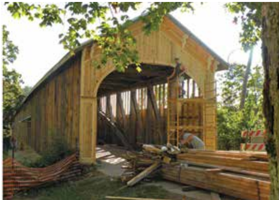
Figure 4.3a-b Although a tornado destroyed most of the Moscow Bridge in Indiana, its Kennedy Bridge character-defining features: vine decorations, roof brackets, and elliptical arch opening were carefully reconstructed, before being painted its original white.
