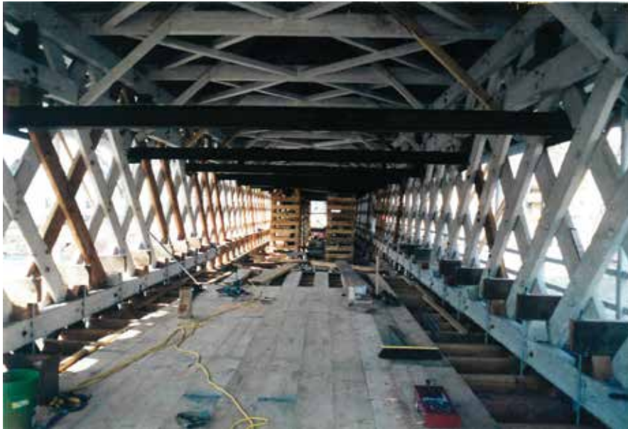
Figure C1.12 Installation of floor beams and decking; note steel needle beams supporting the top chord, spaced at every third lattice opening, 1998. Sean T. James, 1998.
