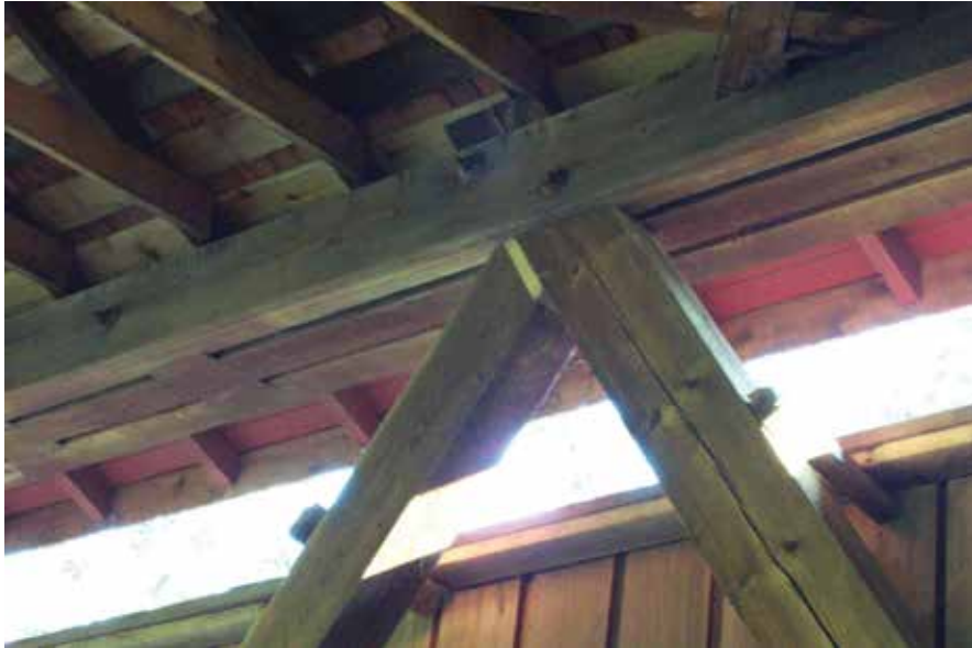
Figure C2.9 Trusses were jacked to restore camber, then held in that position by inserting shims at the top of truss compression diagonals, as shown here. J. A. Barker Engineering, 2004.
