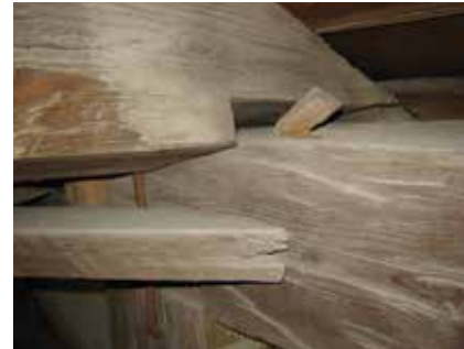
Figure C10.10 Twisted cross beam and bracing to top chord connection near Node N14.
