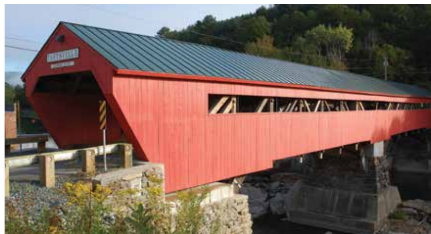
Figure 0.5a-b Vermont's Taftsville Bridge suffered major damage from Hurricane Irene in 2011. While one span needed to be completely rebuilt, a large percentage of the original hand-hewn truss members were salvaged and retained during the rehabilitation project.
