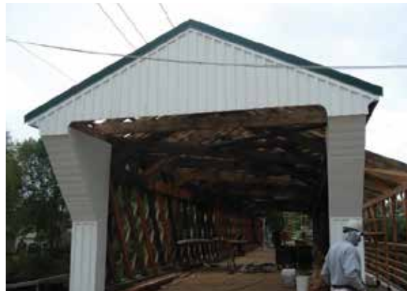
Figure 4.3c-d After the Town lattice truss was rehabilitated, the exterior board-and-batten siding was replaced in kind, and a new standing seam metal roof installed at the Newton Falls Covered Bridge, OH.
