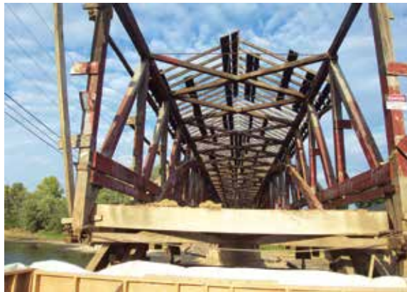
Figure 4.4c-d A neglected, porous roof allowed moisture and mold onto the truss and lateral bracing below. After removal, most of the bracing and rafters were repaired and kept intact, and a new shingle roof was replaced in kind.
