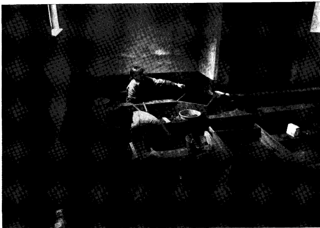
Figure 29. Crawlspace excavations in progress.
