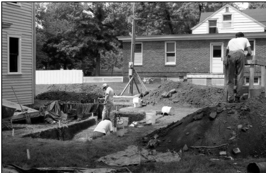
Figure 7. Overview of block excavation area.
