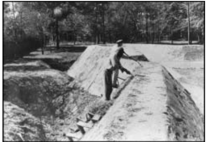
FIGURE 33. Reconstructing earthworks at Fort Raleigh, 1950
