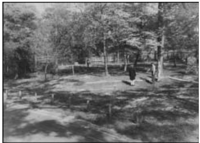
FIGURE 31. Earthwork outlined by granite, ca. 1949
