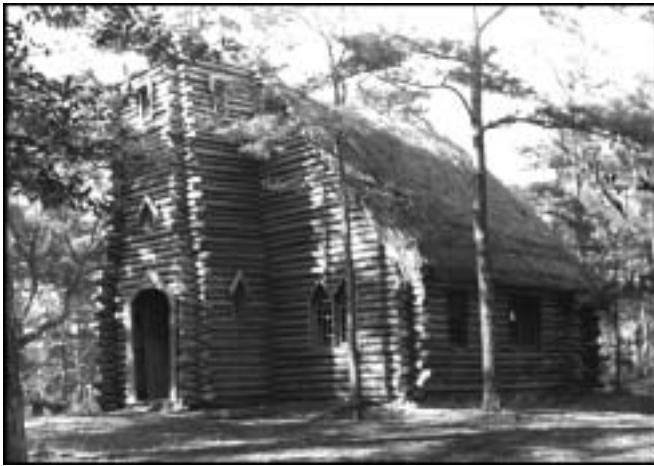
FIGURE 17. The WPA chapel at Fort Raleigh, January 1938
