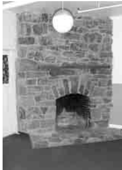
Corner fireplace in Deluxe Guestrooms. Note obtrusive contemporary light fixture. 2001 Courtesy Glacier National Park
