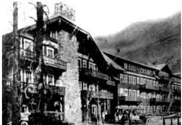
East side of hotel with tourists waiting to board the "Old White" touring buses. 1920 Note stone chimney at entry, flag pole supports, and balconies without extensive "add-on" supports (steel angles, cables, wood posts). Courtesy Glacier National Park Archives
