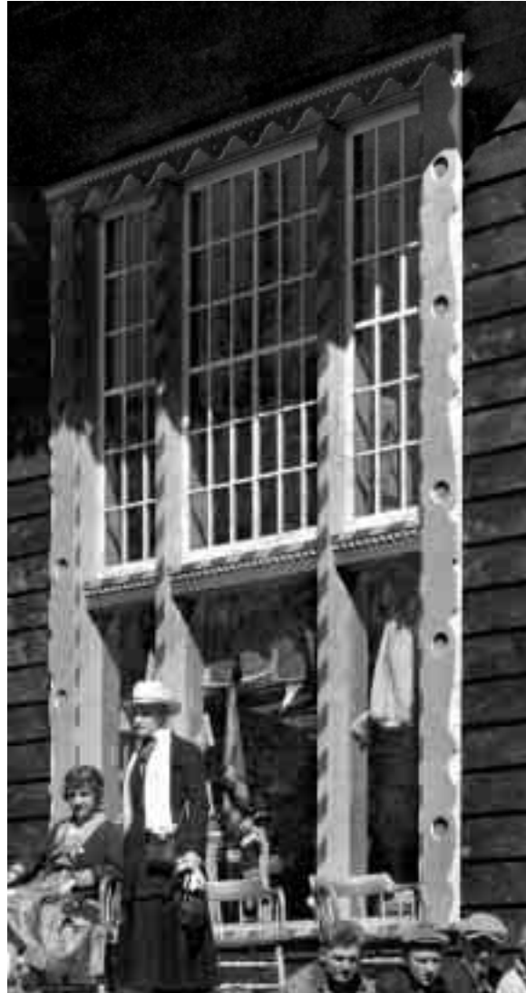
Lobby window. Note diagonal striping on vertical trim. Cut-out circles in perimeter trim were originally designed and in fact believed to be painted blue in color. Courtesy of Glacier National Park Archives
