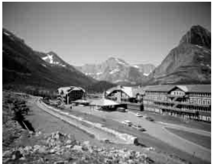
Photograph displays siting of Many Glacier Hotel. Note porte cochere spire attempting to mimic lower spire over original south bridge to left. Courtesy Glacier National Park Archives
