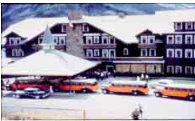
Porte Cochere developed at main entry to hotel to protect guests from "the elements." Courtesy Glacier National Park Archives
