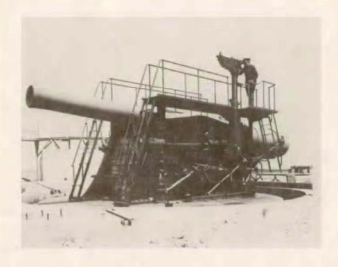
Photograph No. 20. Army designed turret mounted 14-inch rifles tested at Sandy Hook Proving Ground, ca. 1908-10.
