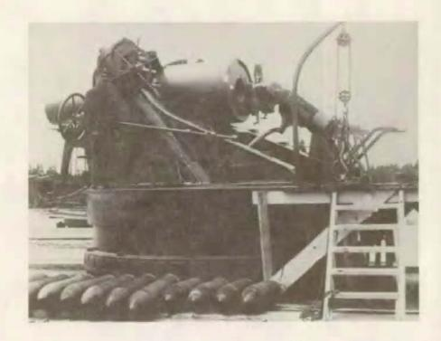
Photograph No. 14. Buffington-Crozier counter weight carriage field tests, ca. 1894.
