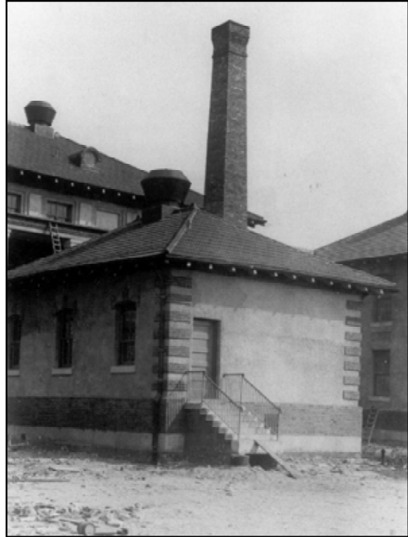
Figure 4.16 Upon completion of the mortuary (animal house) on Island Three, there was still a considerable amount of fill needed to raise the island's grade to its planned elevation. Notice the distance between the bottom of the staircase and the rough grade prior to the addition of topsoil fill. October 14, 1907. (National Archives and Records Administration, RG121-BCP-38A-3)
