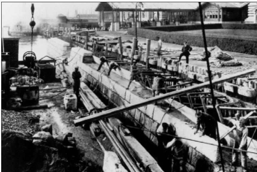
Figure 4.17 In 1913 construction began on the new concrete and granite seawall on Island One. This image of construction on Contract #1 shows how the new seawall was placed outside the existing crib bulkhead, reducing the width of the ferry basin by about thirty feet when the north and south basin seawalls were completed. Circa 1913. (STLI Library, 26.7, #16)
