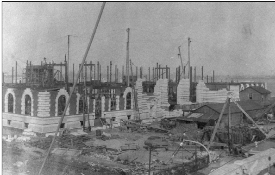
Figure 3.2 Construction of the main immigration building. Notice the wooden fence remaining from the earlier building in the foreground. June 30, 1899. (National Archives and Records Administration, RG121-BCP-37D-6)
