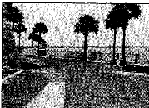
Figure 13. View of water battery from south, 1991
