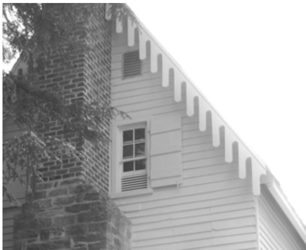
FIGURE 51. View of west gable. (T. Jones, NPS, 2004)
