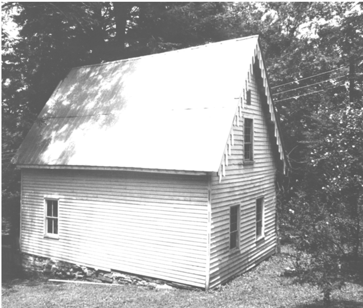
FIGURE 33. View of Swedish House, 1971. (CARL5026/2/3P)
