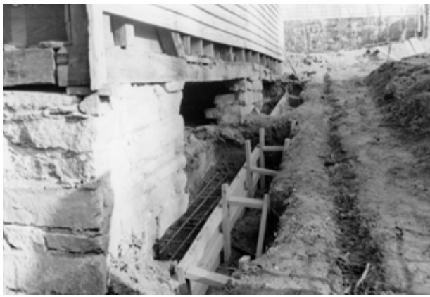
FIGURE 39. View of new footings, 1977. (CARL4008/03/15P)
