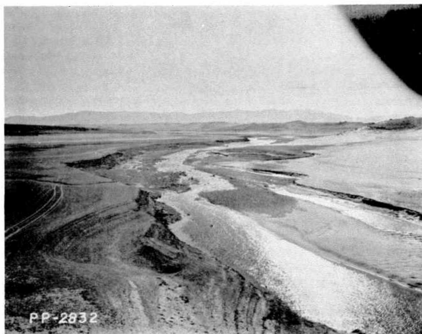
PP-2832--Looking upstream from "narrows" section of North Platte arm of Pathfinder Reservoir toward Range 18. Level deposits shown on left. On right side of picture, sediment deposits have been covered by wind-blown sand. 10-30-58
