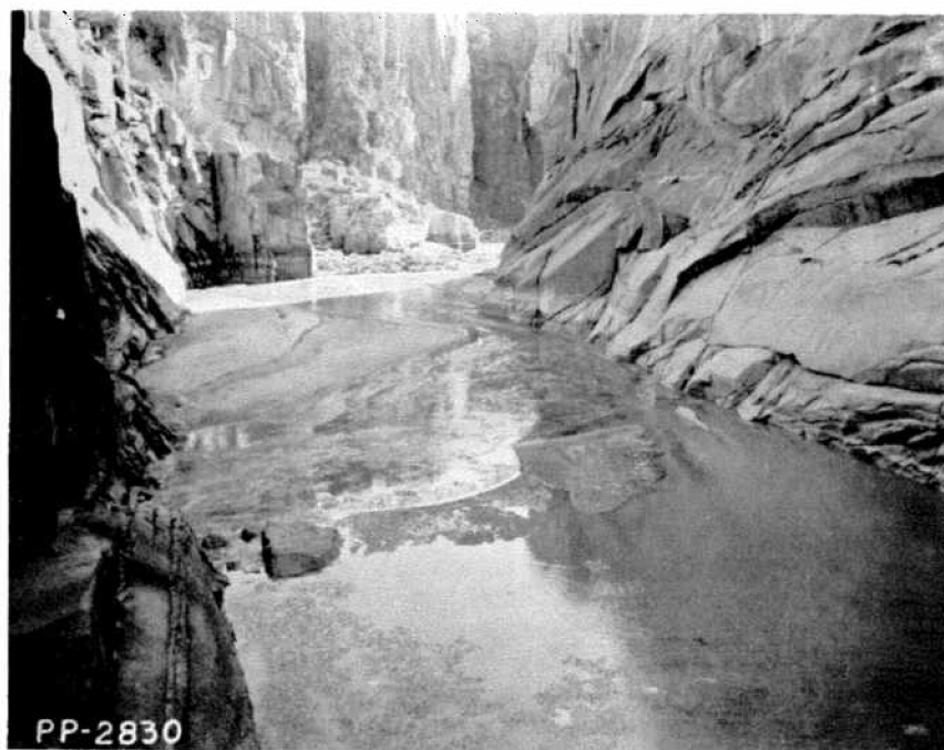
PP-2830--Deposits of material washed from Pathfinder Reservoir and deposited just below Pathfinder Dam. No deposits were present in the river channel before the reservoir was evacuated. 10-31-58
