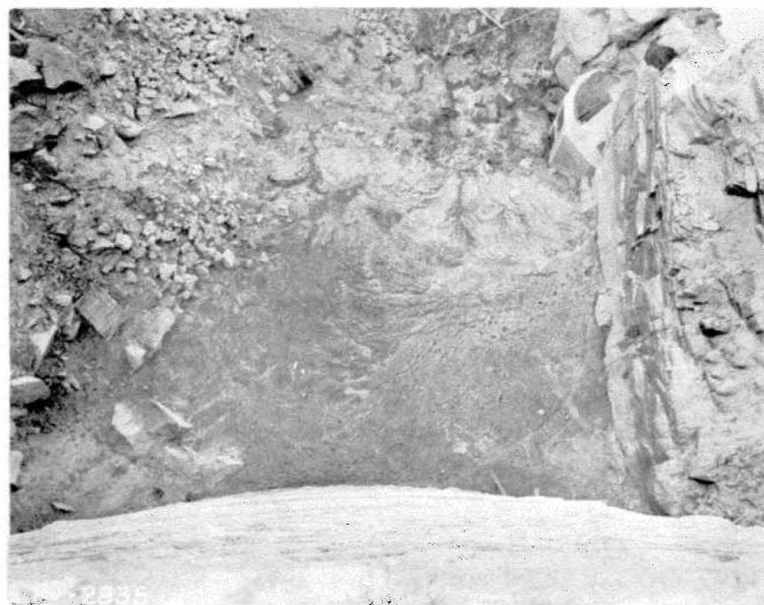
PP-2835--View of upstream face of Pathfinder Dam after reservoir evacuation. River is flowing into lower north outlet tunnel. The triangular shaped lower right deposits of clay, silt, and fine sand have been undisturbed by construction activity and are at elevation 5696.7, approximately up to the top of the north intake vertical trashracks. 10-31-58
