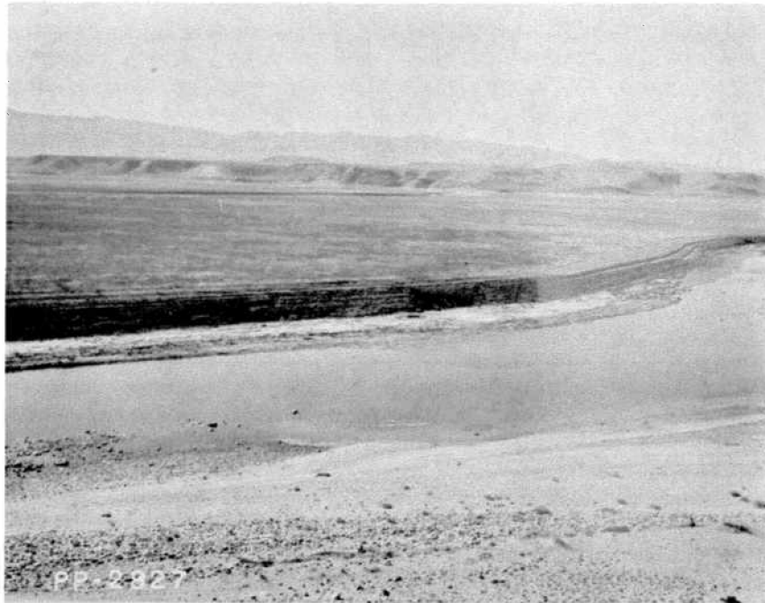
PP-2827--Sediment deposits on North Platte River arm of Pathfinder Reservoir about 1/4 mile upstream from Range 22. Deposits are about 7 feet high and were deposited before construction of Kortes and Seminole Dams upstream. 10-30-58
