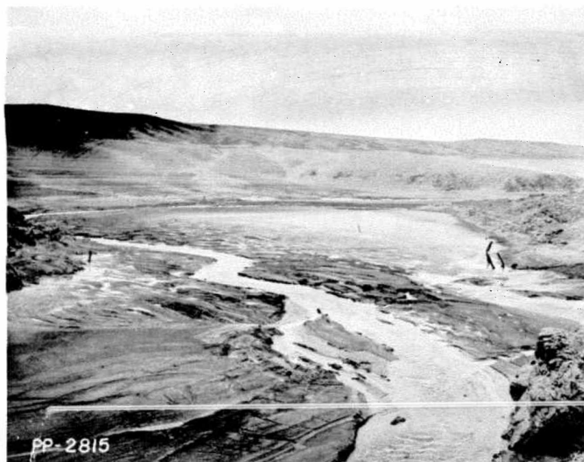
PP-2815--Exposed sediment deposits at Range 2, Pathfinder Reservoir about one-half mile above the dam. Deposits are mostly clay, silt, and fine sand of light to medium density. 10-28-58
