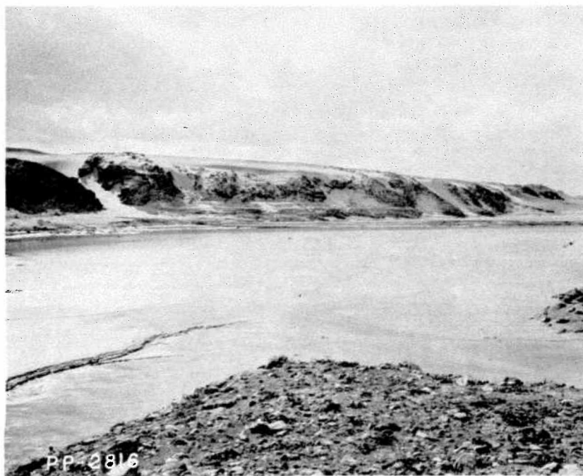
PP-2816--Exposed sediment deposits between Ranges 2 and 3, Pathfinder Reservoir about three-fourths mile above the dam. Deposits are mostly clay, silt, and fine sand of light density that will not support the weight of a rock. Wind-blown sand is also apparent on the upper bench above the river flood plain. 10-28-58
