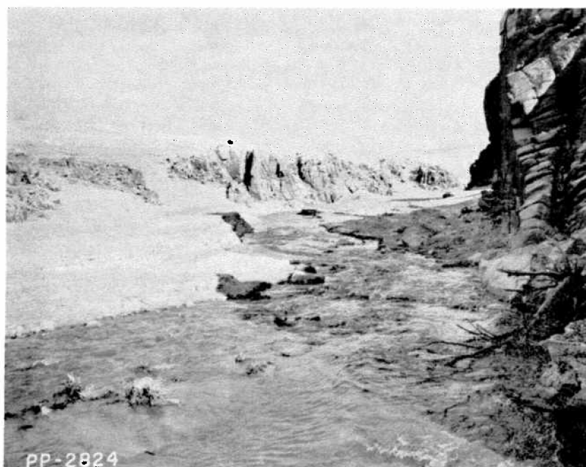
PP-2824--Sweetwater River in "narrows" at Range 34A, Pathfinder Reservoir. River has cut through 3 to 4 feet of coarse sand deposits in this area and is in its original cobble bed. 10-29-58
