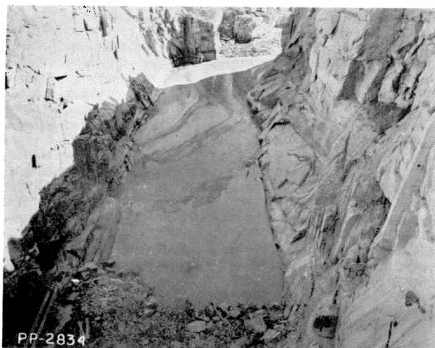
PP-2834--Deposits of material washed from Pathfinder Reservoir and deposited just below Pathfinder Dam. No deposits were present in the river channel before the reservoir was evacuated. 10-31-58
