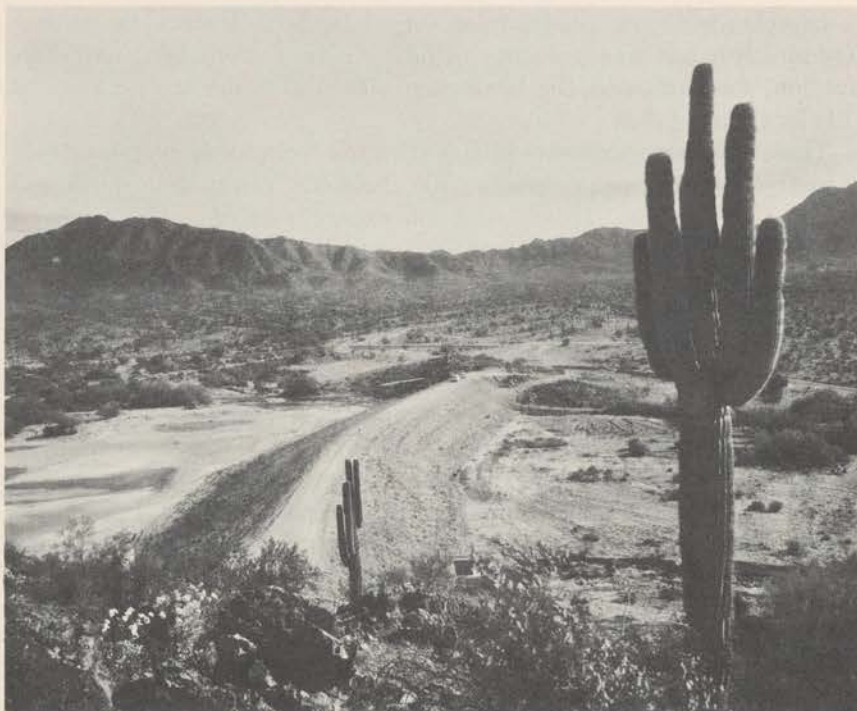
Earth dams will hold the water and prevent the water from running off too fast. Many such dams have been built by BLM on western rangelands.
