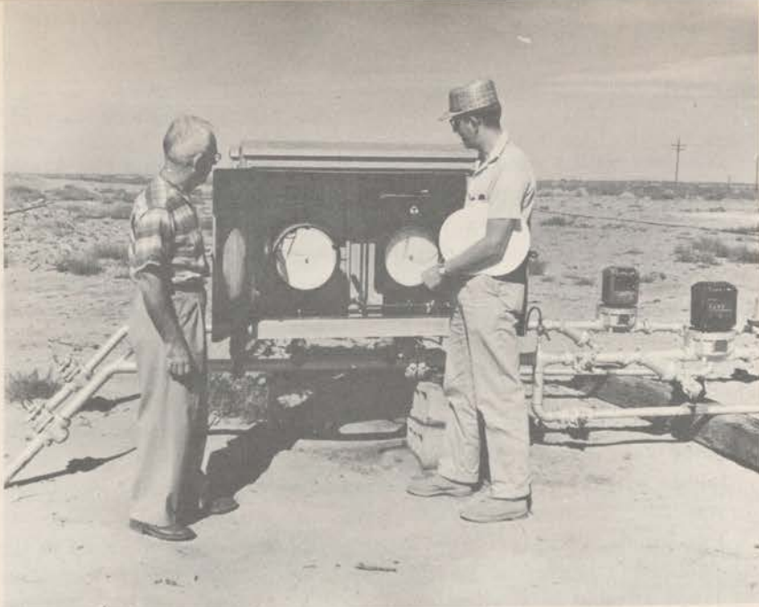
Survey petroleum engineer, accompanied by operator's representative, checking temperature and volume of butane going from lease to storage. On-site inspections assure resource conservation and protection of the Government's royalty interest.
