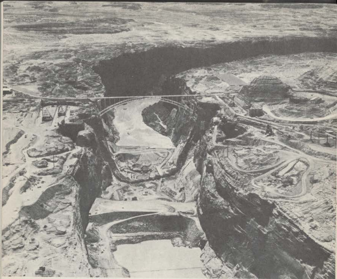
Aerial view looking downstream at Glen Canyon Damsite as excavation work has been almost completed. The upstream cofferdam is 160 feet high.
