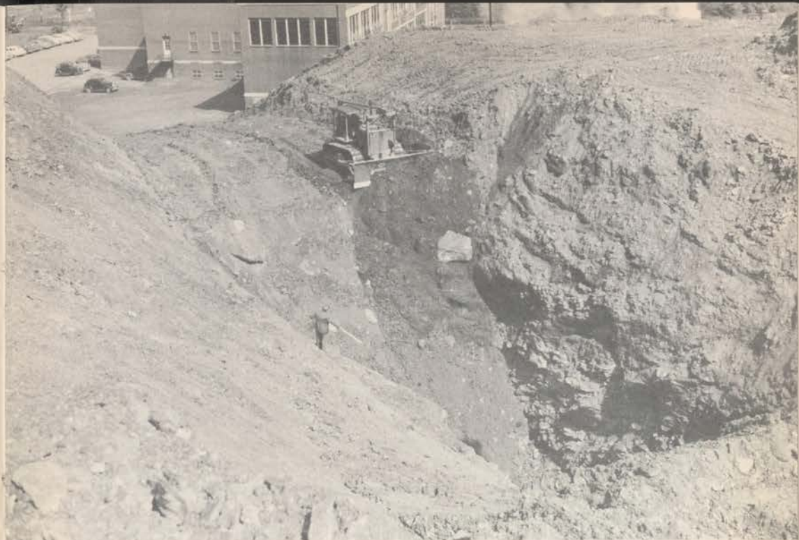
Large-scale excavations by private contractors often are involved in coal fire control projects directed by the Bureau of Mines. This big trench, being backfilled with incombustible material, was necessary in cutting off underground fire threatening school in background.
