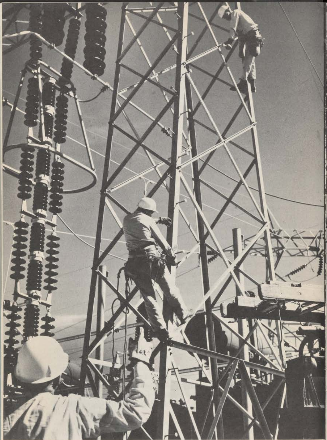
Workmen on the 230-kilovolt bus structure in the substation yard at the Watertown substation, South Dakota.
