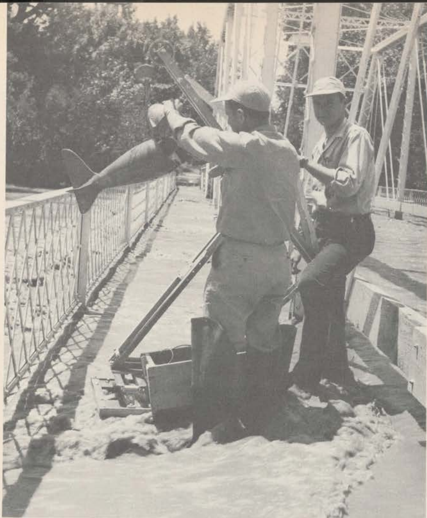
Sampling the sediment load of the Solomon River at Beloit, Kansas during a flood.
