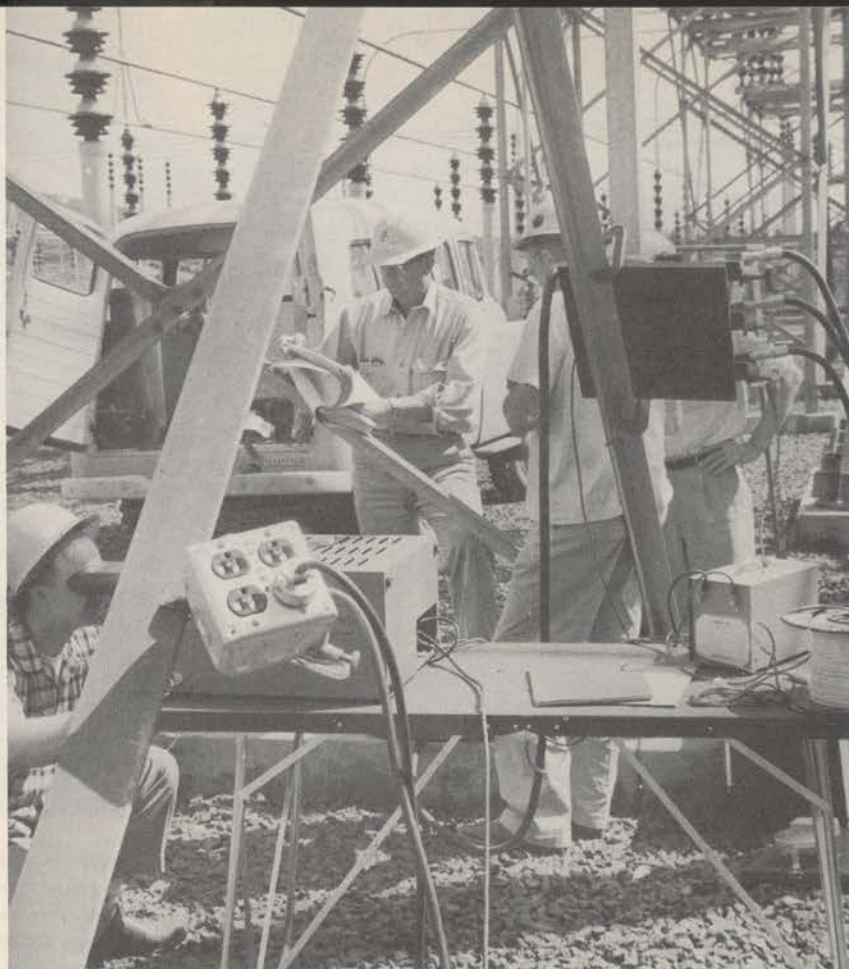
A Bonneville Power Administration testing crew checks out a fault locator and phase selector at one of BPA's large substations.
