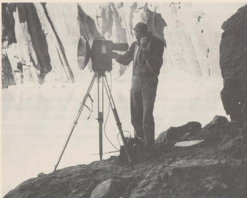
Electronic surveying has replaced the miles of weary walking to measure distances. Deep in Colorado's Glen Canyon this surveyor will move by helicopter to his next station.
