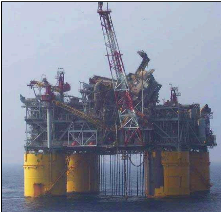
Figure 6.21. Damage to Mars TLP by Hurricane Katrina.
