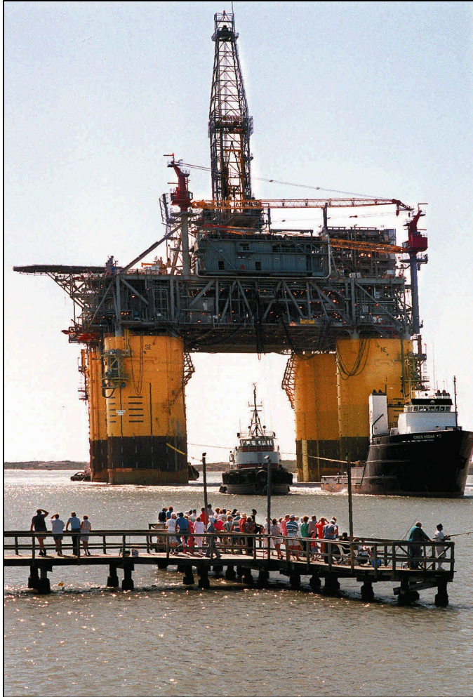
Figure 4.18. Mars TLP tow-out from Ingleside.
