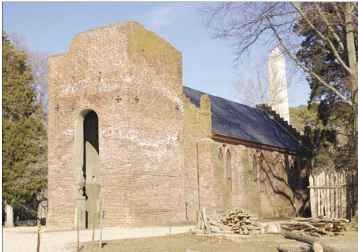
The old church tower at Historic Jamestowne is the only surviving 17th century structure (circa 1680). Photo by Bill Haley, Haley Sharpe Design, LTD.
