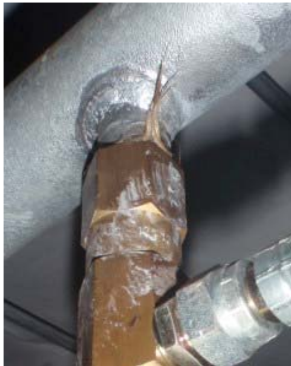
Photograph 23 - Photo showing hemp packing in CO2 system fittings
