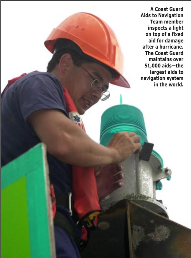
**A Coast Guard Aids to Navigation Team member inspects a light on top of a fixed aid for damage after a hurricane. The Coast Guard maintains over 51,000 aids—the largest aids to navigation system in the world.**
