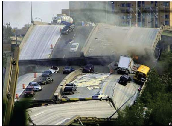
Figure 1. Scene of the Collapse.
