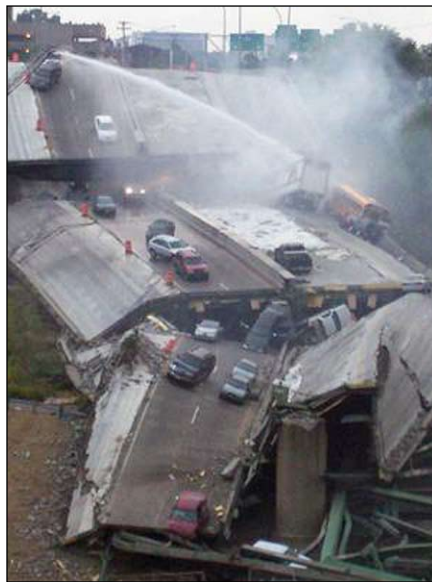
Figure 4. Fire Suppression at the Bridge.
