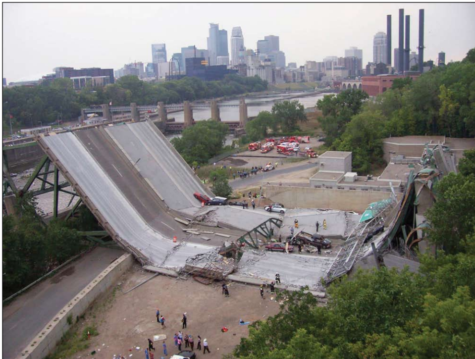
Figure 2. One Section of Collapsed Bridge.
