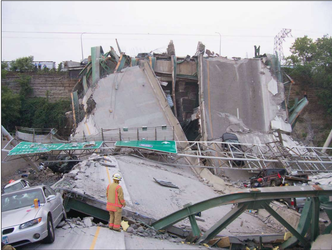
Figure 3. Another View of the Bridge Collapse.
