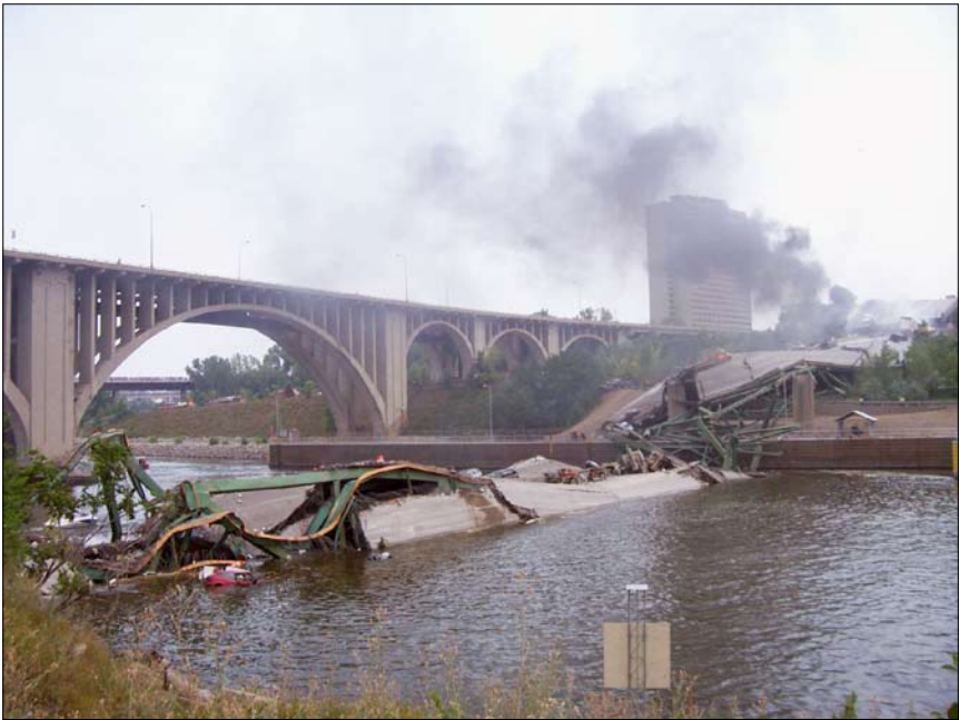
Figure 5. View of the 10th Avenue Bridge.
