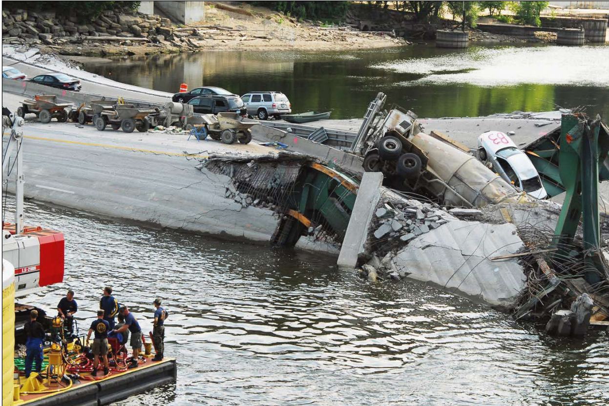
Figure 14. Divers Operating from the Barge.
