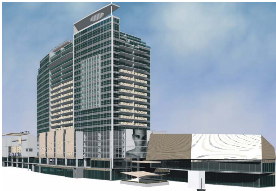
Figure 4-4 Hotel and convention complex. Meeting rooms, ballrooms, and exhibit spaces located above the tsunami inundation elevation can be used to provide areas of refuge.
