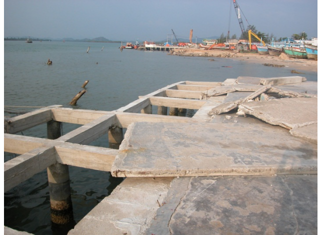
Figure 2-20 Uplift damage to precast concrete floor panels and harbor piers (photo courtesy of M. Saatcioglu, A. Ghobarah and I. Nistor, CAEE, 2005).
