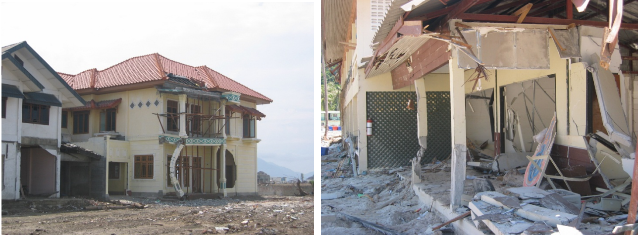
Figure 2-17 Damage to non-engineered concrete columns due to debris impact (photos courtesy of M. Saatcioglu, A. Ghobarah and I. Nistor, CAEE, 2005).
