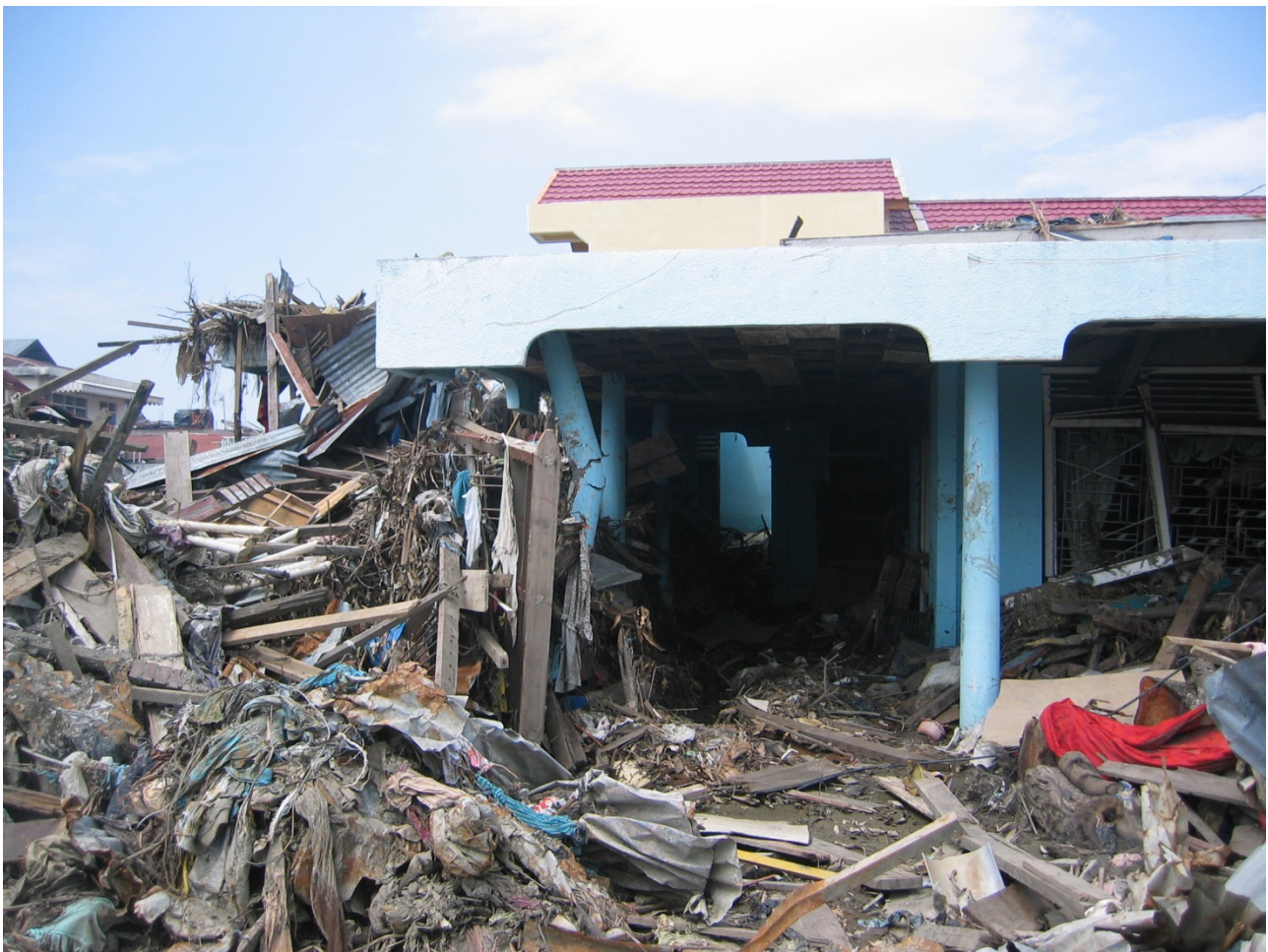
Figure 2-18 Damage to corner column due to debris damming (photo courtesy of M. Saatcioglu, A. Ghobarah and I. Nistor, CAEE, 2005).
