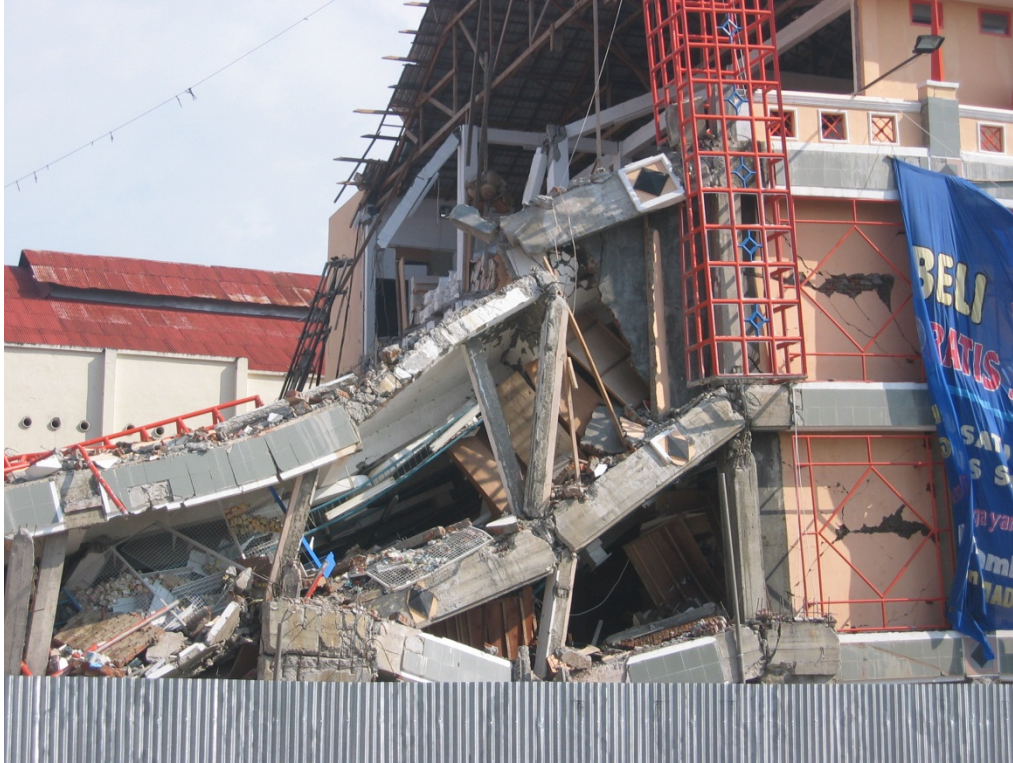
(a) Beam-column connection failures
