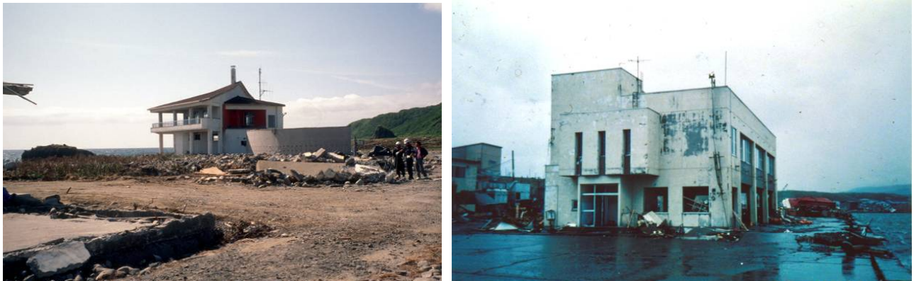
Figure 2-13 Examples of reinforced concrete structures that survived the 1993 Okushiri Tsunami: vista house at Cape Inaho (left); and fish market in Aonae (right) (photo courtesy N. Shuto).
