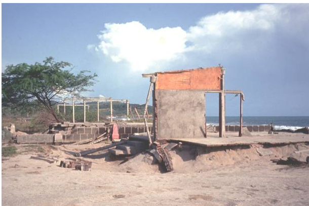
Figure 2-11 Beach houses with varying levels of damage in El Popoyo, Nicaragua (1992 Nicaragua Tsunami). All three houses are in the same vicinity.
