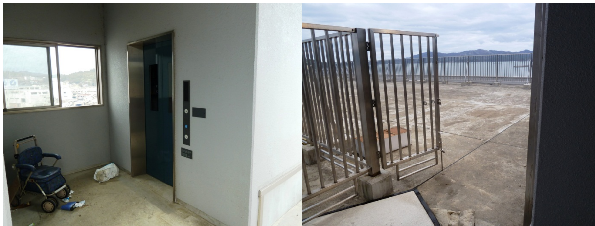
Figure 2-24 Exterior elevator and stairway access to large roof evacuation area protected by 2 meter high braced guard fence on Minamisanriku coastal evacuation building (photo courtesy of I. Robertson, ASCE, 2012).
