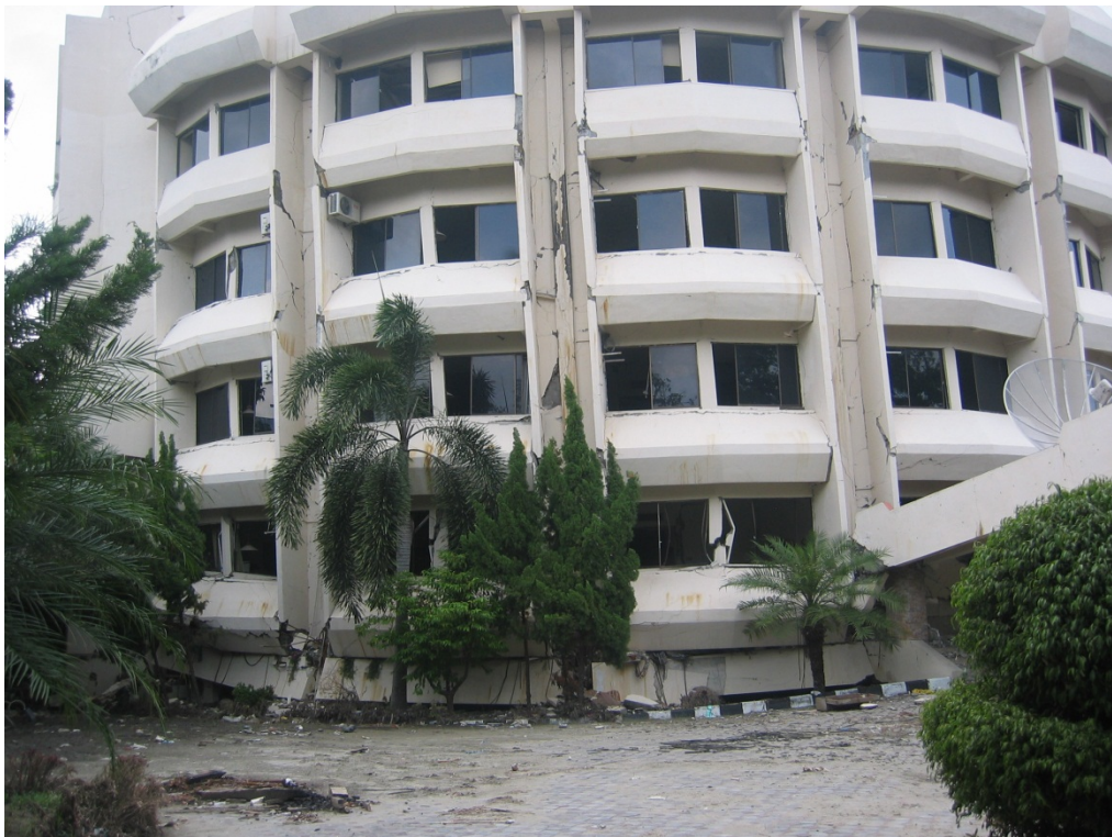
(b) Soft story failure
