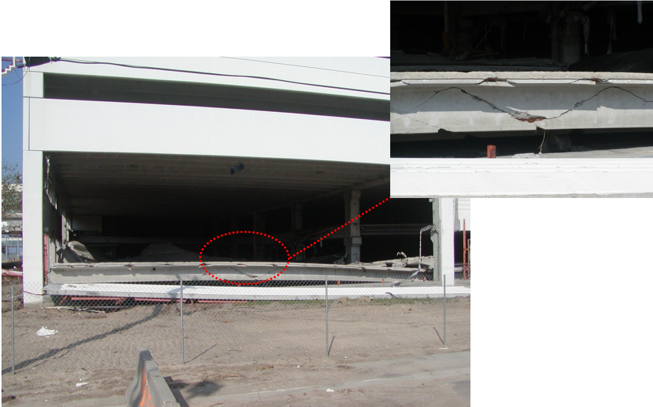
Figure 2-34 Negative bending failure of a prestressed double-tee floor system due to uplift forces (Hurricane Katrina, 2005).
