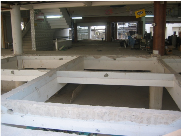
Figure 2-20 Uplift damage to precast concrete floor panels and harbor piers (photo courtesy of M. Saatcioglu, A. Ghobarah and I. Nistor, CAEE, 2005).
