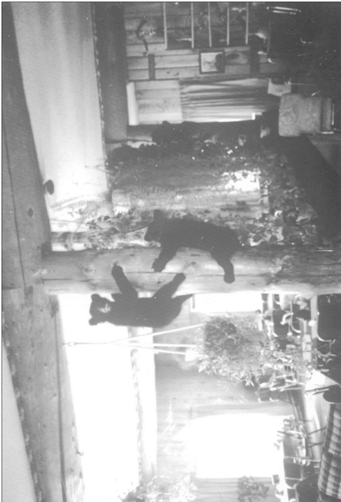
Photo provided by the Minnesota State Fire Marshal Dining room and lounge area on first floor. Note ceiling separations at log beams.
