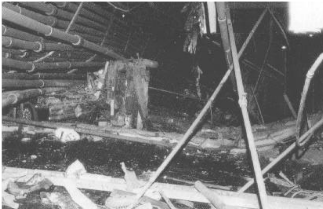
Photo by FDNY Photo Unit
