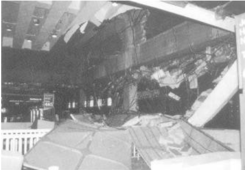
The explosion collapsed a portion of ceiling on the B-5 level onto a PATH train concourse.
