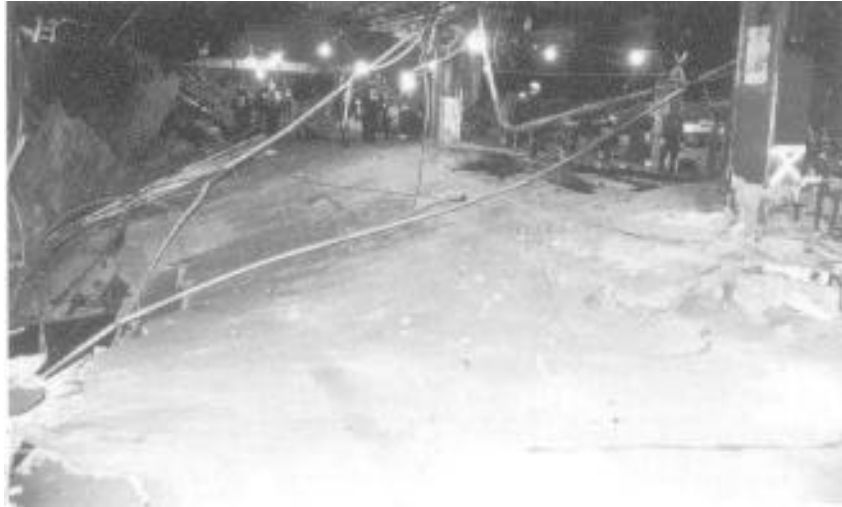
Photo by FDNY Photo Unit
