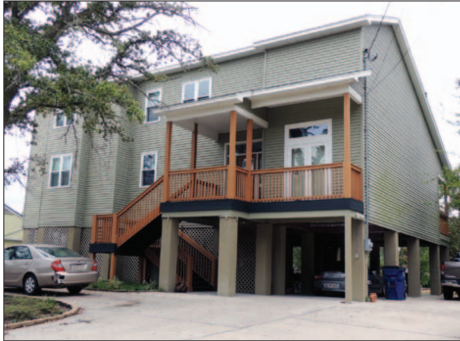
Figure 3-18: Post-Katrina residential reconstruction with service drop attached to the side of house (Slidell, LA).
