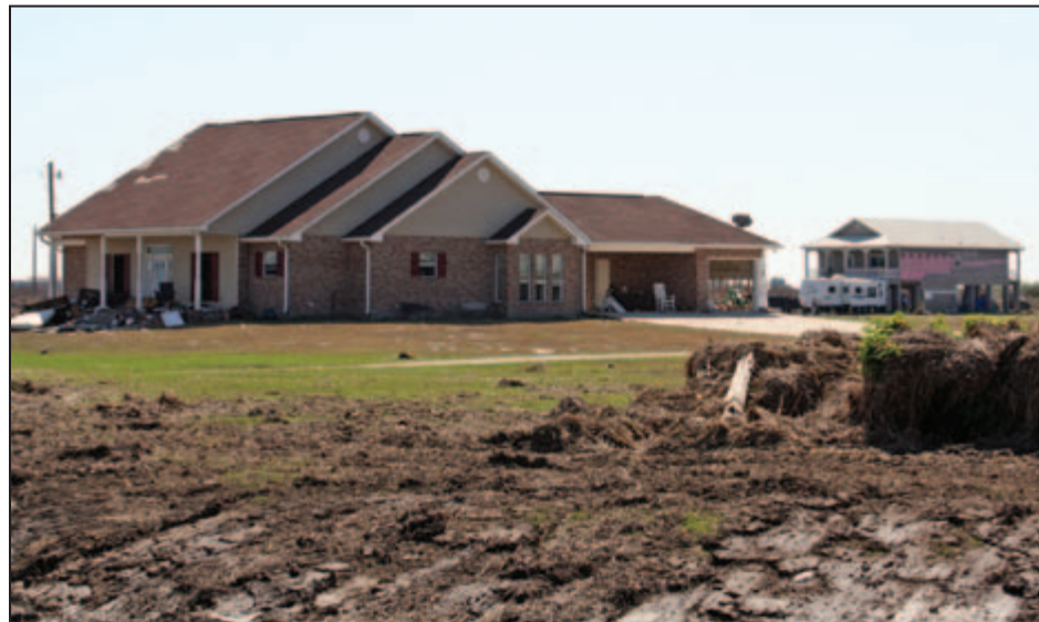
Figure 5-1: Comparison of elevated versus at-grade constructions (Plaquemines Parish, LA).
