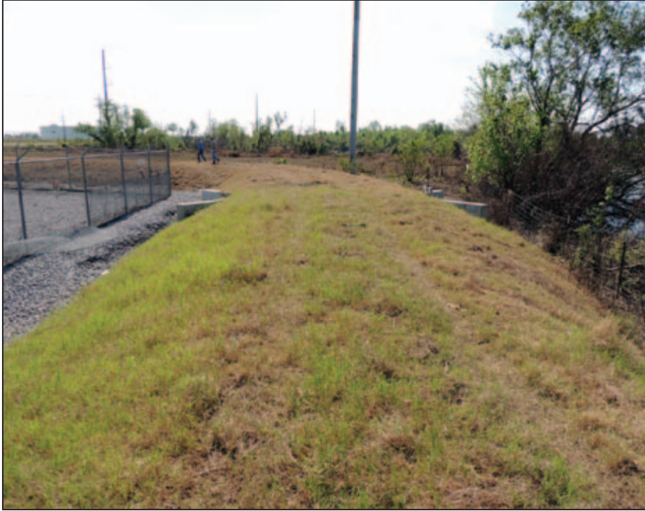
Figure 4-15: A berm was constructed around the perimeter of this substation to protect it after Hurricane Katrina (Belle Chase [West Bank] – Plaquemines Parish, LA).
