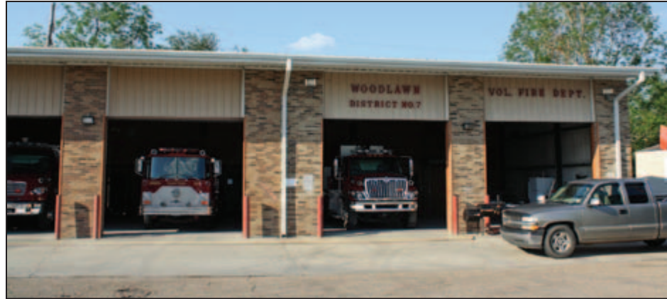
Figure 4-8: Woodlawn Fire Station (Woodlawn [East Bank] – Plaquemines Parish, LA).
