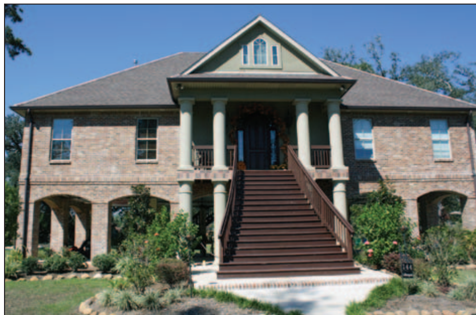
Figure 3-10: House elevated as part of the HMGP Pilot Mitigation Reconstruction Program (Mandeville, LA).
