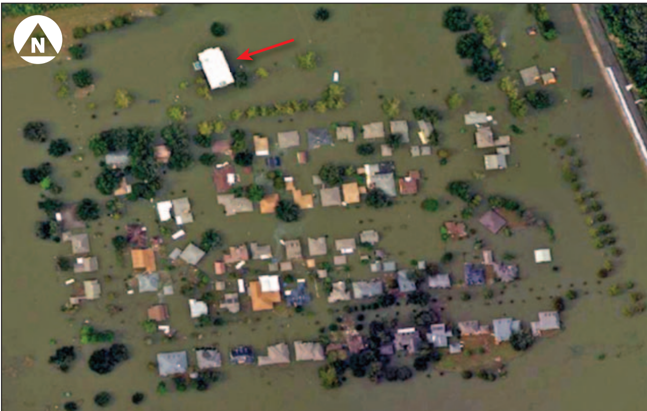
Figure 4-5: Residences in the Braithwaite Park subdivision were inundated with more than 8 feet of water; the auditorium (red arrow) is at the north end of the subdivision (Braithwaite Park [East Bank] – Plaquemines Parish, LA).
