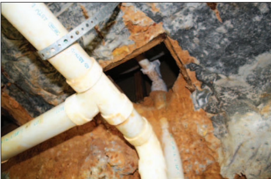
Figure 3-26: Elevated house with open space to interior of the home that would allow fire to spread (Mandeville, LA).
