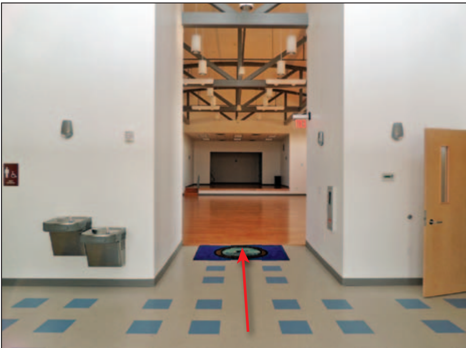
Figure 4-4: No damage was observed in the auditorium (Braithwaite Park [East Bank] – Plaquemines Parish, LA).
