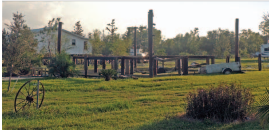
Figure 5-21: Remains of residential building that was approximately 2 to 3 feet above grade (Structure D in Figure 5-18) (St. John the Baptist Parish, LA).
