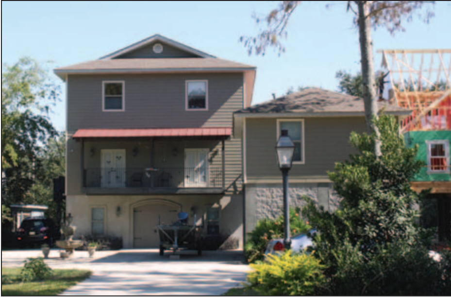
Figure 3-8: Pilot Mitigation Reconstruction Program project; no observed wind damage (Mandeville, LA).
