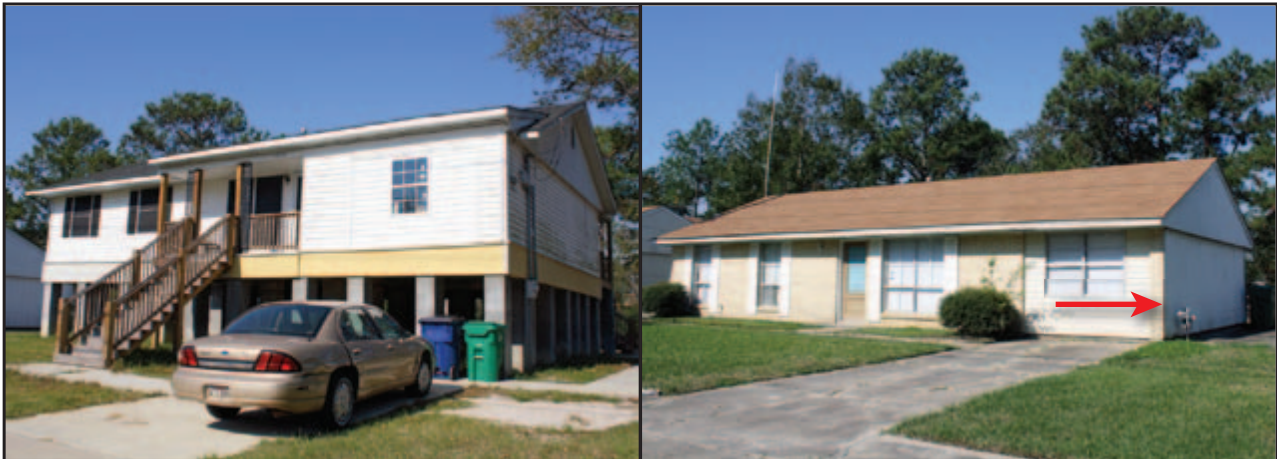
Figure 3-9: Neighboring residential buildings; the elevated residence had no observed damage, while the non-elevated home had significant interior damage caused by more than 2 feet of flooding (red arrow indicates flood depth) (Slidell, LA).
