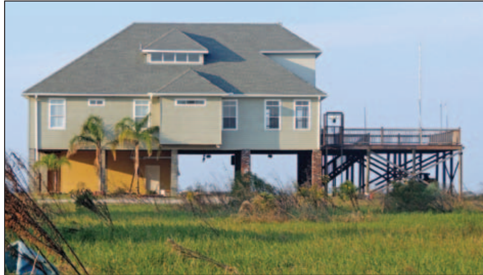
Figure 5-25: Residence built about 2000 with minimal damage to partially enclosed areas below the lowest floor (Structure F in Figure 5-18) (St. John the Baptist Parish, LA).
