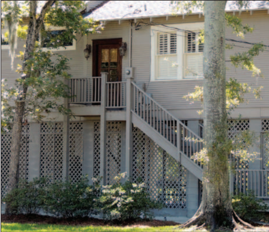
Figure 3-16: Residential building with electric meter installed adjacent to side entrance (Mandeville, LA).
