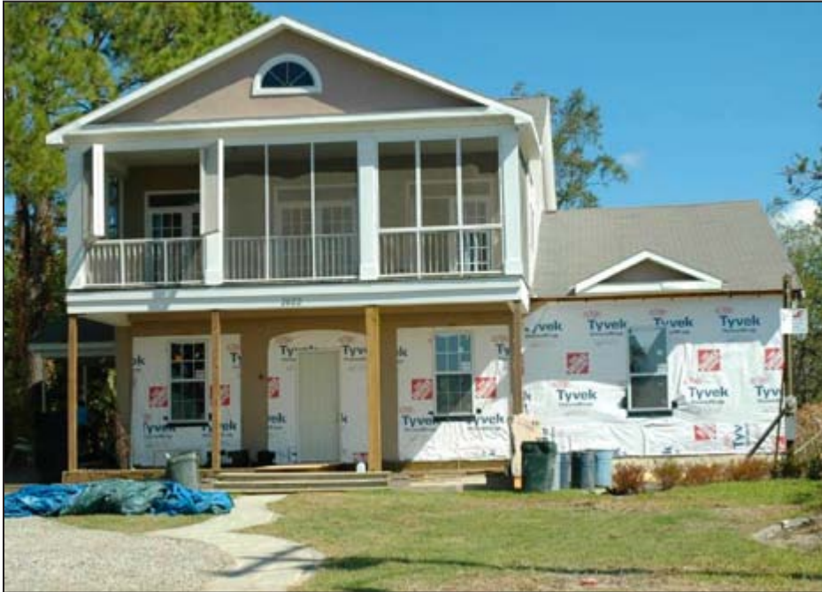
Figure 5-9: Single-family residence post-Katrina (Mandeville, LA).
