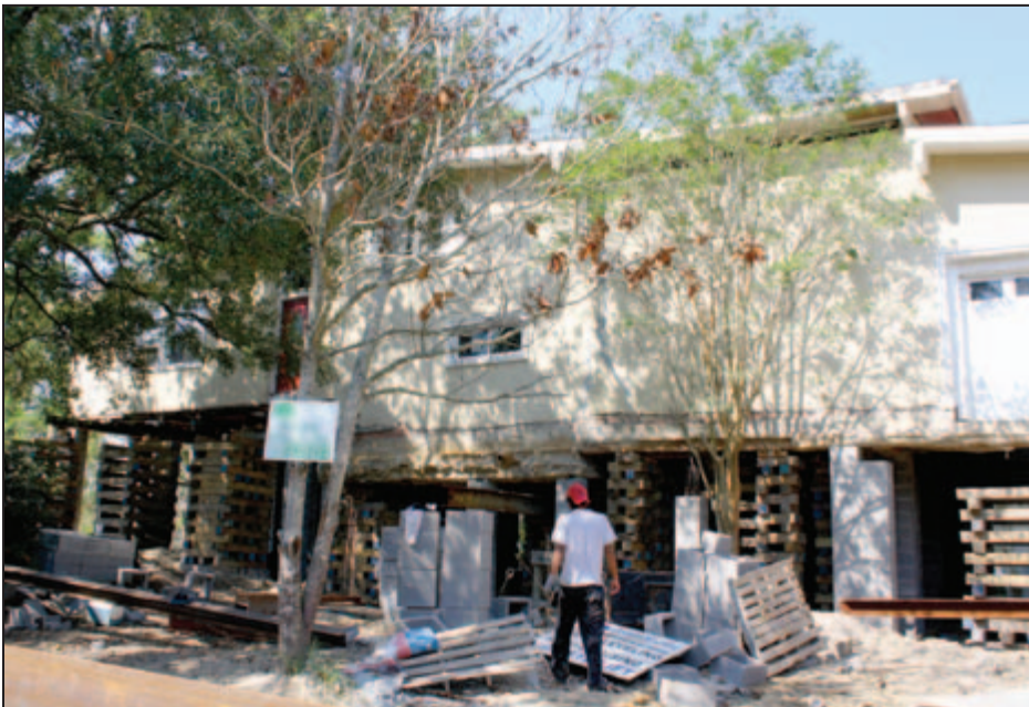
Figure 3-12: Slab-on-grade elevation in progress (Slidell, LA).
