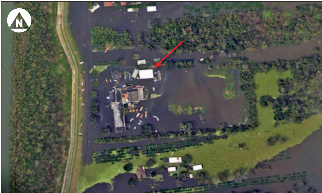
Figure 4-9: Post-Hurricane Isaac aerial of Woodlawn Fire Station (Woodlawn [East Bank] – Plaquemines Parish, LA). AERIAL COURTESY OF NOAA; GENERATED FROM HURRICANE ISAAC RESPONSE IMAGERY VIEWER AT HTTP://STORMS.NGS.NOAA.GOV/STORMS/ISAAC/ .
