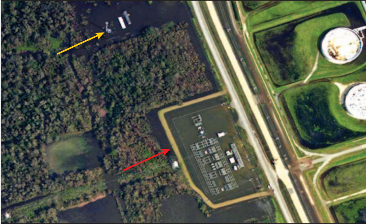
Figure 4-17: The protective berm (red arrow) was overtopped, resulting in damage to the substation; note cellular tower (yellow arrow) northwest of the substation (Belle Chase [West Bank] – Plaquemines Parish, LA).
