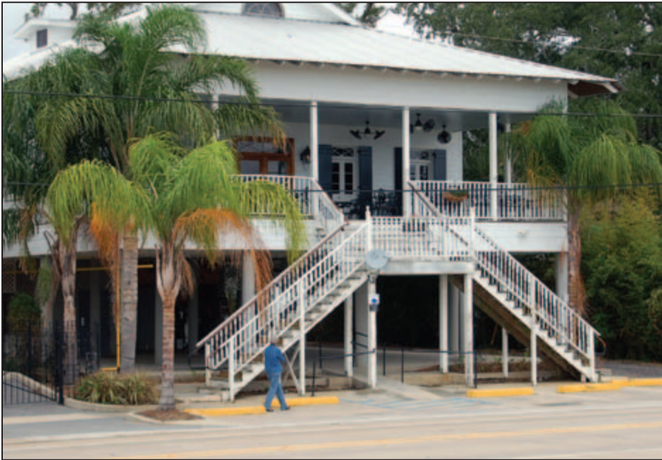
Figure 5-14: The same nonresidential building along Lakeshore Drive in Mandeville elevated post-Hurricane Katrina (Mandeville, LA).
