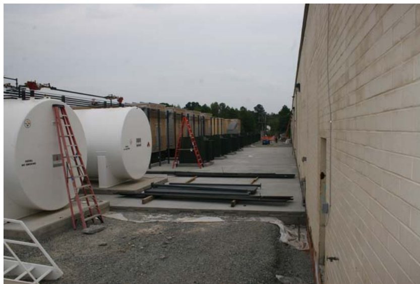
Figure 2: Diesel fuel tanks and backup generators adjacent to DC2.
