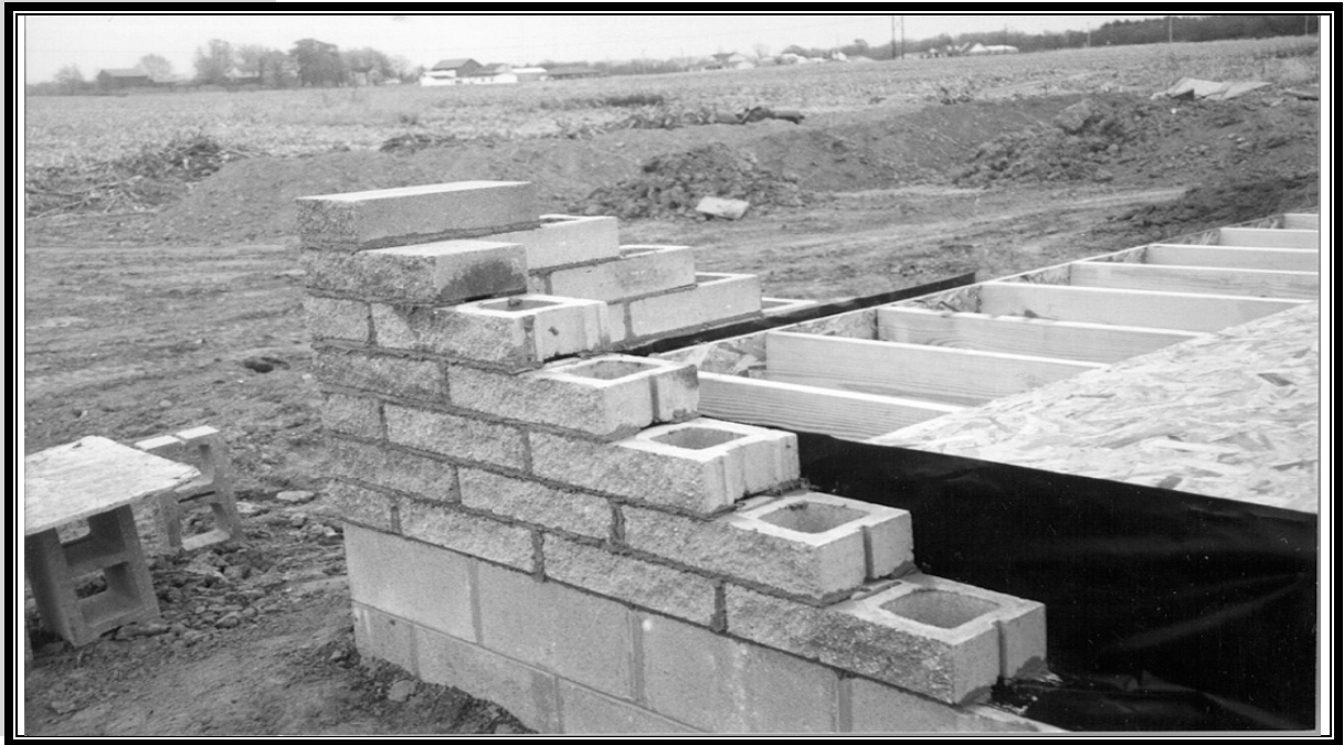
FIGURE 1.6 House Construction Using Concrete Masonry
