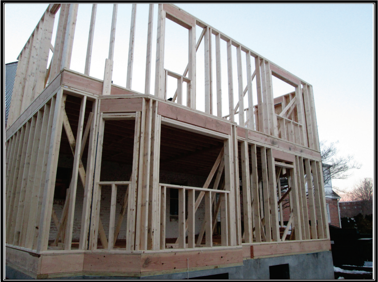
Modern Platform-Framed House Under Construction
