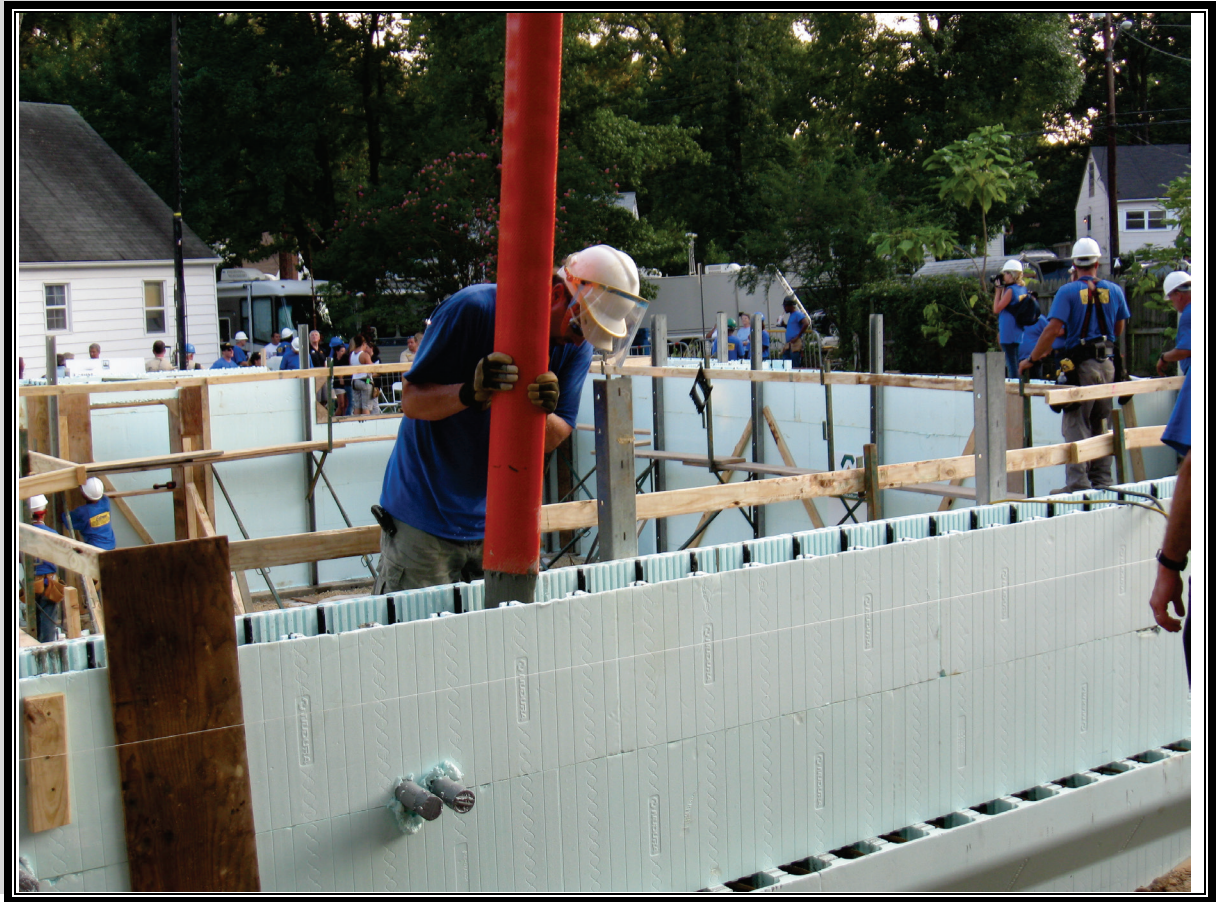
House Construction Using Insulating Concrete Forms
