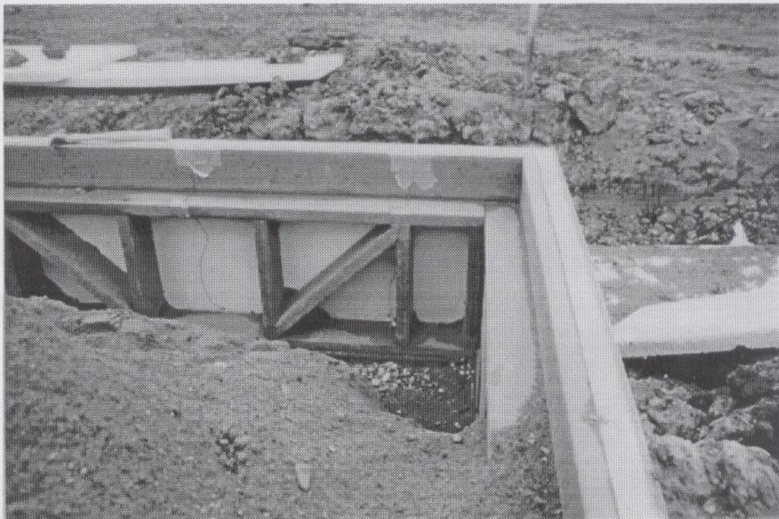
Figure 9. Photograph of the recycled plastic lumber used in the FPSF design at the second Fargo, North Dakota site (home #2)
