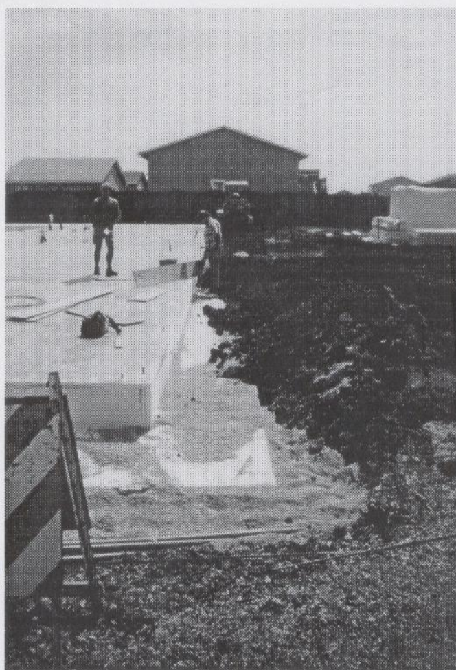
Figure 7. Photograph of the FPSF foundation construction at Fargo, North Dakota (home #1).
