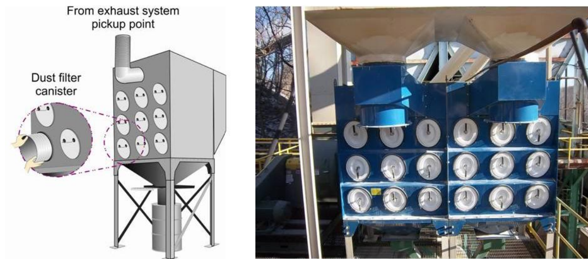
Figure 1.20. Cartridge collector with dust filter canisters.
