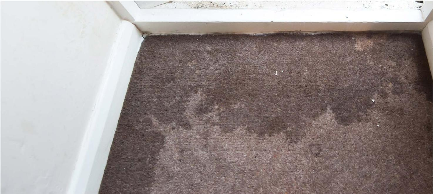
This entryway carpet is visibly saturated along the edges. Therefore, combine the size of the wet edges for scoring.
